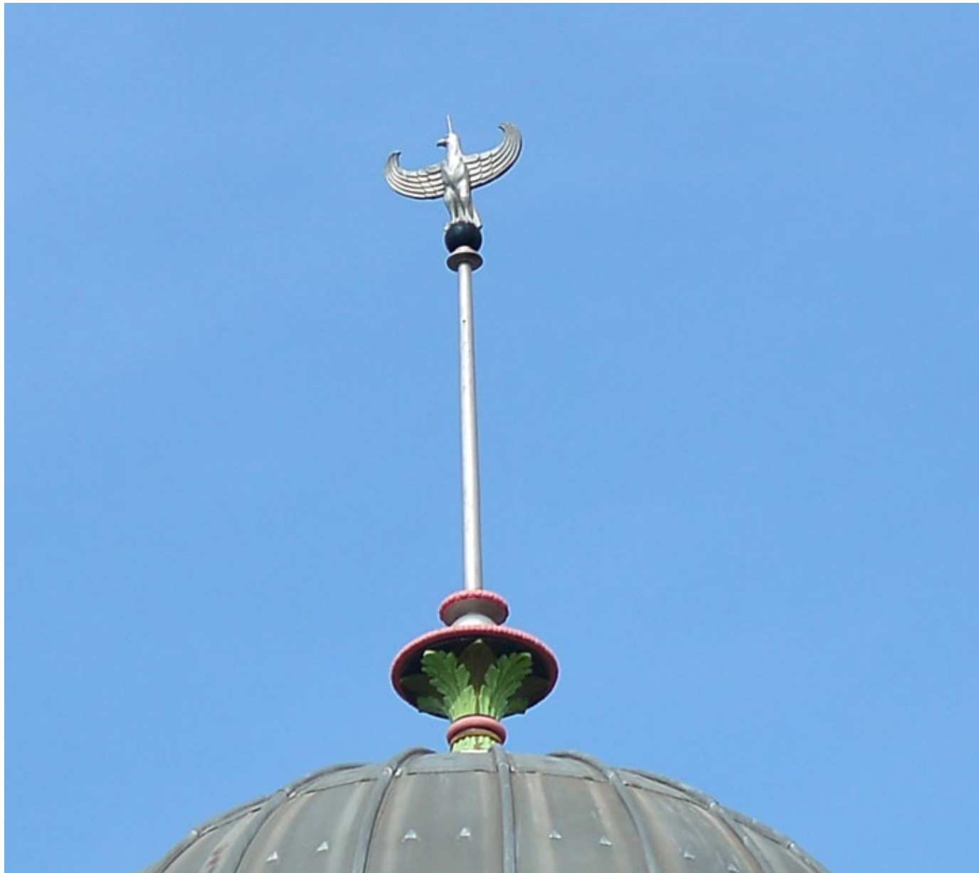
The domed roof of each tower.
