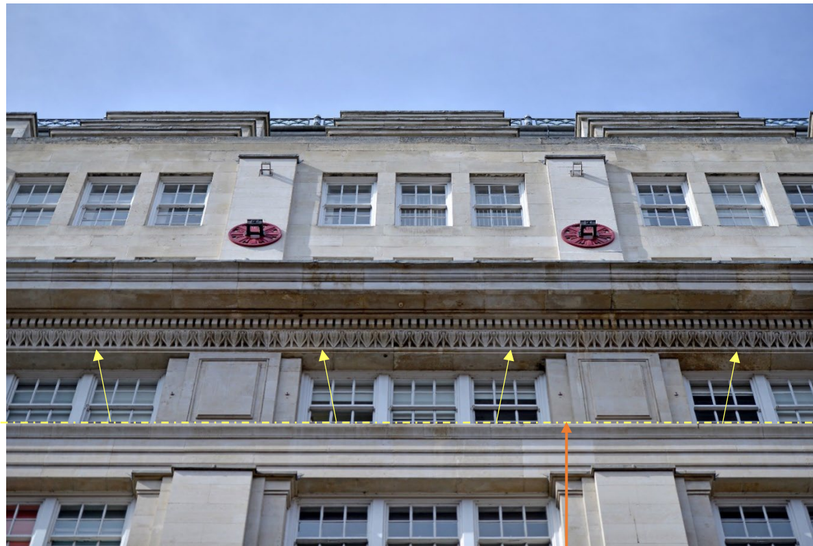
Concealed linear LED to uplight grand parapet on all three facades
