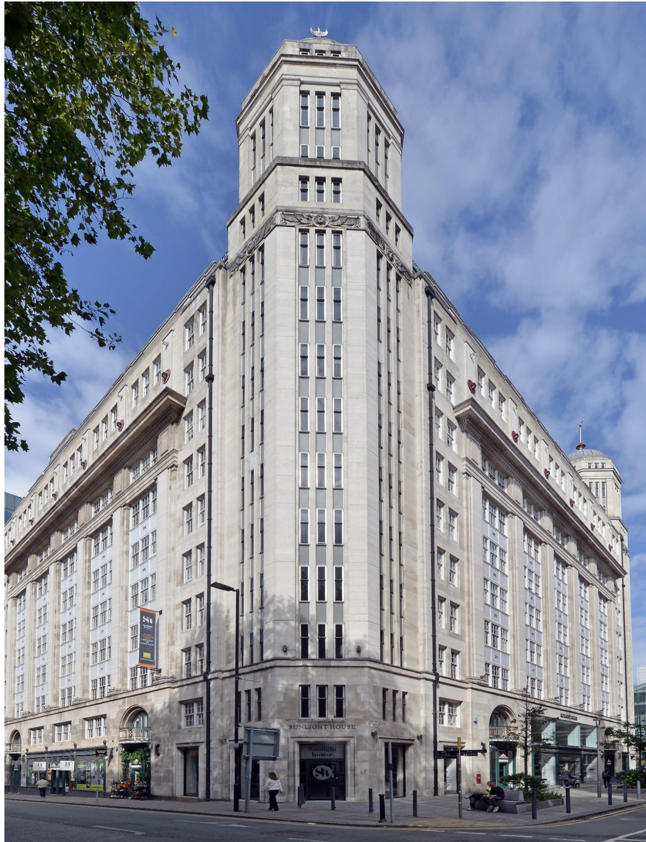
Sunlight House. Intersection of Quay Street and Little Quay Street
