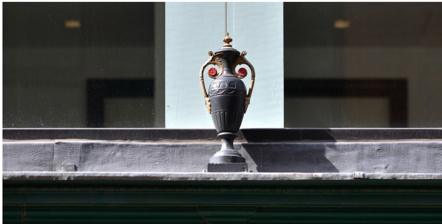
Existing Entrance Canopy to Little Quay Street with original decorative vases above.
