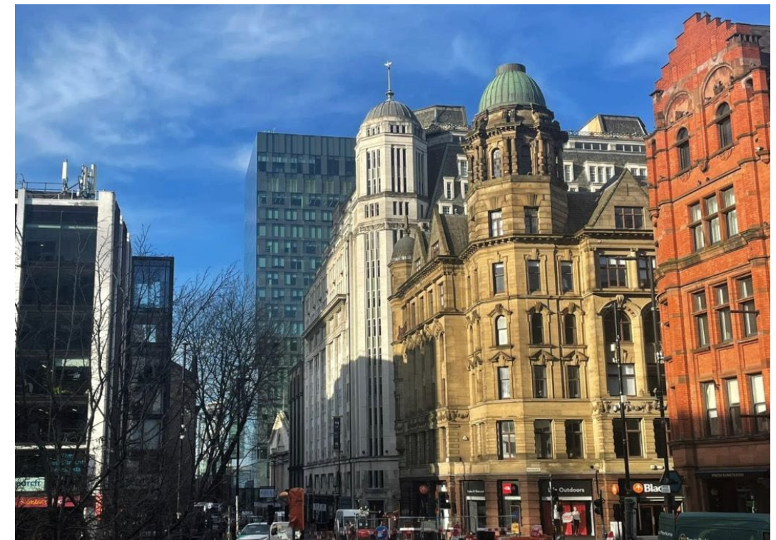
Sunlight House view looking West on Quay Street
