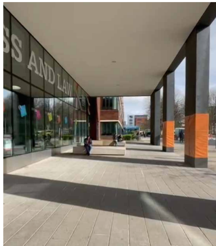
Existing view of external covered walkway
