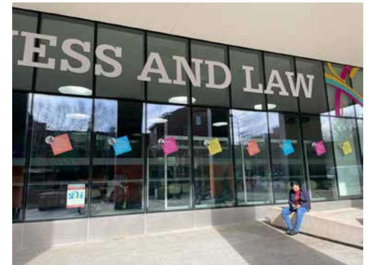
Existing view of external elevation & existing manifestation
