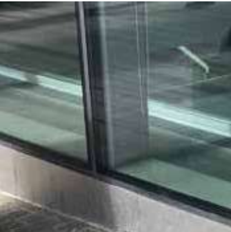
2 Structural silicone glazed curtain walling system
