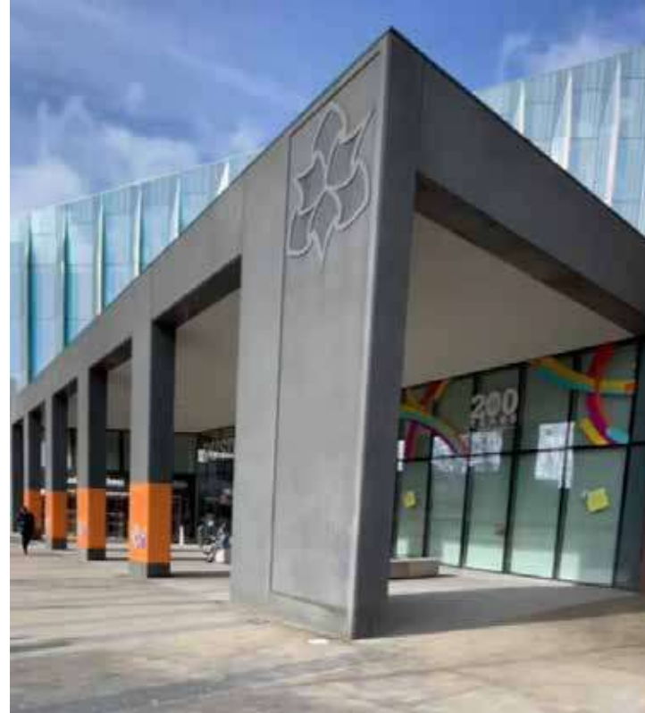
Existing view of canopy and entrance space
