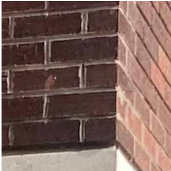
3 Red brick facade to adjacent library building
