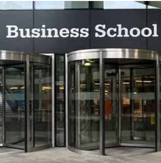
4 Brushed stainless steel finish to entrance doors
