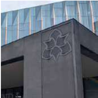
1 Pre cast concrete panels to canopy roof and columns
