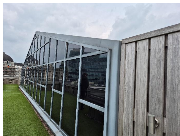
Photo 8: PVC and glass rooftop area (south-western elevation)
