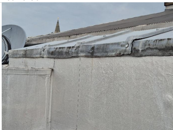
Photo 15: Sealed flashing at rooftop structure
