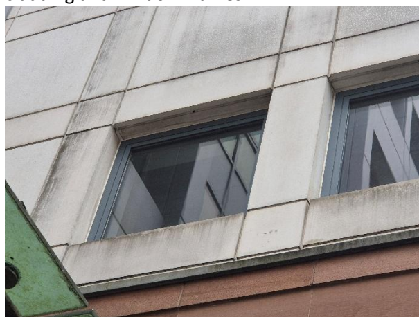
Photo 5: No gaps or opportunities for bat access at recessed areas
