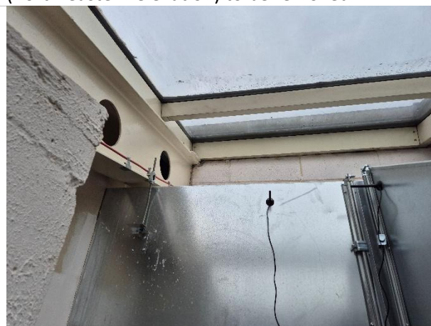
Photo 12: Interior of PVC rooftop area
