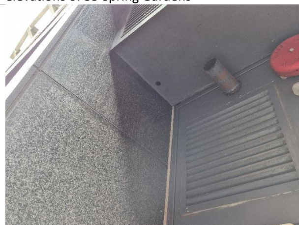
Photo 4: No gaps or opportunities for bat access at recessed areas
