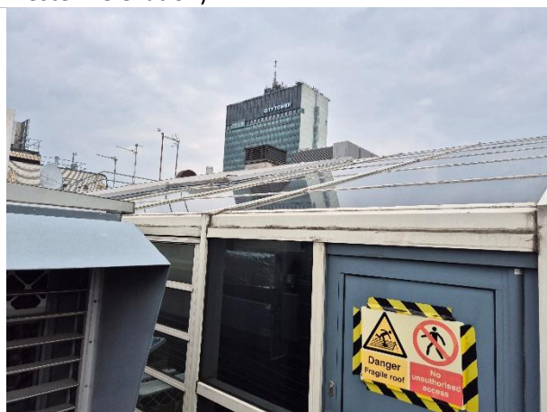
Photo 9: Roof of PVC framed areas at rooftop
