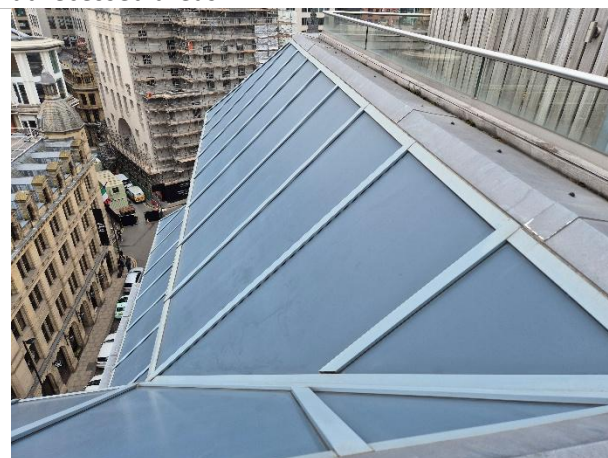
Photo 6: Sealed windows and frames at upper floor levels
