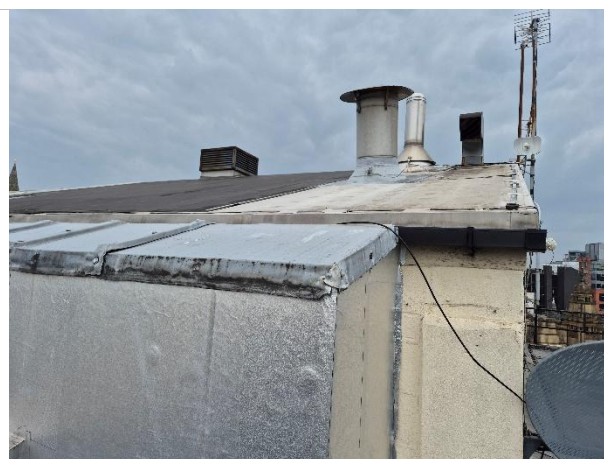
Photo 14: Roof of PVC framed areas at rooftop (this north-eastern section will be removed)
