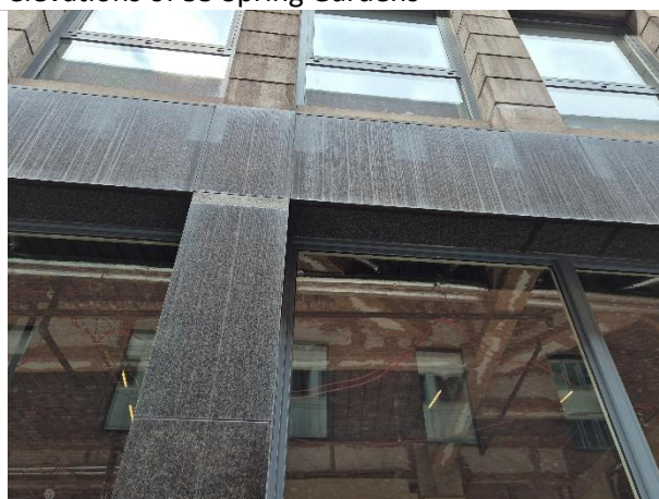
Photo 3: Ground floor elevation showing sealed cladding and window frames
