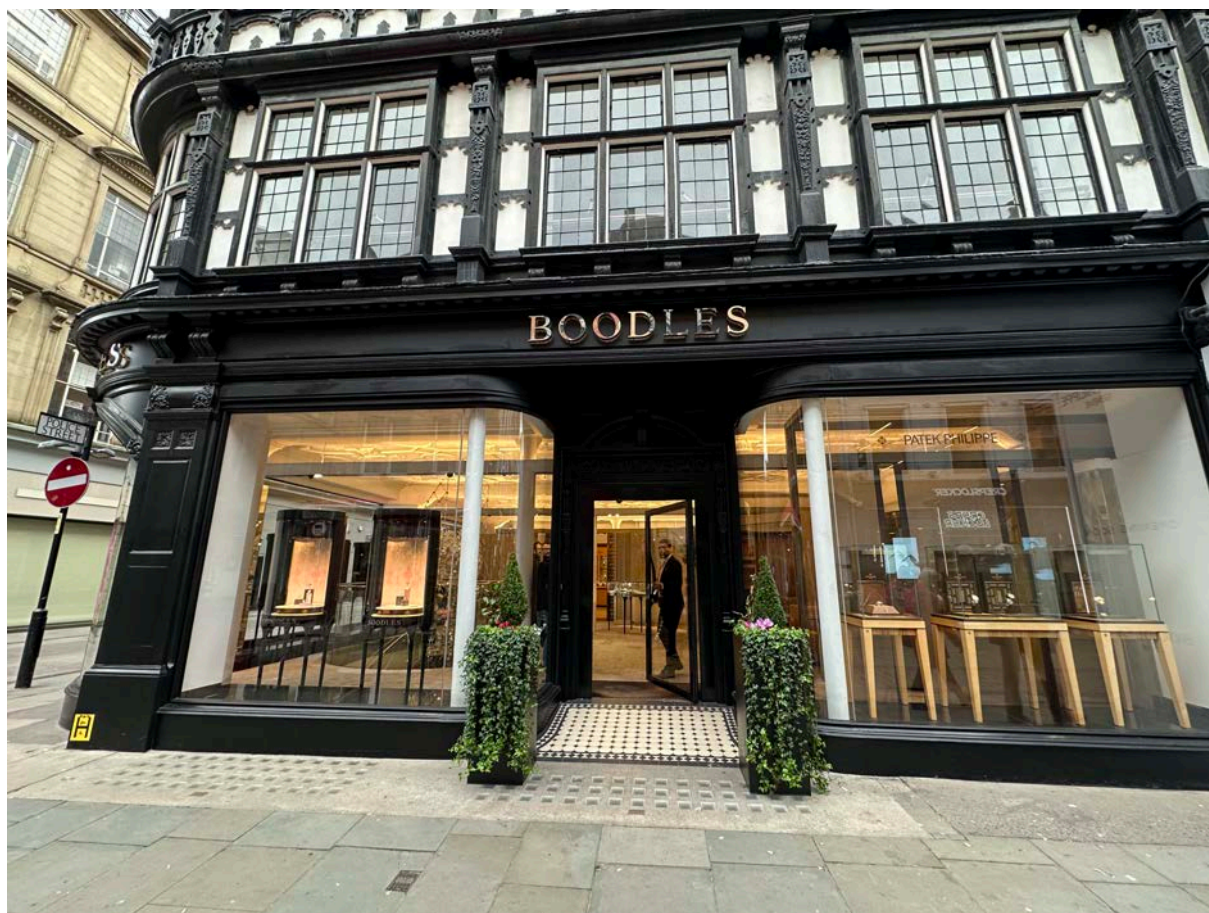
Photograph 4 - Adjacent retail unit shopfront as is currently in 2025.
