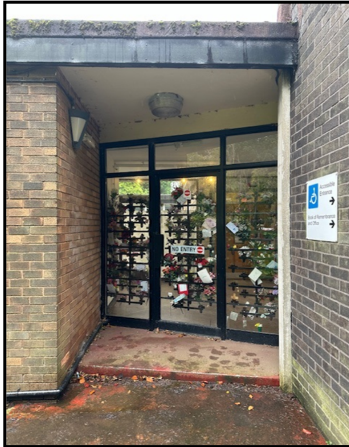
Figure.6: Chapel entrance doors (external) northwestern elevation
