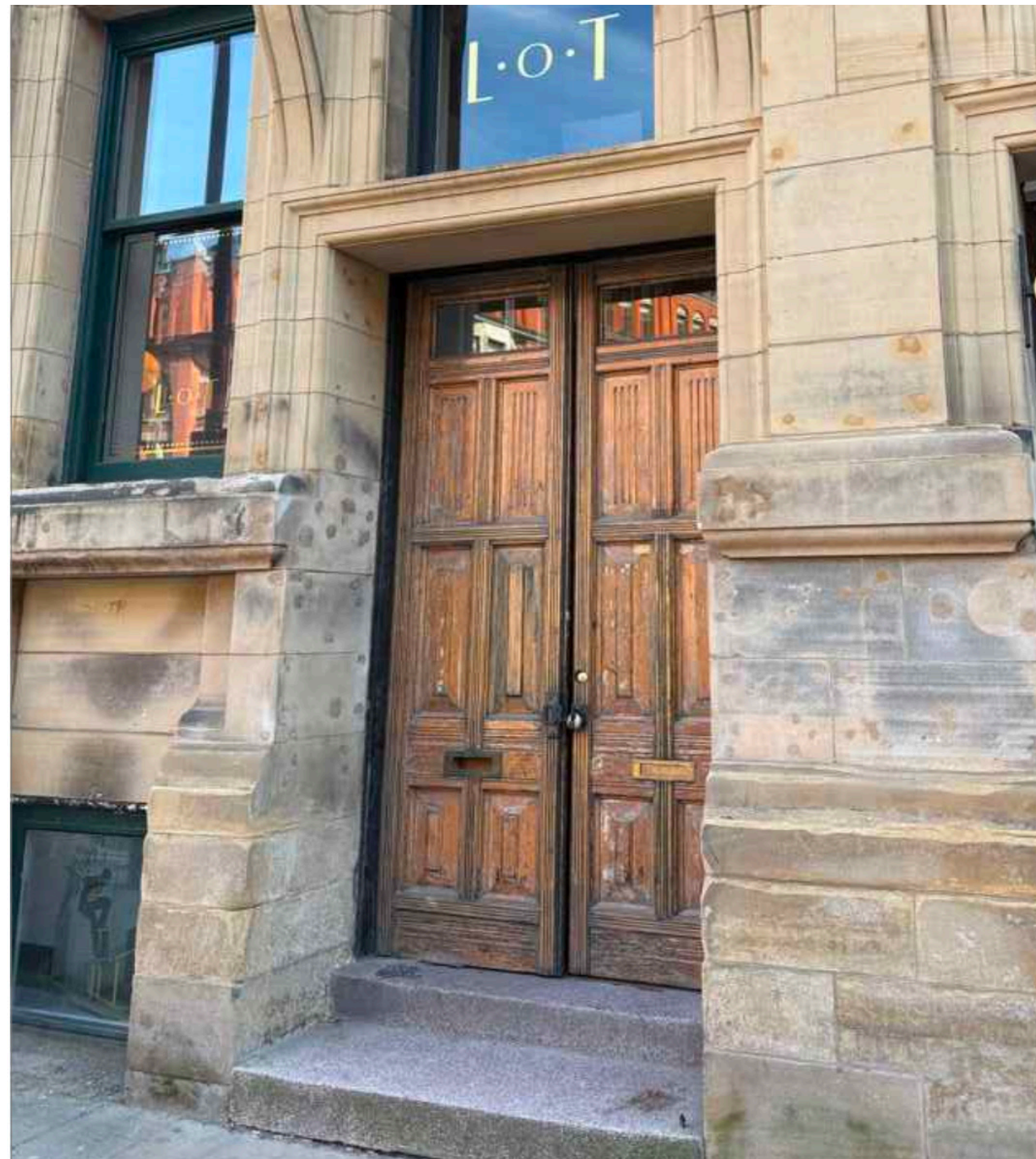
Main entrance on Newton Street
