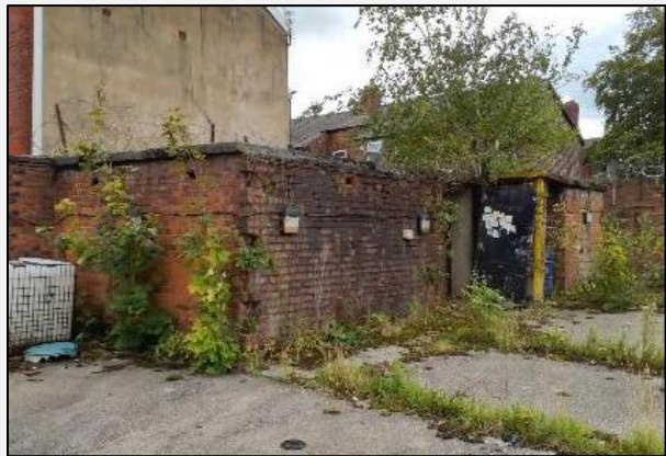
IMAGE 3A – BUILDING 3 EXTERNAL
