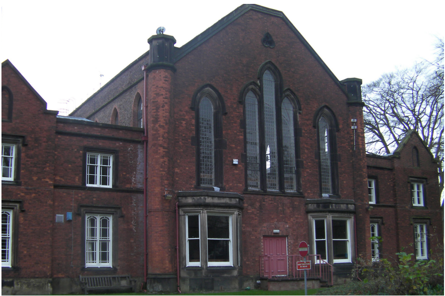
the chapel, previous to conversion into 10 no. apartments
