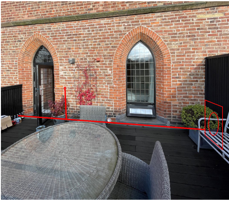
external equipment in exinting roof terrace
