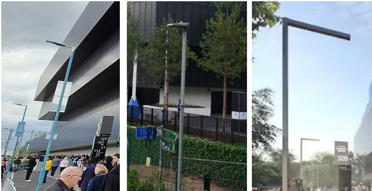
Figures 8, 9 and 10 (from left to right) - 8m tall LED lighting columns along Joe Mercer Way, 4m tall LED lighting columns along the Ashton Canal, and 6m tall rectangular style feature columns on the canal side external concourse of the arena.
