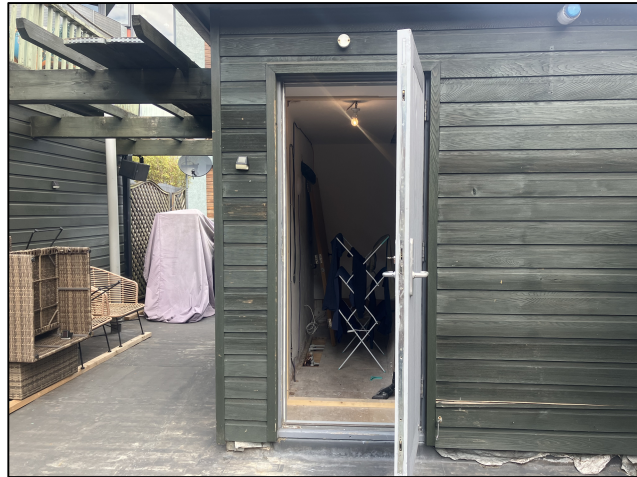
Image of existing roof structure and 'pagoda'
