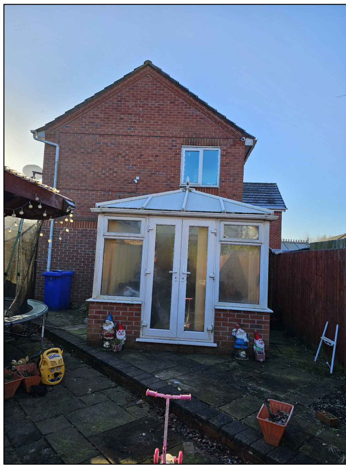
Site Photo-Existing Side Elevation
