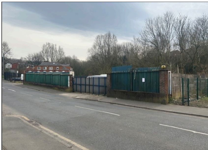
View of application site from opposite side of Old Market St
