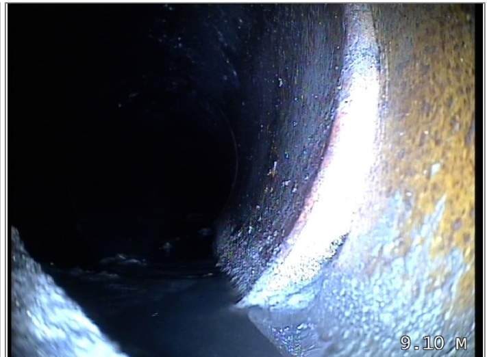
Survey abandoned - Remark: UNABLE TO PUSH FURTHER
