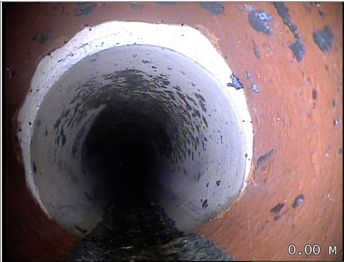
Start node type, manhole, reference MH 03
