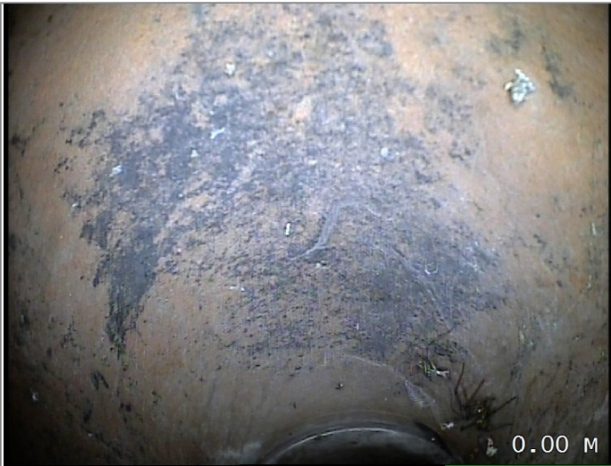
Start node type, gully, reference GULLY 2
