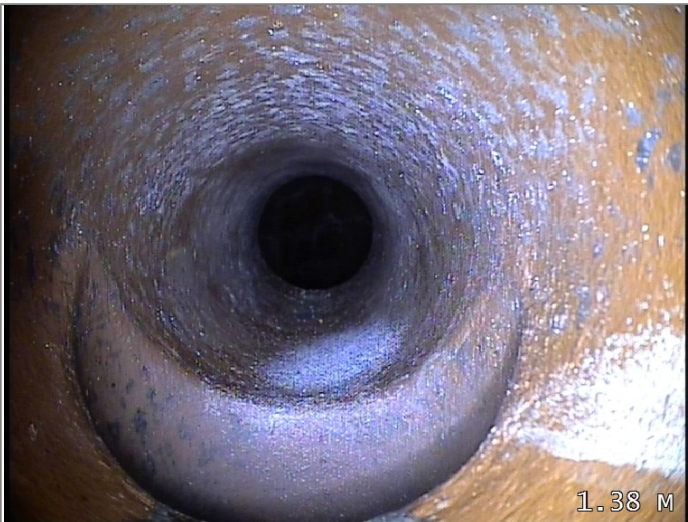
Line of drain/sewer deviates down - Remark: BACKDROP
