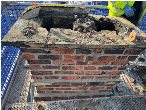
Images showing poor quality of brickwork:
