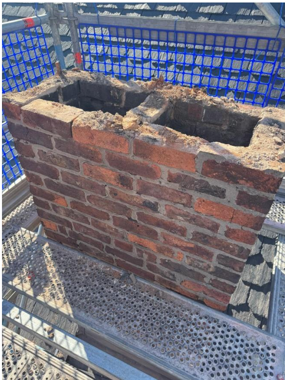
Images showing poor quality of brickwork:
