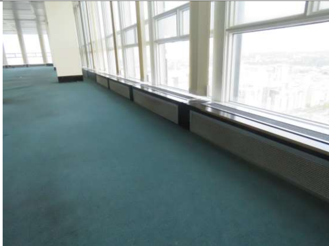
22-12 View of curtain walling and Weathermaster.
