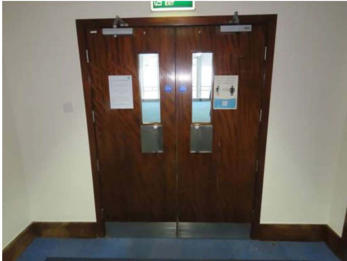
22-02 View of original timber double doors to office space.
