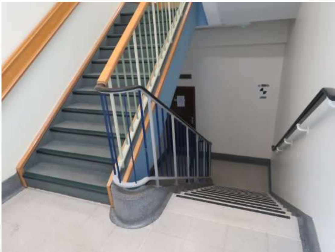
22-07 View within east stairwell.
