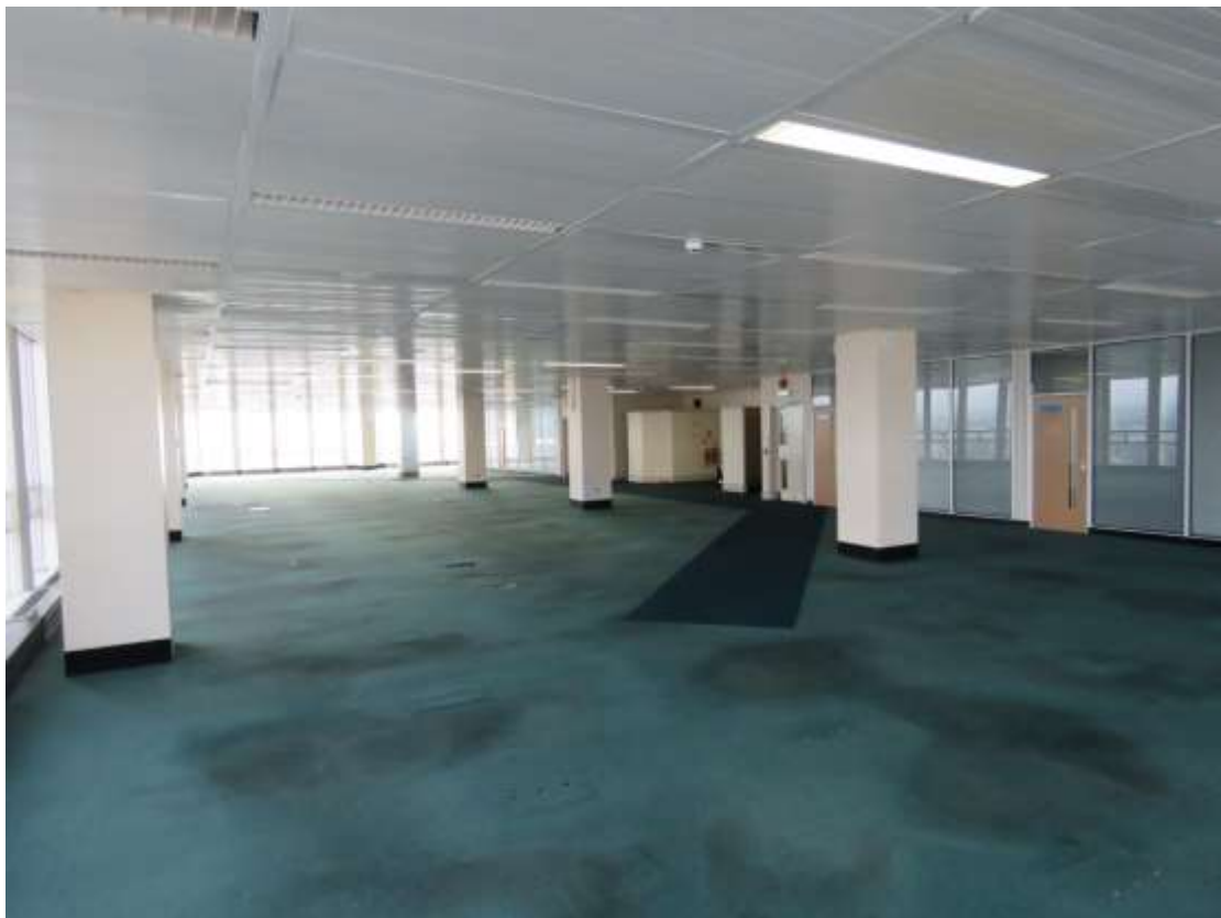
22-05 View south across office space.
