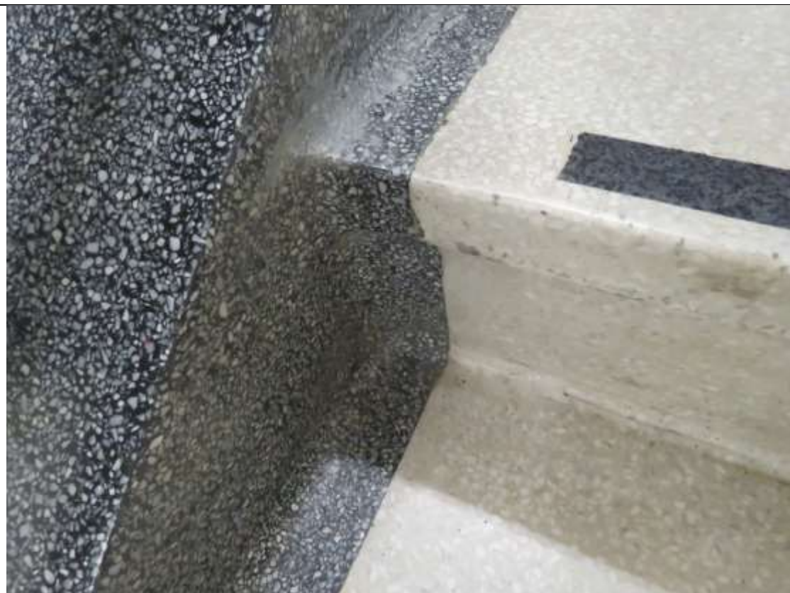
22-11 Detail of terrazzo floor covering to stairwell,
