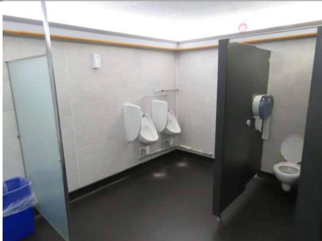
22-10 View within men's WC with original glazed screen and non-original sink, fixtures, fittings, wall finishes and vinyl floor covering.
