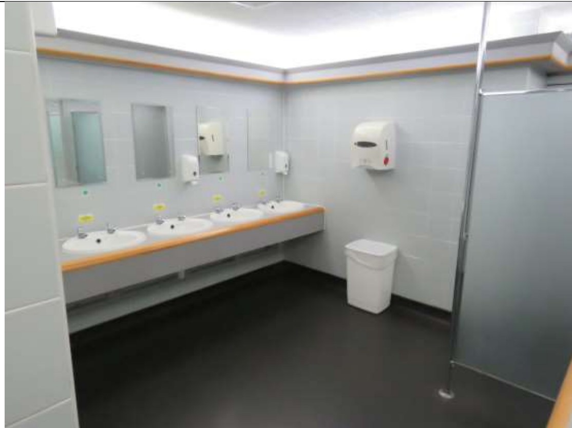
22-08 View within female WC looking towards the sink and original glazed screen to the right-hand side.
