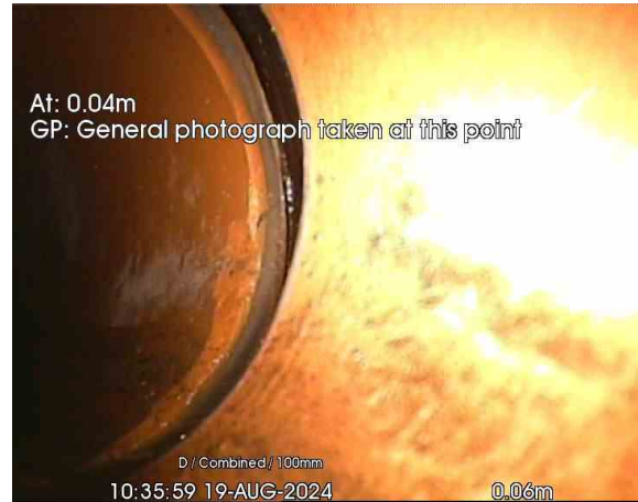
6_0-06m_103559.jpg, 00:00:11, 0.06 m General photograph taken at this point
