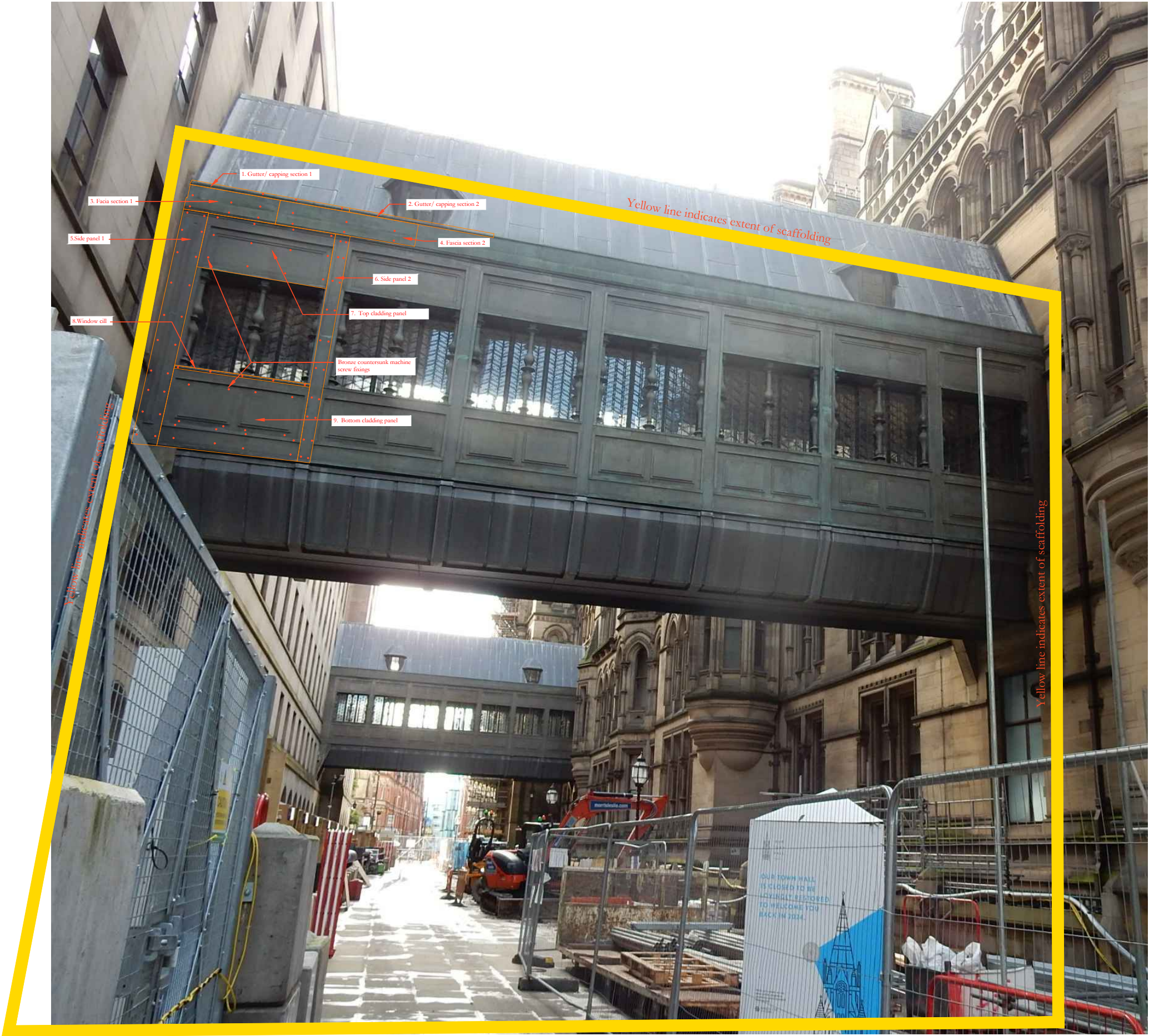
Yellow line indicates extent of scaffolding
