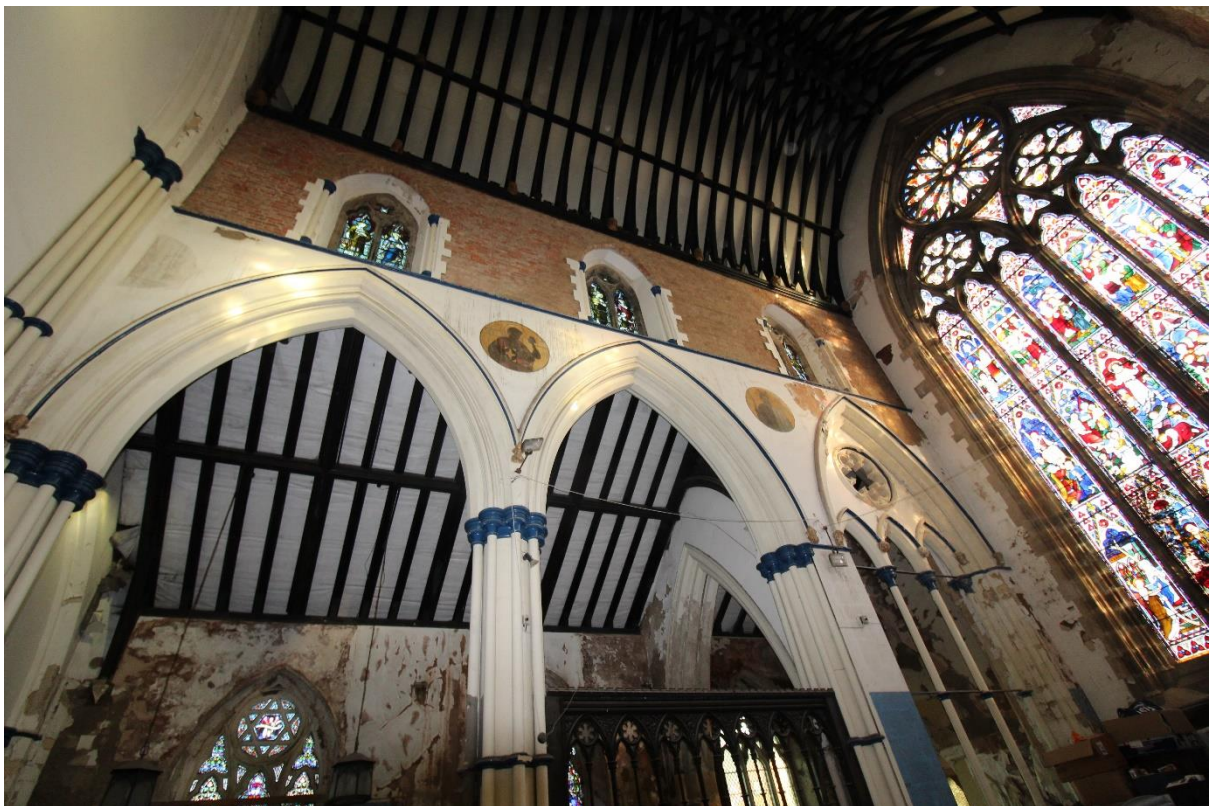
Plate 16 – Side Aisle & Clerestory
