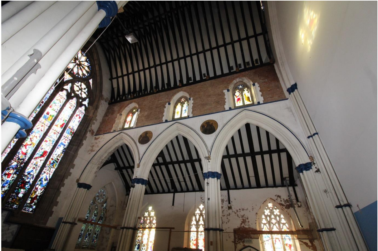
Plate 15 – Side Aisle & Clerestory
