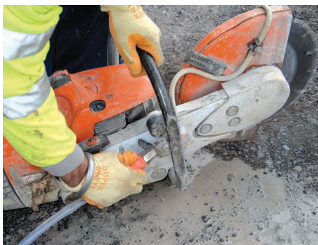
Figure 3 Water suppression on a cut-off saw
