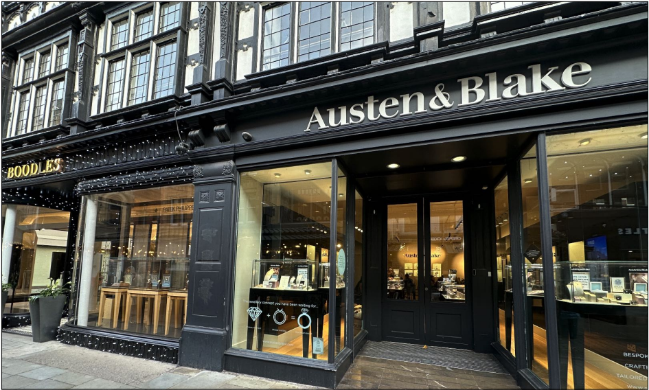
17 KING STREET EXISTING SHOPFRONT
