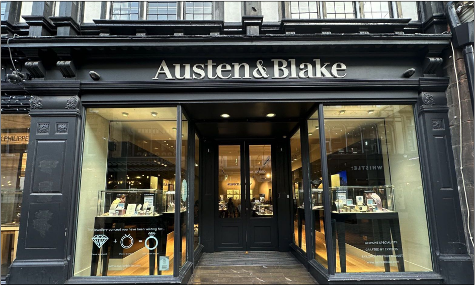
17 KING STREET EXISTING SHOPFRONT
