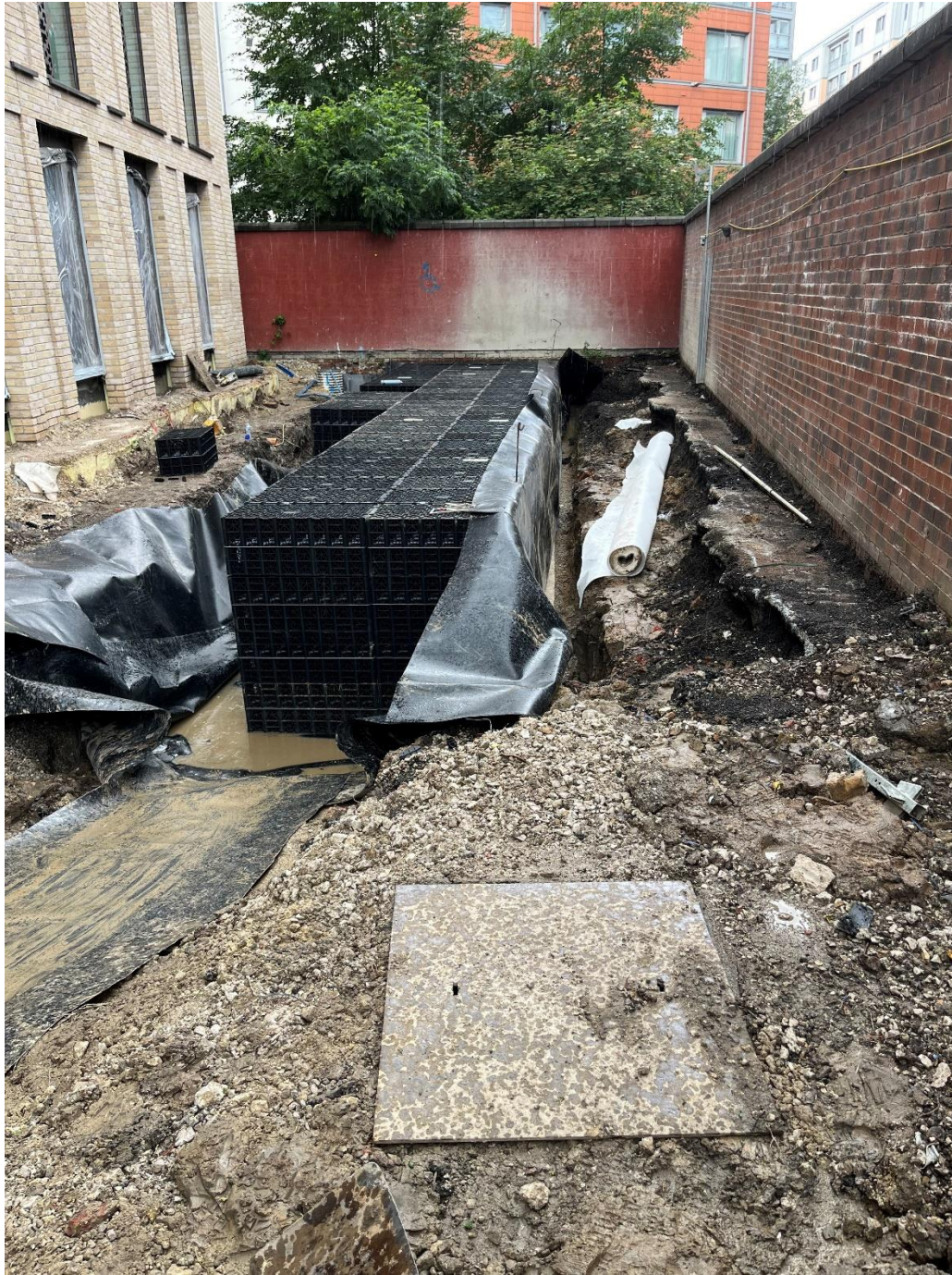
Figure D2 – Tank units being installed – Beginning of assembly process
