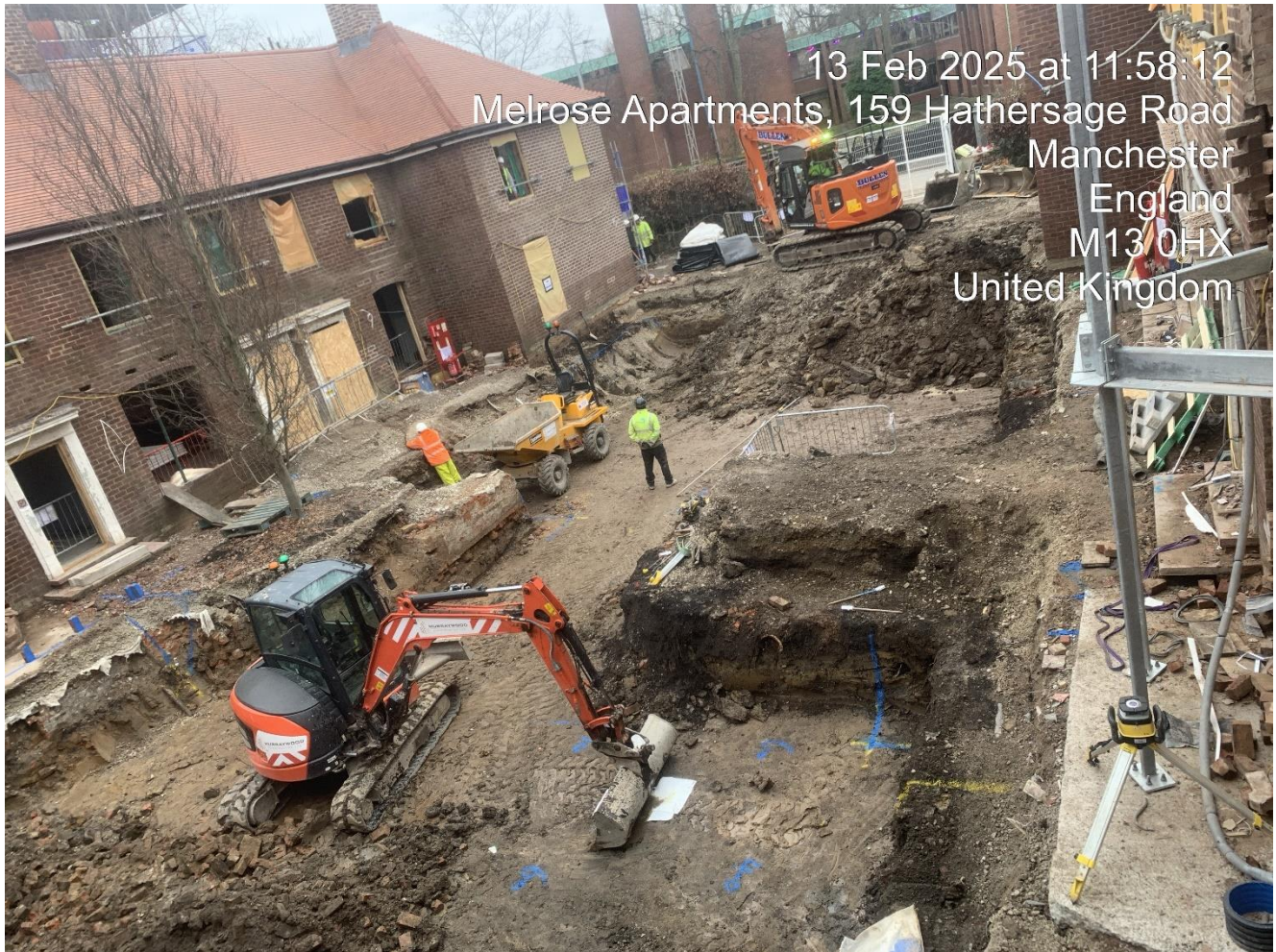
Figure D1 – Excavation works for drainage installation
