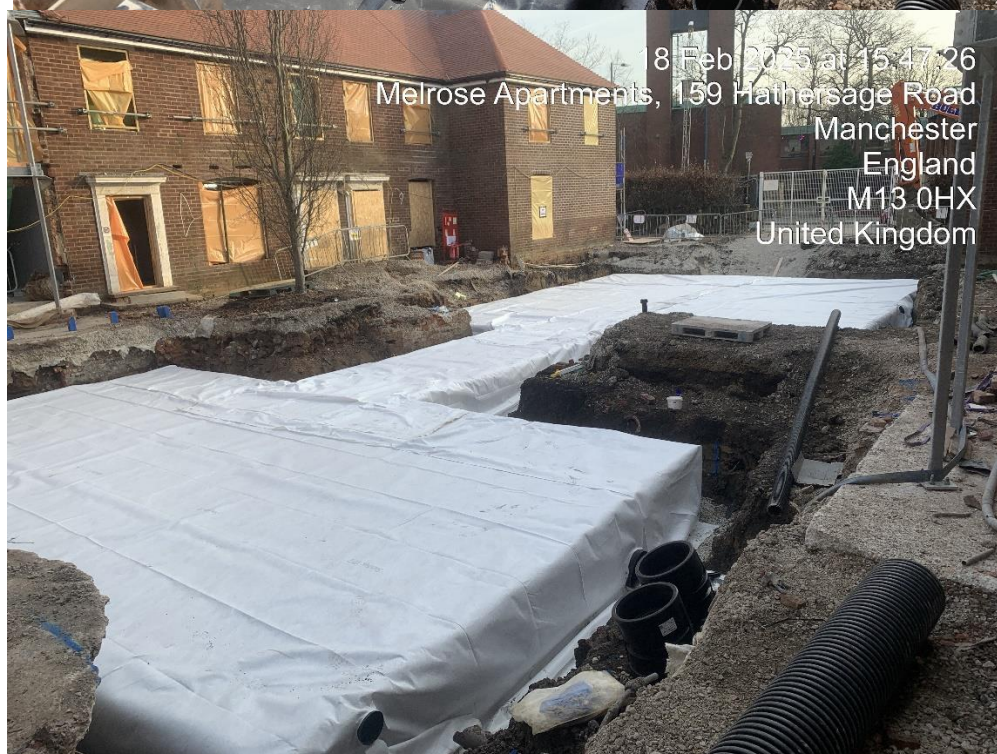
Figure D3 & D4 – Tank modules installed in final arrangement with geotextile layer
