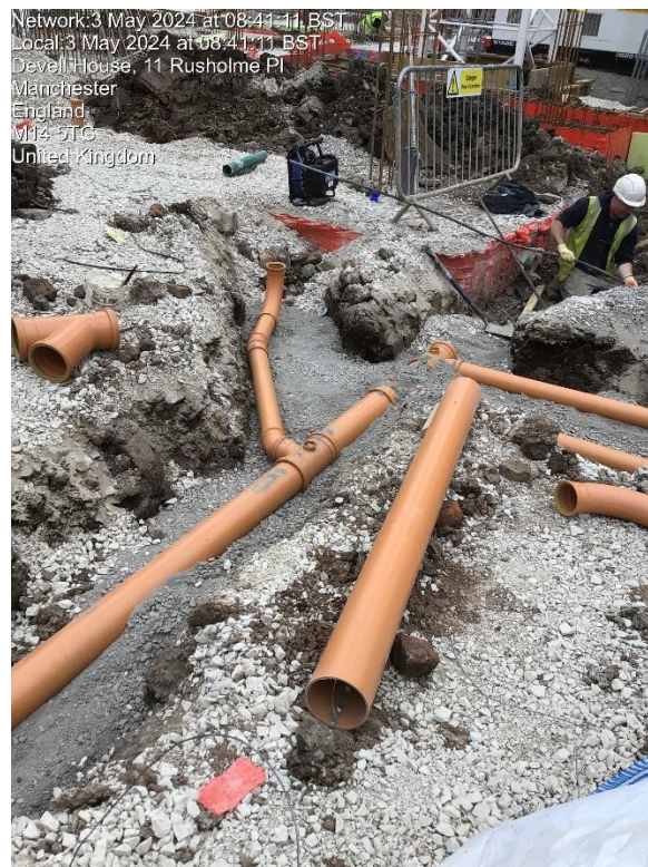
Figure D 6,7,8 & 9– Installation of Surface and Foul Water Pipework
