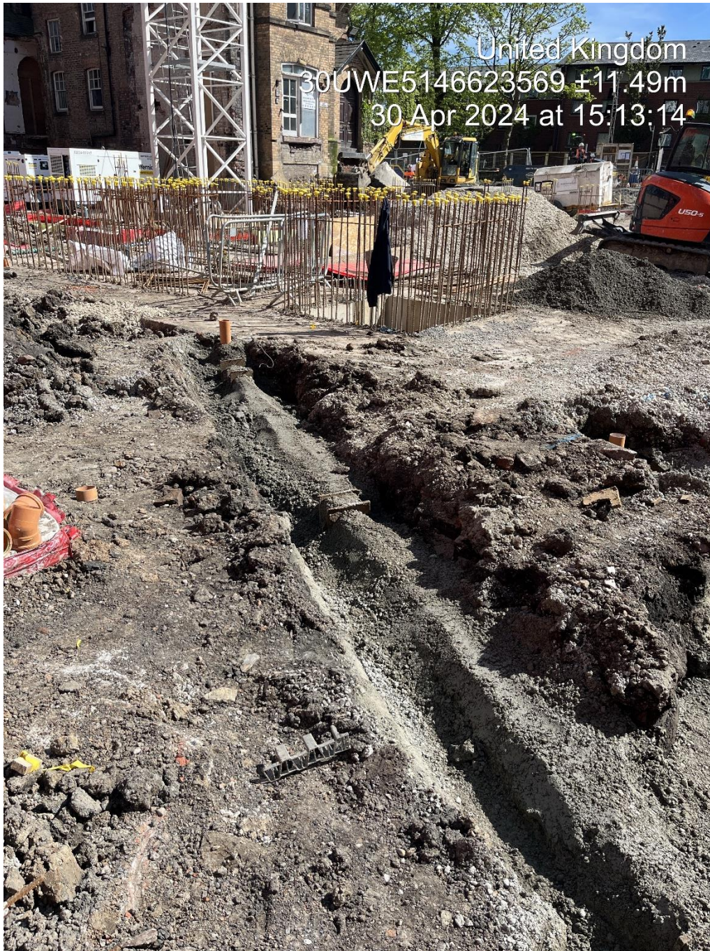
Figure D5 – Prepared trench with granular bedding for drainage pipe installation
