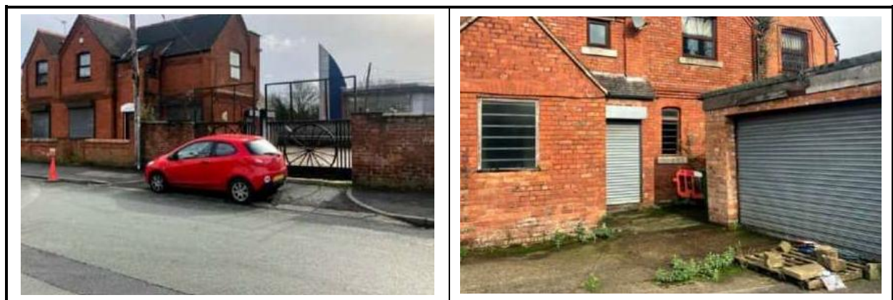
Figure 3 – General Site Photographs
