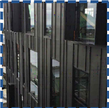
TYPE -VM ZINC STANDING SEAM CLADDING
