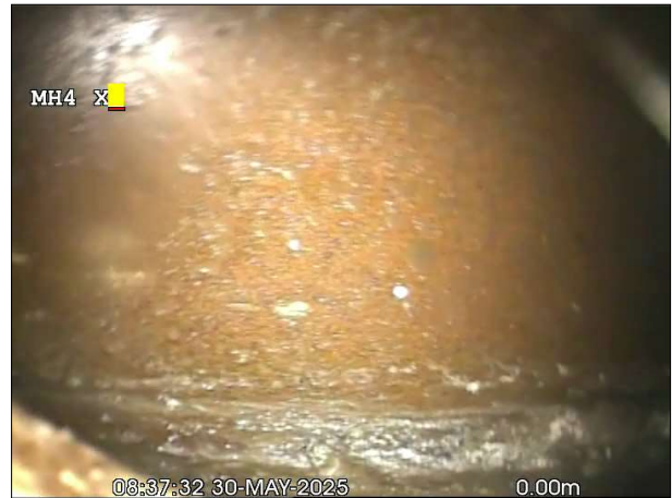
Photo: 54_5a, 00:00:00 0.1m, Finish Survey, Remark: Drops into sewer line.
