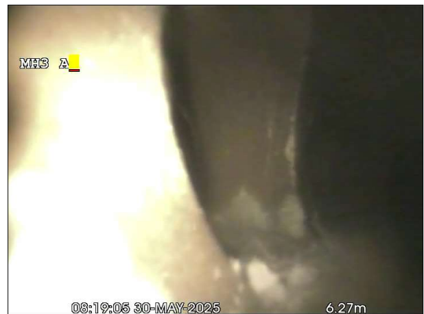
Photo: 30_10a, 00:00:00 6.3m, Junction at 09 o'clock, dia 150 mm
