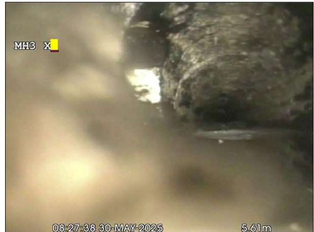
Photo: 3_5a, 00:00:00 5.8m, Junction at 09 o'clock, dia 225 mm
