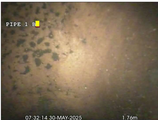
Photo: 103_8a, 00:00:00 2.2m, Finish Survey, Remark: Rest bend reached.
