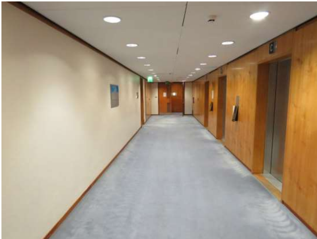
24-01 View of the lift lobby with cherry veneer panelling.
