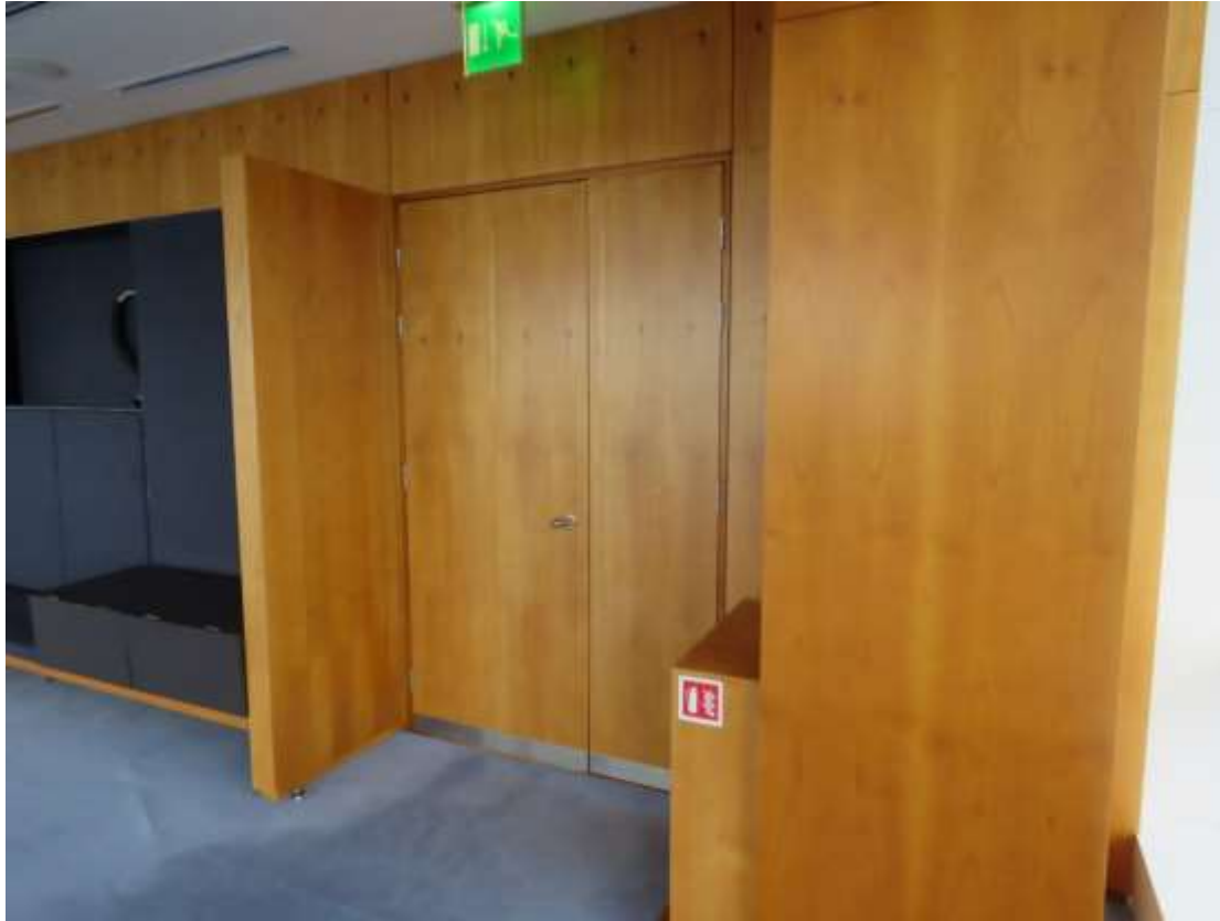
24-10 View of high quality timber panelling and doors (non-original).
