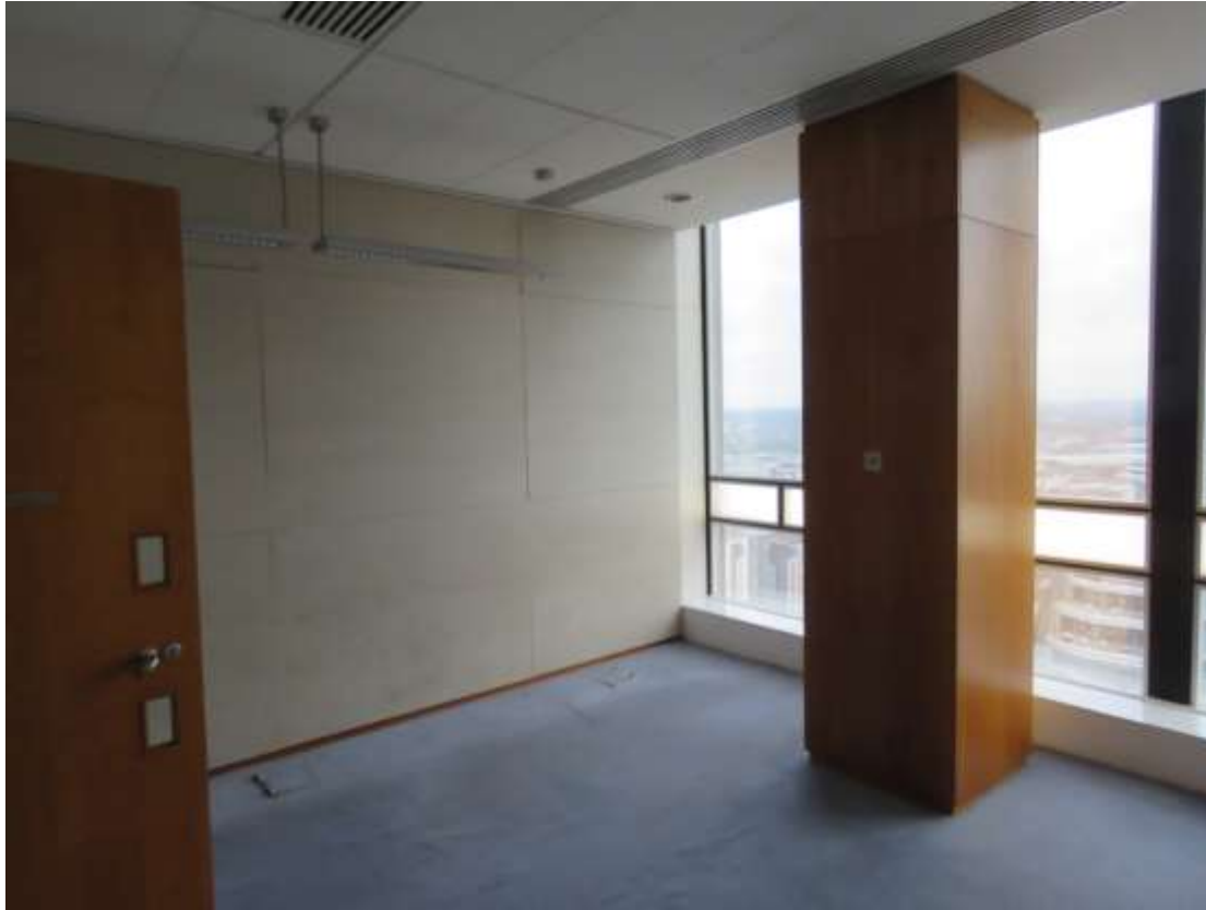
24-12 View within office with partition covered with white panelling.
