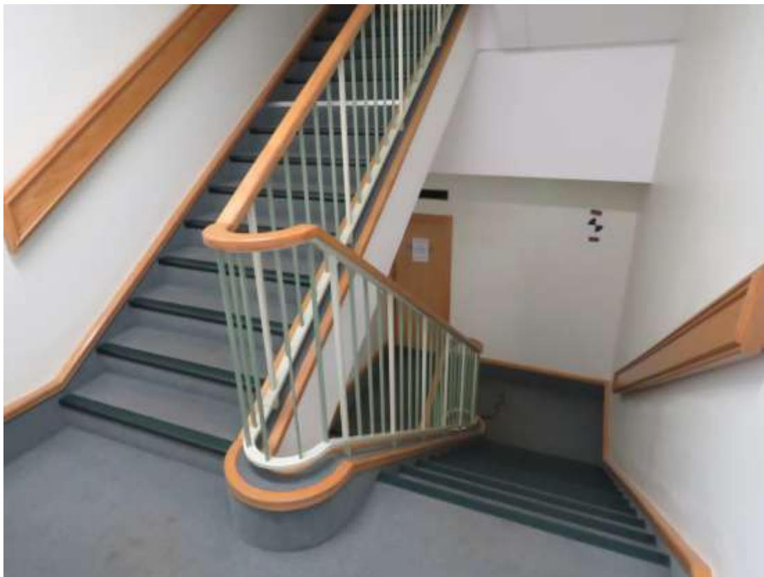
24-25 View within eastern stairwell.
