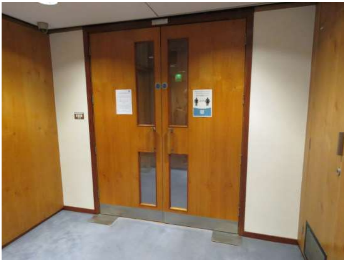
24-03 View of double doors between the lift lobby and foyer.
