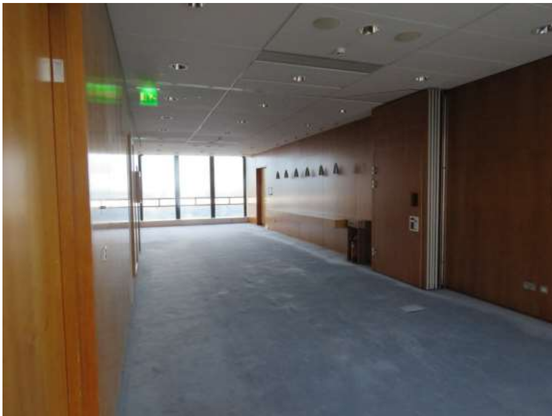
24-05 View north in ante-chamber outside the committee / board room.
