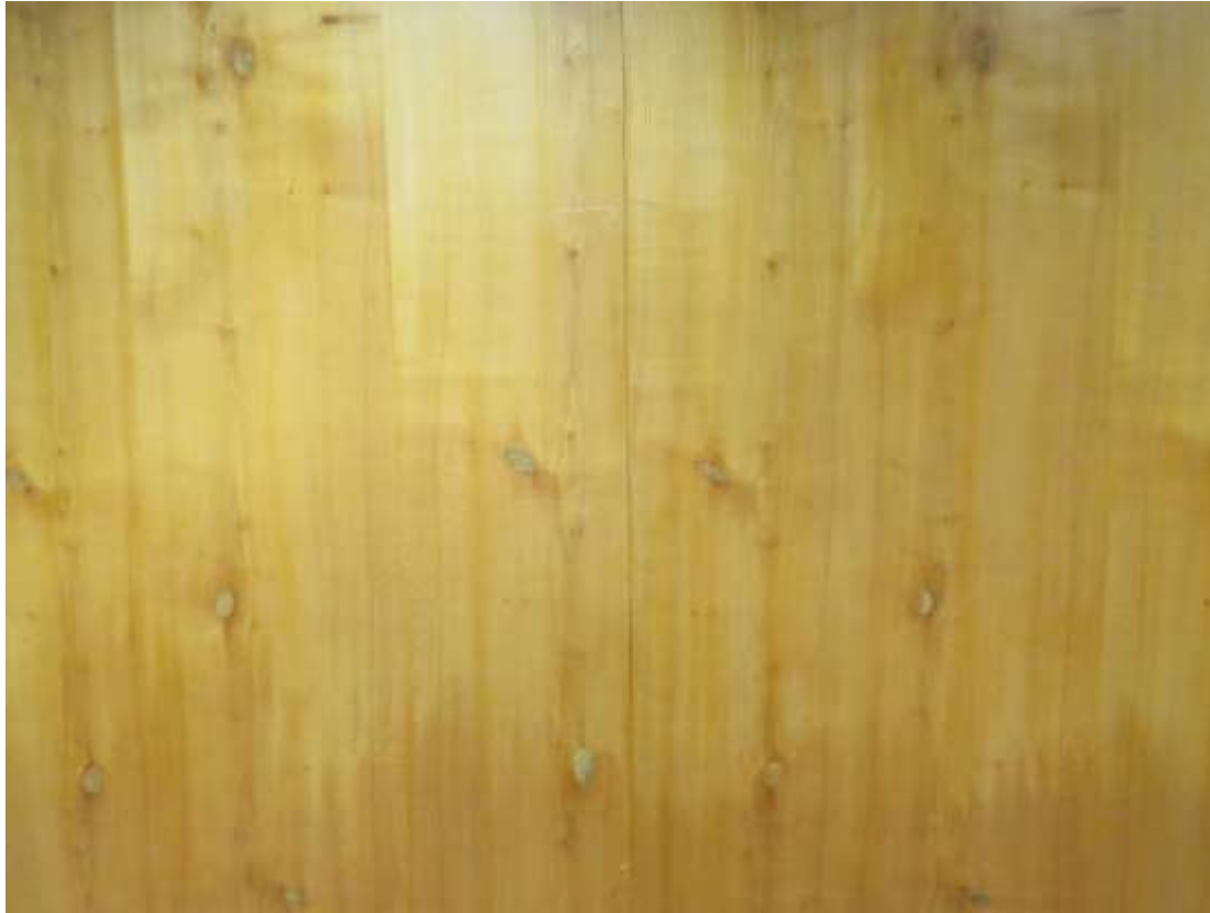
24-02 Close up view of cherry panelling to lift lobby.
