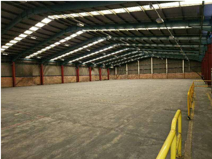
Photograph 7 – A view east, inside the main, central warehouse.
