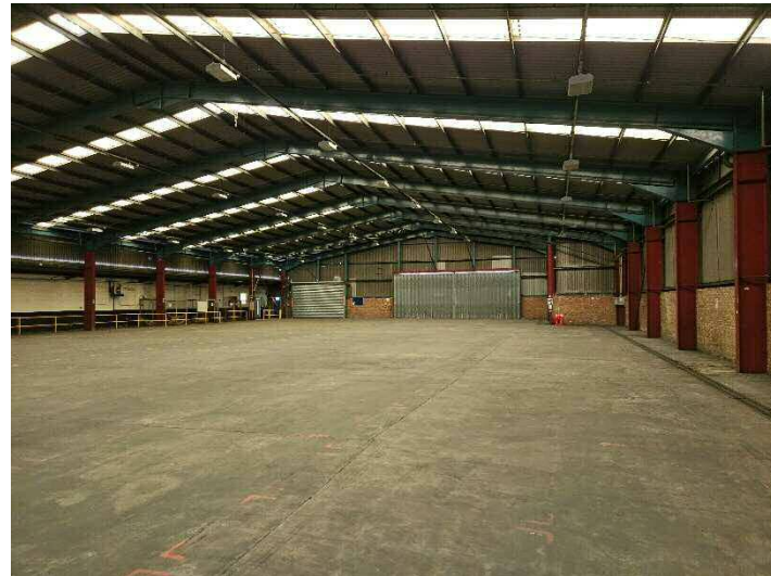
Photograph 8 – A view west, inside the main, central warehouse.
