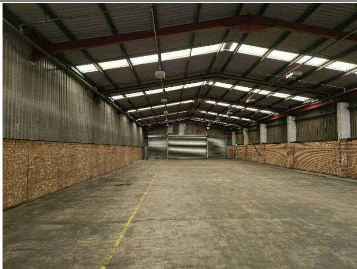
Photograph 9 – A view west, inside the smaller, northern warehouse.
