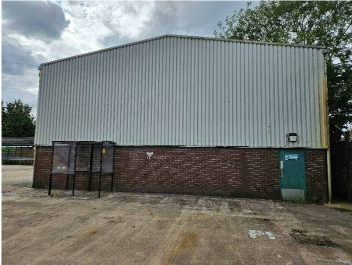
Photograph 17 – A view of the former location of AGST's and holes within the former vehicle maintenance building wall for now removed, connecting pipe work.
