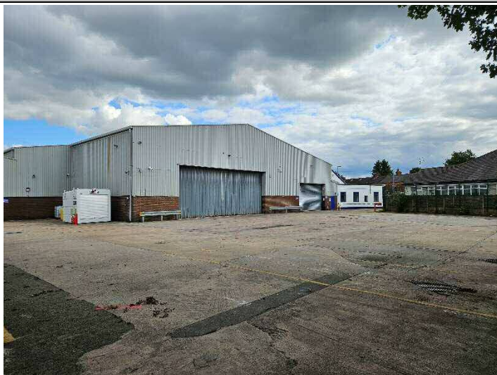
Photograph 11 – A view east, across the western yard area towards the main building.
