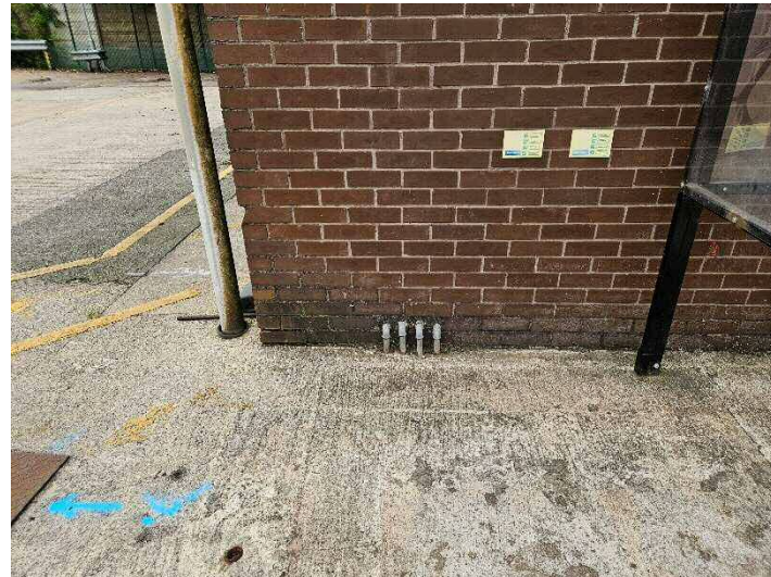
Photograph 16 – A view of pipe work exiting the building and potentially connecting with buried infrastructure..
