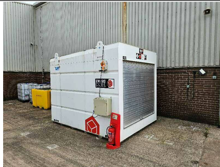
Photograph 10 – A view of the AGST an IBC's adjacent to the western elevation of the main warehouse.
