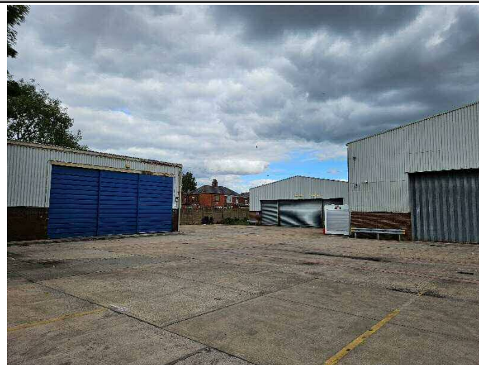
Photograph 12 – A view north, across the western yard area with the former vehicle repair building in the west.
