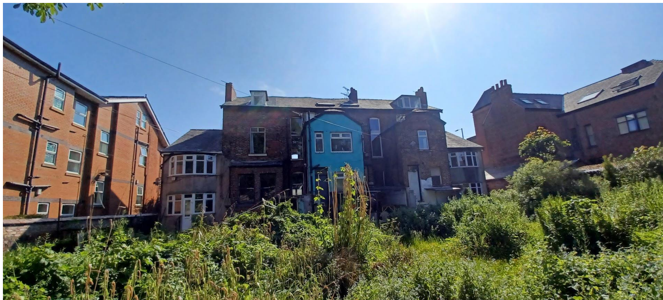
Rear elevation of the application site, 2025
