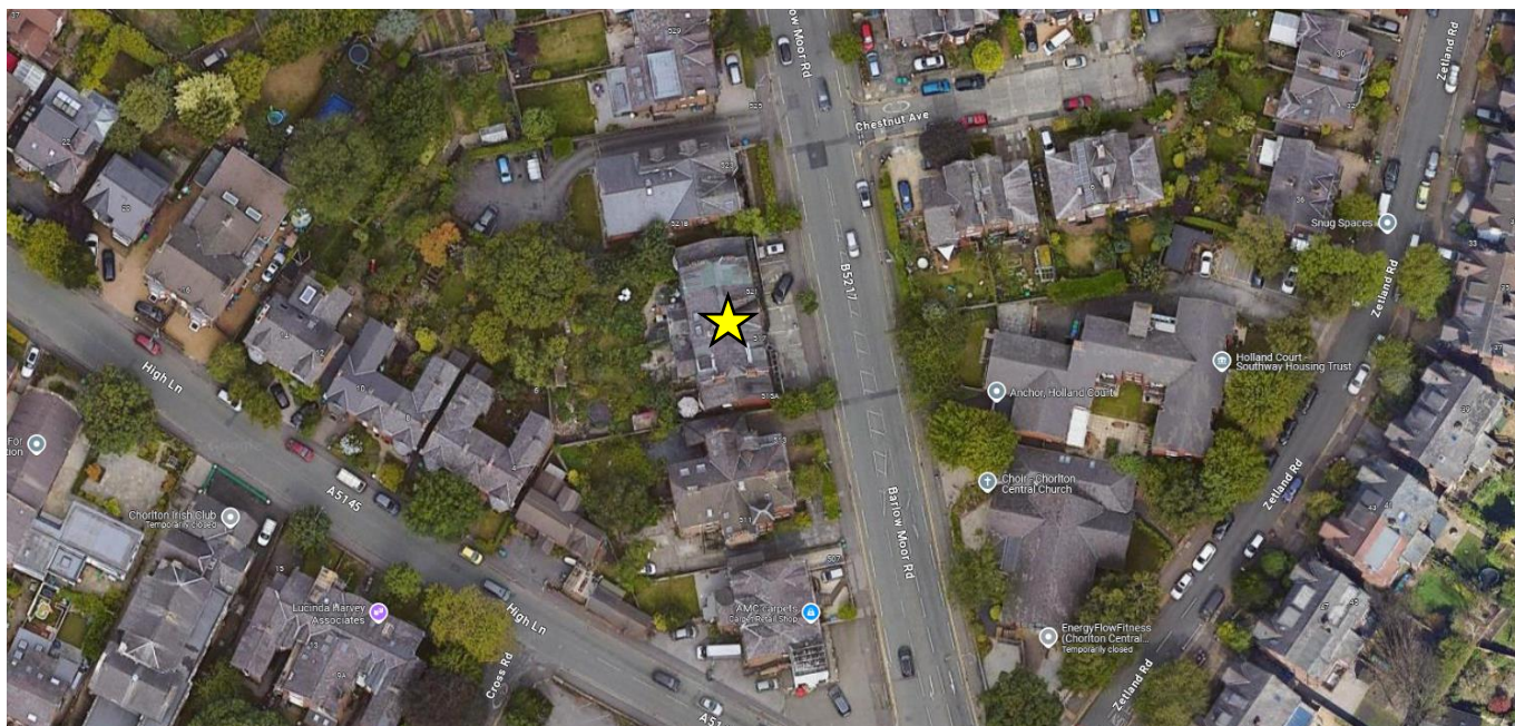
Application site, as viewed on Google Maps
