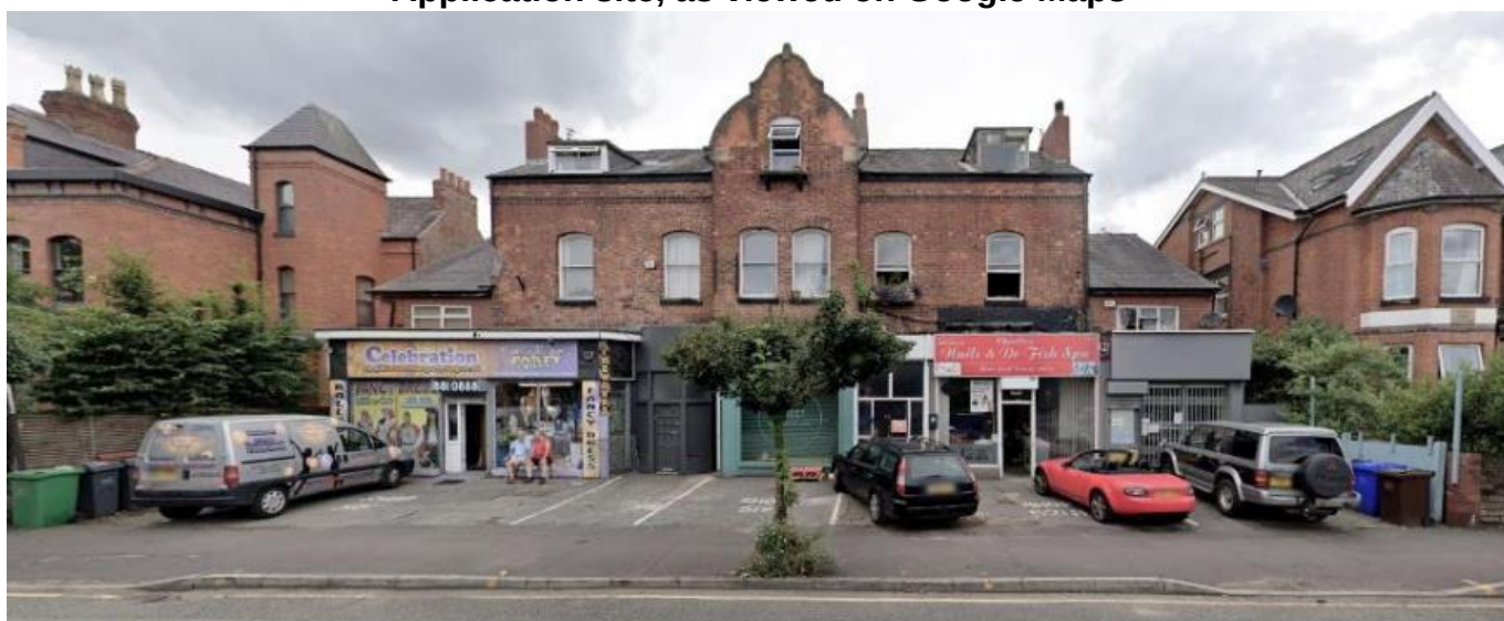
Front elevation of the application site, as viewed from Barlow Moor Road, c. 2021
