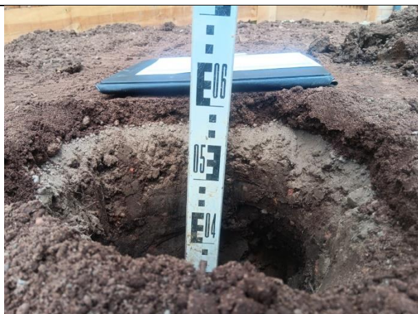
Photograph 53: Evidence of suitably chemically validated soil cover to 600mm in the rear garden of plot 20. Note that soil was laid over a period of time, therefore was partially dry by time of inspection.
