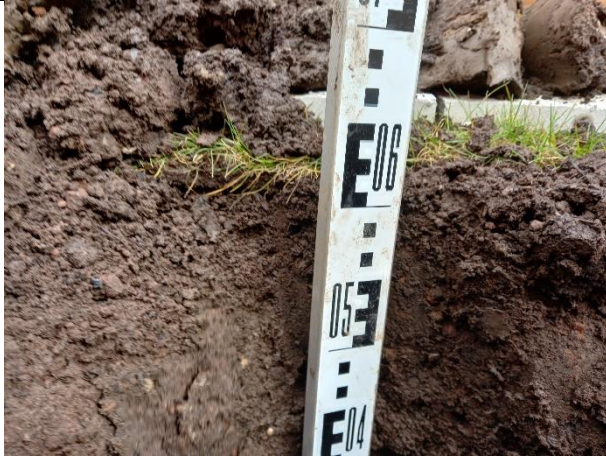
Photograph 49: Evidence of suitably chemically validated soil cover to 600mm in the rear garden of plot 19.
