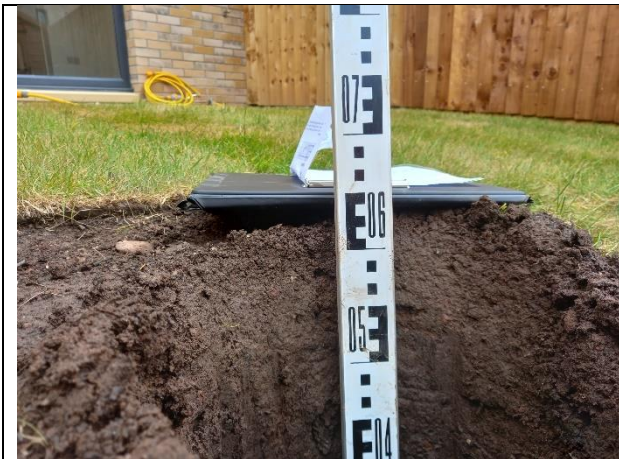
Photograph 40: Evidence of suitably chemically validated soil cover to 620mm in the rear garden of plot 17.
