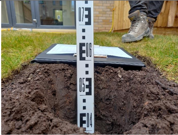
Photograph 58: Evidence of suitably chemically validated soil cover to 600mm in the rear garden of plot 21.
