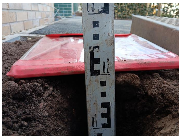
Photograph 48 Evidence of suitably chemically validated topsoil with a minimum of 150mm growing medium in the shared front strip of Plot 18-19 over MOT.
