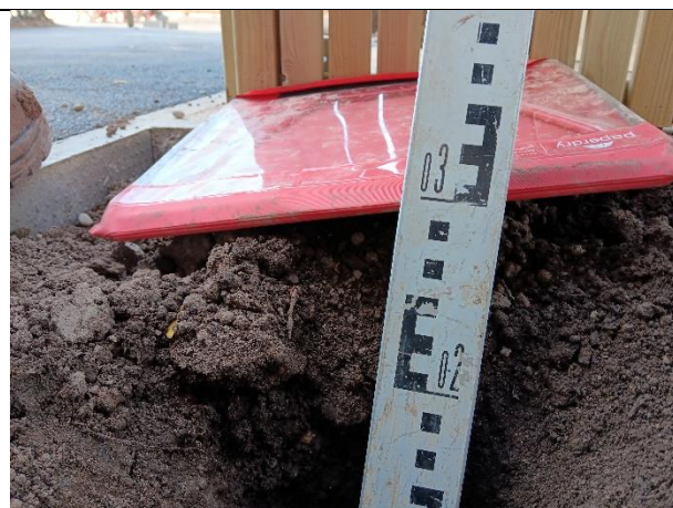
Photograph 31: Evidence of suitably chemically validated topsoil with a minimum of 150mm growing medium in the shared front strip of Plot 14-15 over MOT.
