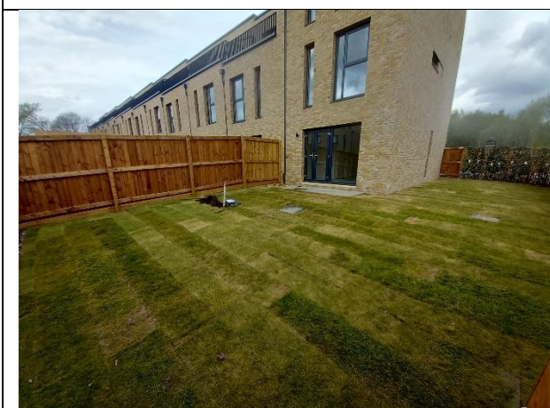
Photograph 64: View showing rear of plot 22.
