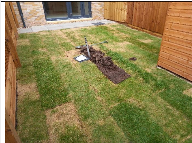
Photograph 38: View showing rear of plot 16.
