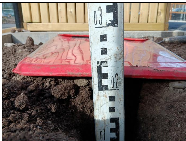
Photograph 9: Evidence of suitably chemically validated topsoil with a minimum of 150mm growing medium in the shared front strip of Plot 10-11 over MOT.
