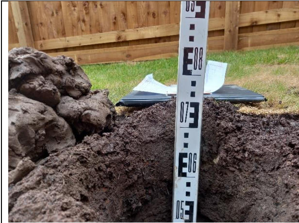
Photograph 36: Evidence of suitably chemically validated soil cover to 700mm in the rear garden of plot 16.
