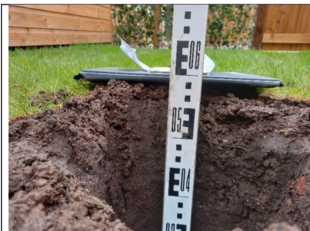
Photograph 14: Evidence of suitably chemically validated soil cover to 600mm in the rear garden of plot 12.
