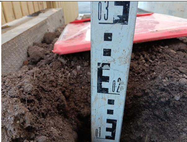
Photograph 9: Evidence of suitably chemically validated topsoil with a minimum of 150mm growing medium in the shared front strip of Plot 16-17 over MOT.
