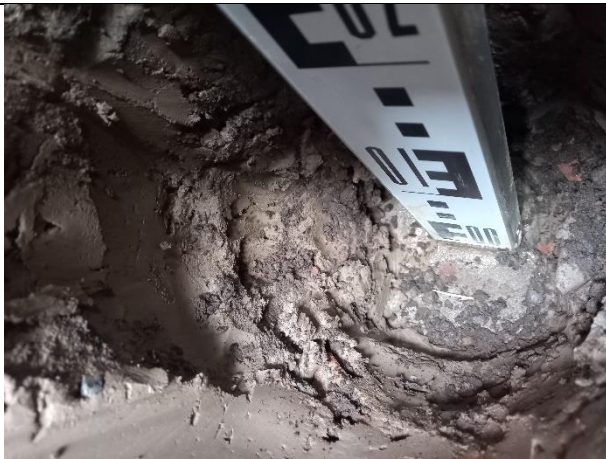
Photograph 59: Evidence of geotextile membrane in plot 21.
