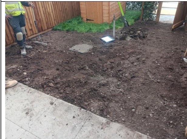
Photograph 7: View showing rear of plot 10.
