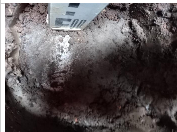
Photograph 15: Evidence of geotextile membrane in plot 12.
