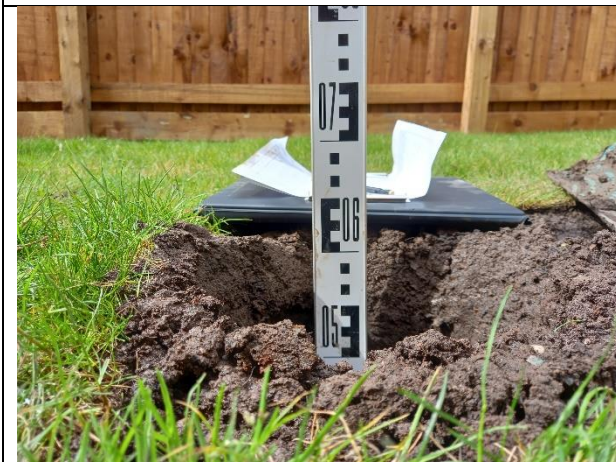
Photograph 27: Evidence of suitably chemically validated soil cover to 620mm in the rear garden of plot 14.
