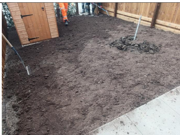
Photograph 55: View showing rear of plot 20.
