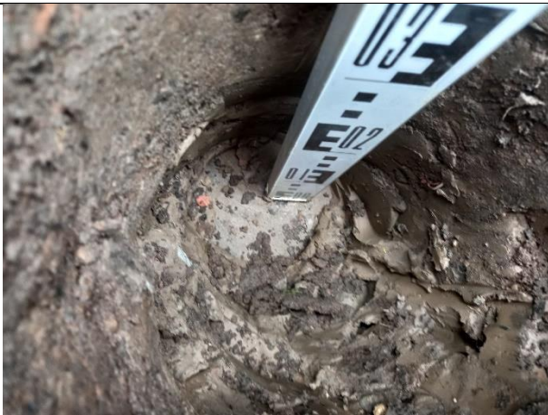
Photograph 45: Evidence of geotextile membrane in plot 18.
