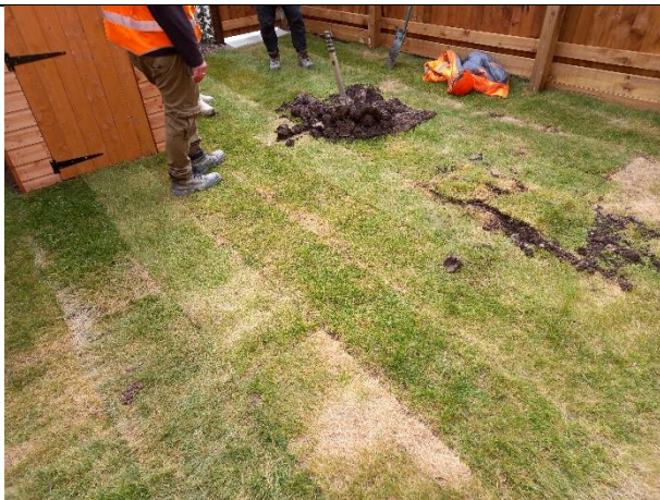
Photograph 51: View showing rear of plot 19.
