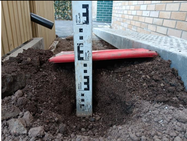
Photograph 57: Evidence of suitably chemically validated topsoil with a minimum of 150mm growing medium in the shared front strip of Plot 20-21 over MOT.
