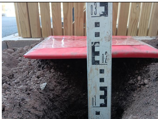
Photograph 18: Evidence of suitably chemically validated topsoil with a minimum of 150mm growing medium in the shared front strip of Plot 12-13 over MOT.
