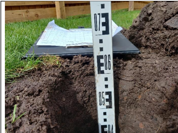
Photograph 32: Evidence of suitably chemically validated soil cover to 640mm in the rear garden of plot 15.
