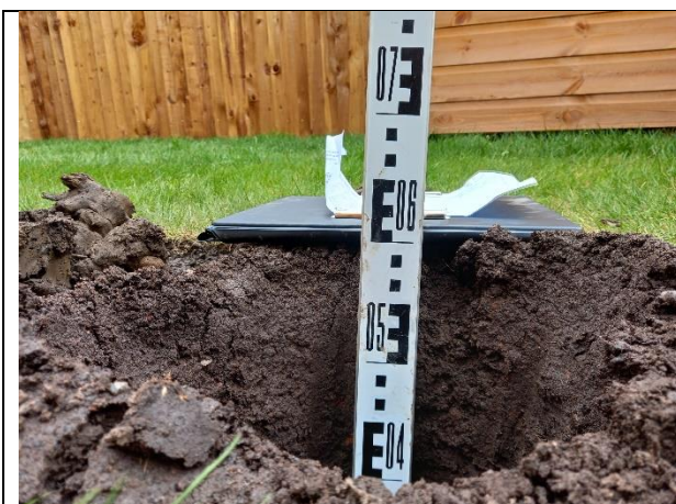
Photograph 10: Evidence of suitably chemically validated soil cover to 600mm in the rear garden of plot 11.
