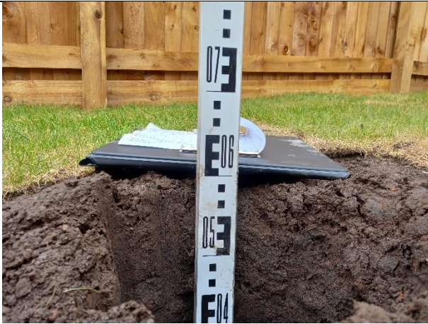
Photograph 44: Evidence of suitably chemically validated soil cover to 600mm in the rear garden of plot 18.
