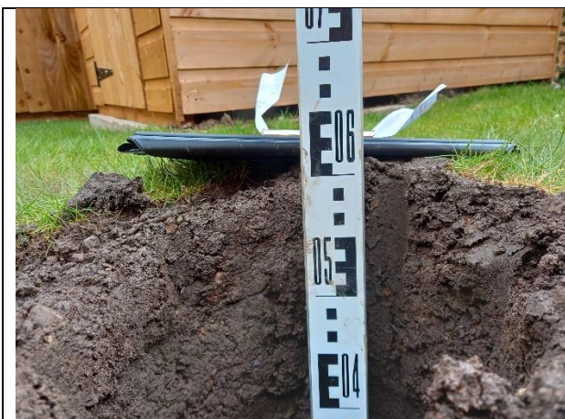
Photograph 23: Evidence of suitably chemically validated soil cover to 600mm in the rear garden of plot 13.
