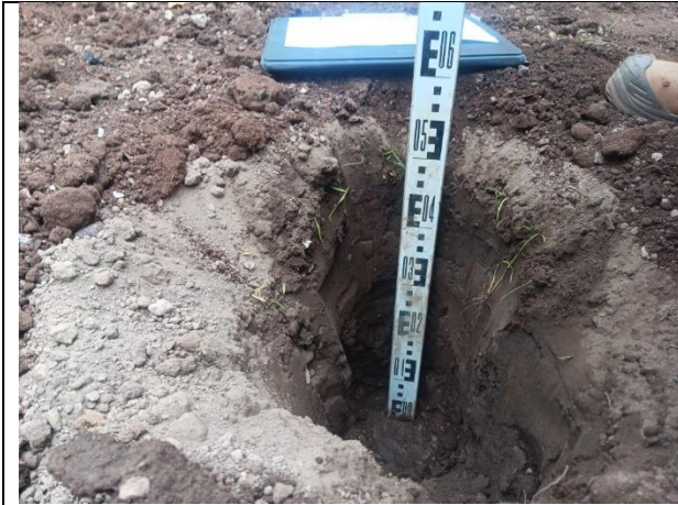
Photograph 5: Evidence of suitably chemically validated soil cover to 600mm in the rear garden of plot 10.
