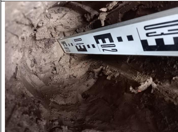
Photograph 37: Evidence of geotextile membrane in plot 16.
