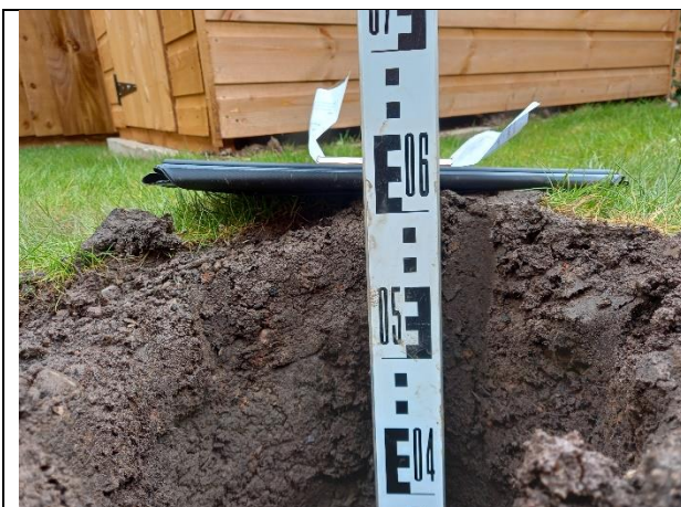
Photograph 19: Evidence of suitably chemically validated soil cover to 600mm in the rear garden of plot 13.
