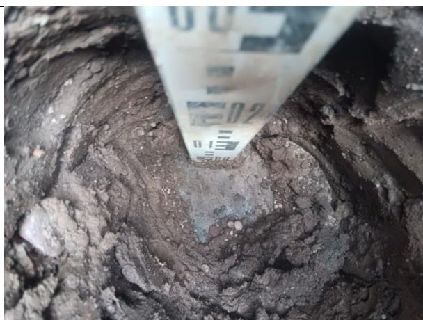
Photograph 54: Evidence of geotextile membrane in plot 20.
