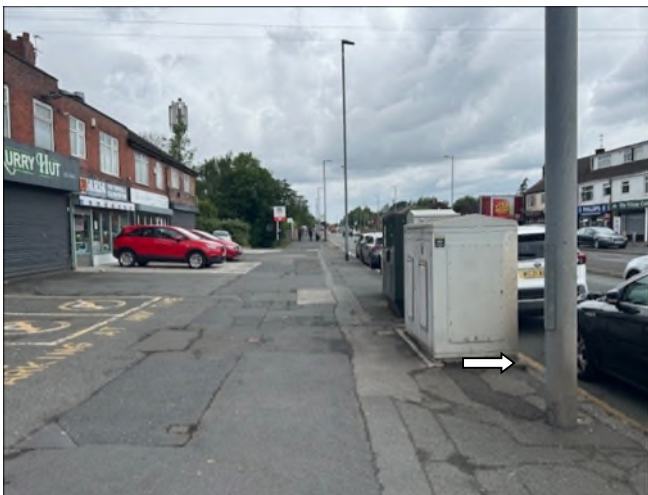
View looking westwards (arrow indicating position of proposed installation)
