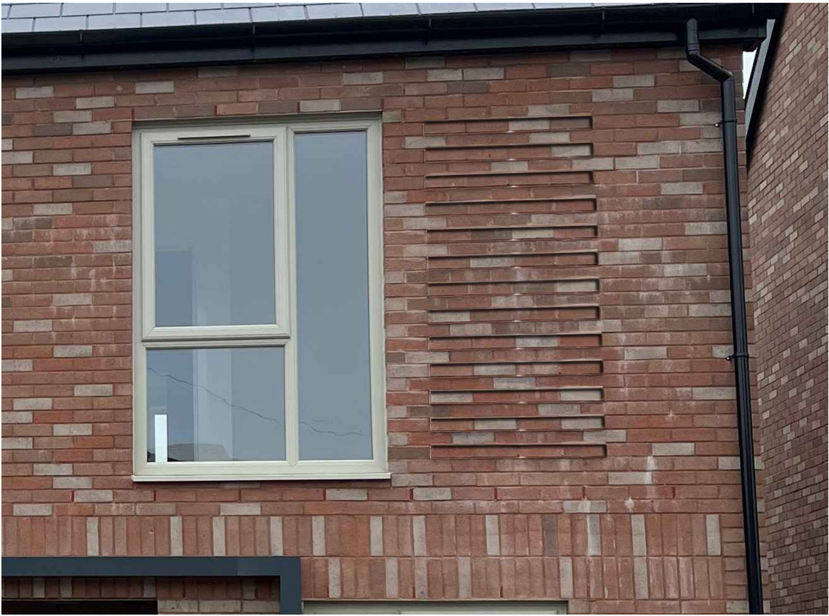
3. Brick Detailing Recessed Horizontal Brick Feature Bands
