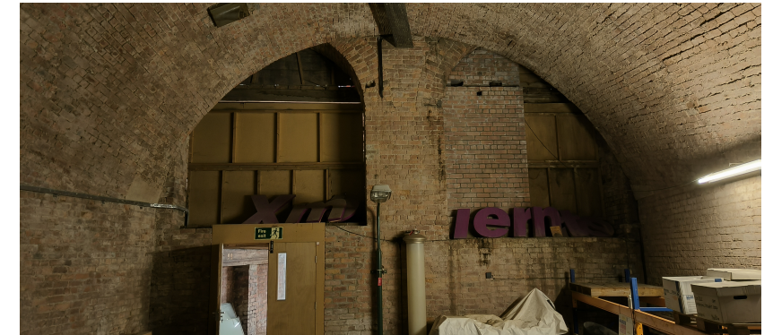
Photo 1 SIM.SB.-1.15 PINs A1SB-115A and A1SB-115B
