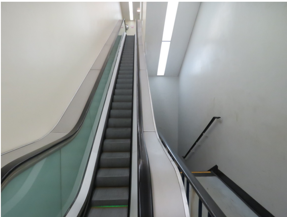
B1-01 View from the base of the escalator looking up to ground floor, note the stairs to the right hand side go down to B3.
