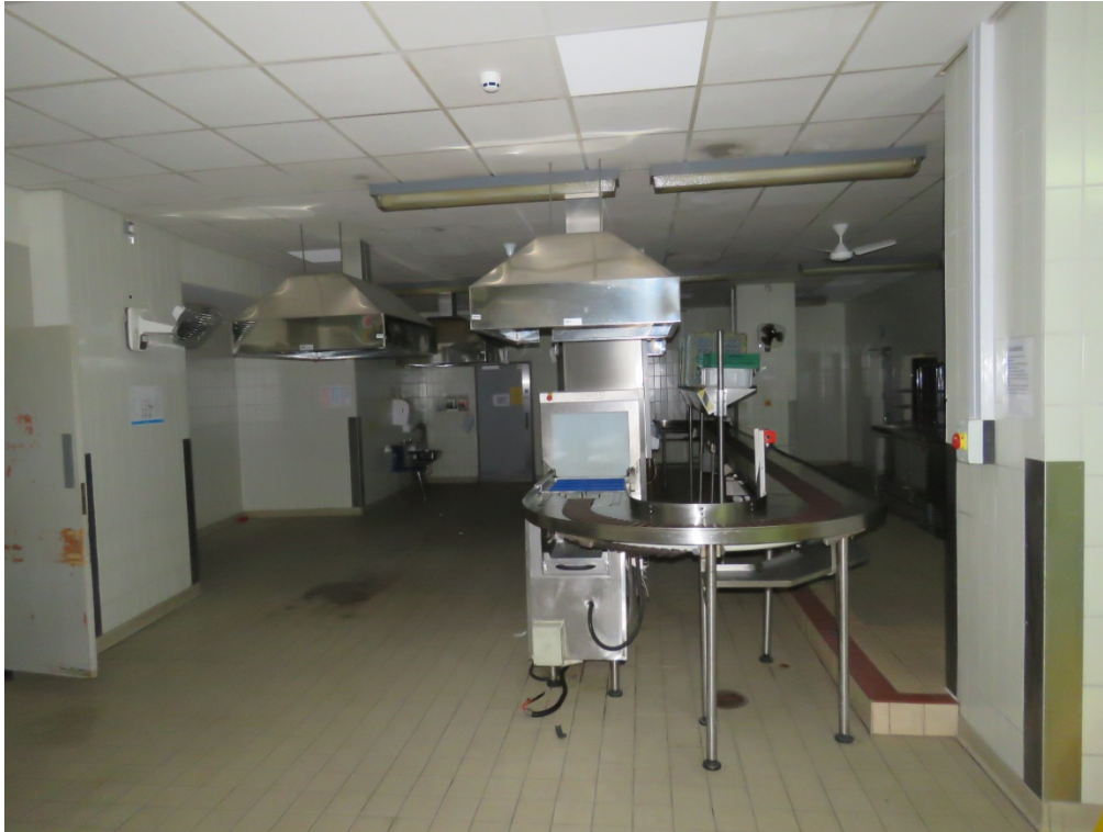
B1-14 View of the kitchen pot washing facilities directly north of the collection point.
