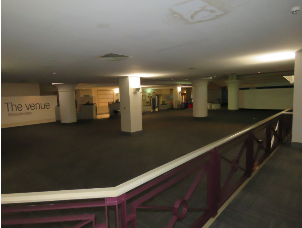
B1-12 View from raised seating area looking south across the canteen seating area back towards the foyer.
