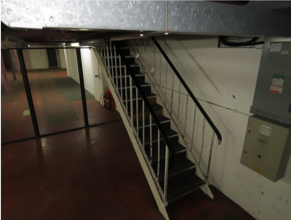
B1-26 Metal stairs leading to B1 upper.
