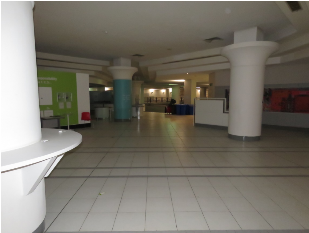
B1-03 View from the foyer of the canteen towards the canteen.
