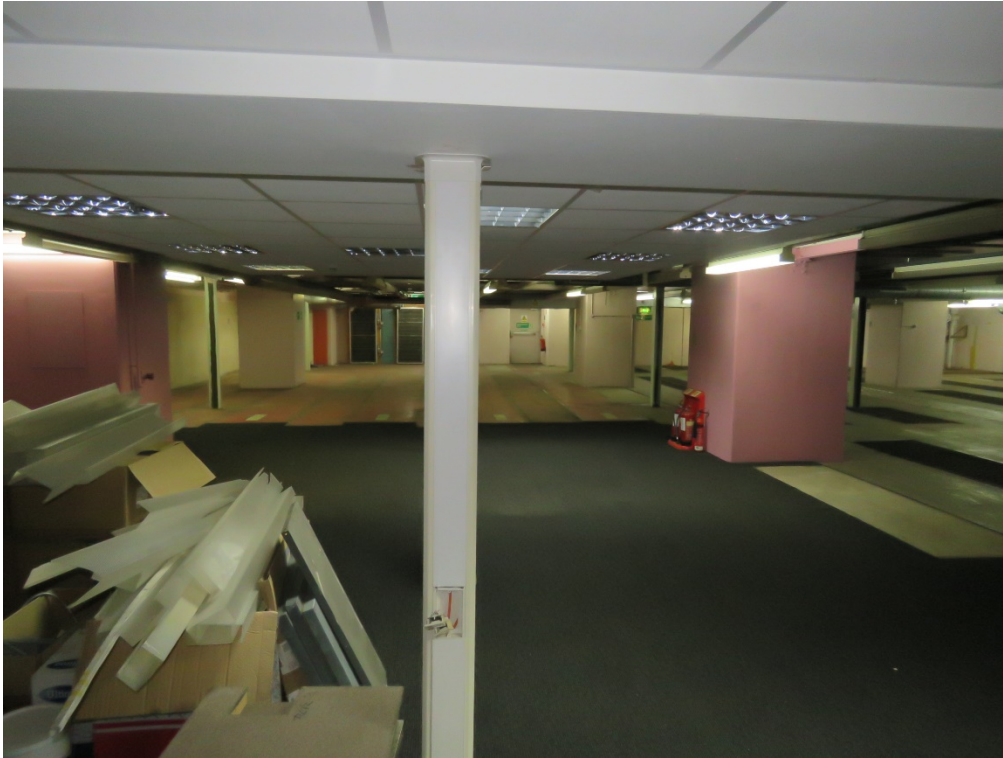
B1-20 Looking north within the document store.
