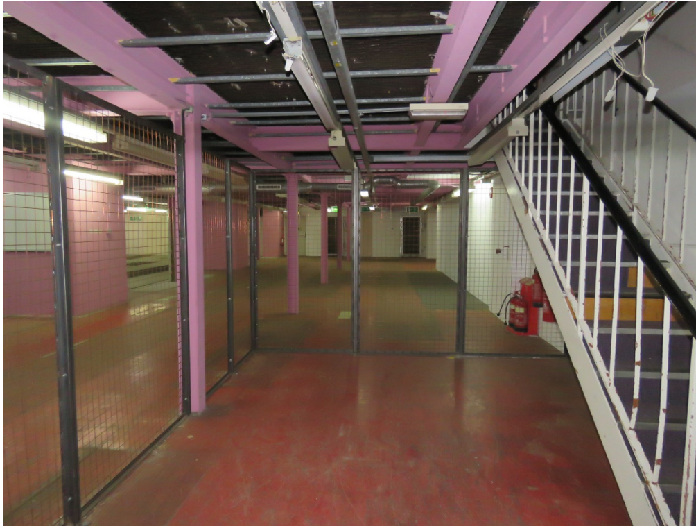
B1-24 View south with stairs up to the B1 upper level.
