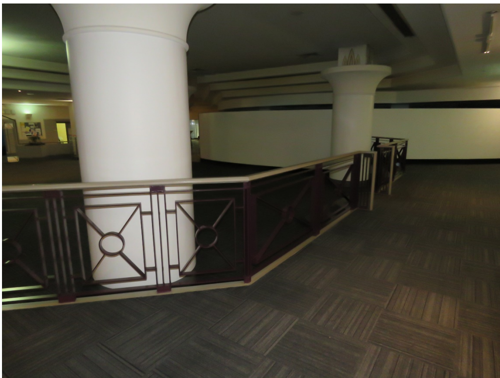
B1-11 View of handrail between the raised seating area and lower seating area.
