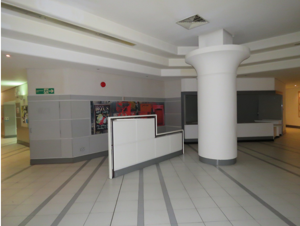
B1-06 View looking east within foyer with half height partition / screen and desk. Note the square columns now clad to be circular.
