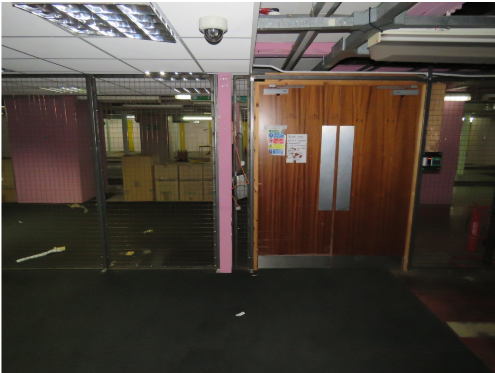
B1-19 View of the document store on entrance.
