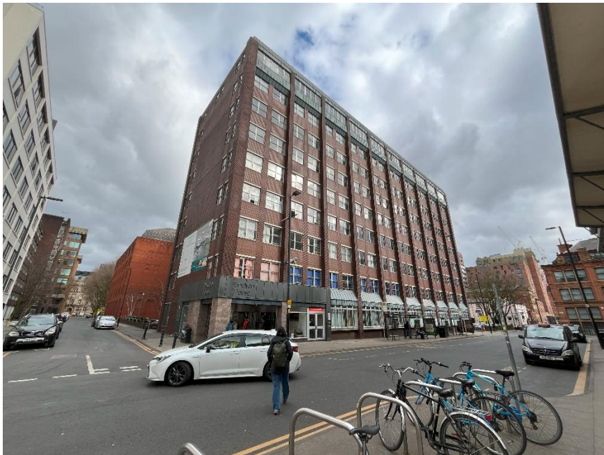
Figure 3: View of Boulton House from along Chorlton Street.
