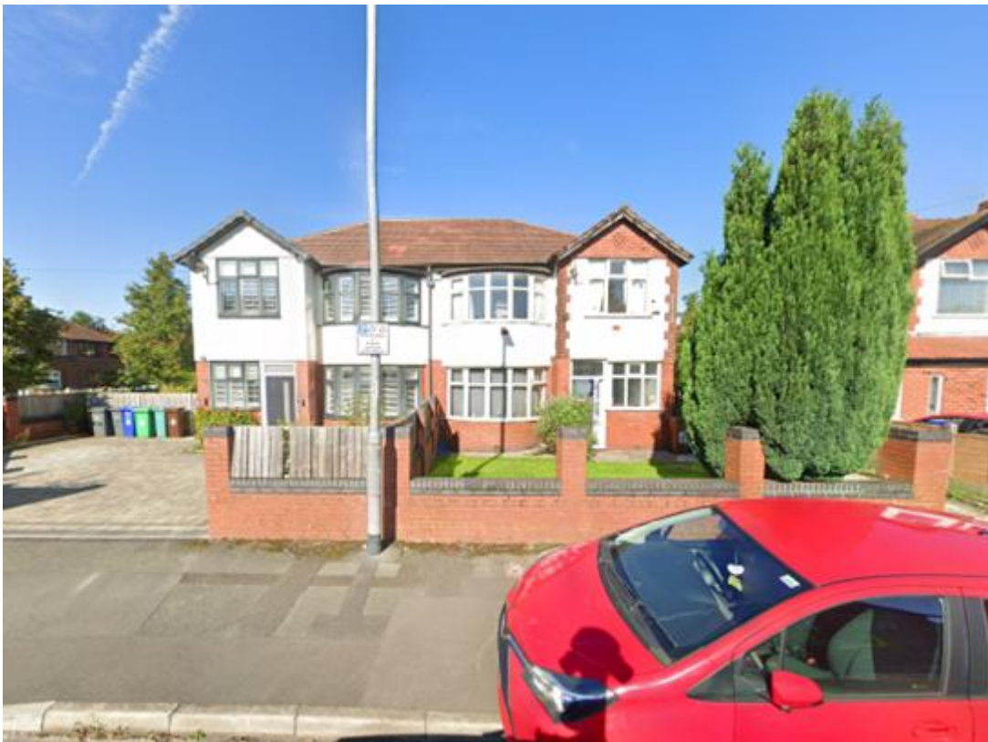
Image 3: Photograph of the front elevation of the site as viewed from Abberton Road with No. 14 located to the right hand side.
