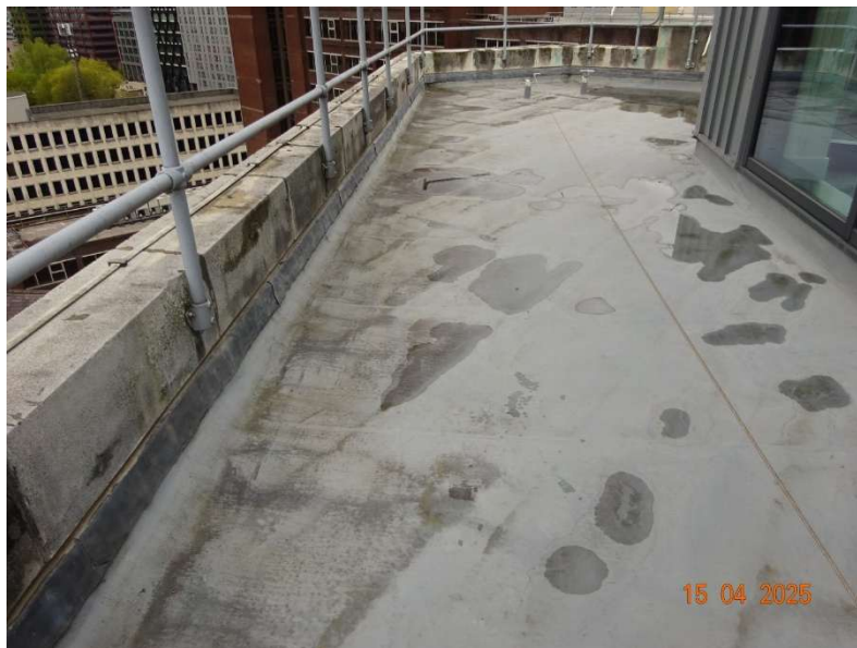
Photograph 19 6 th floor roof (looking west)
