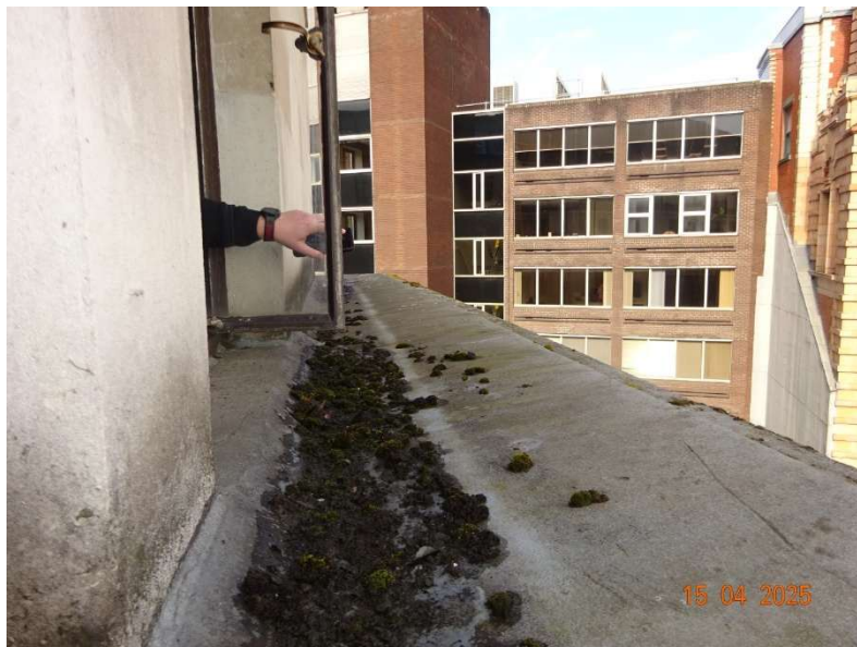
Photograph 2 North elevation 5 th floor ledge (looking west)
