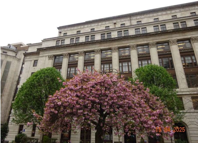
Photograph 21 View of north elevation (left-hand side)
