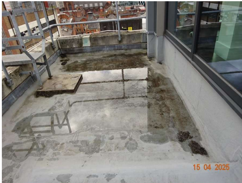
Photograph 5 6 th floor roof (looking south)
