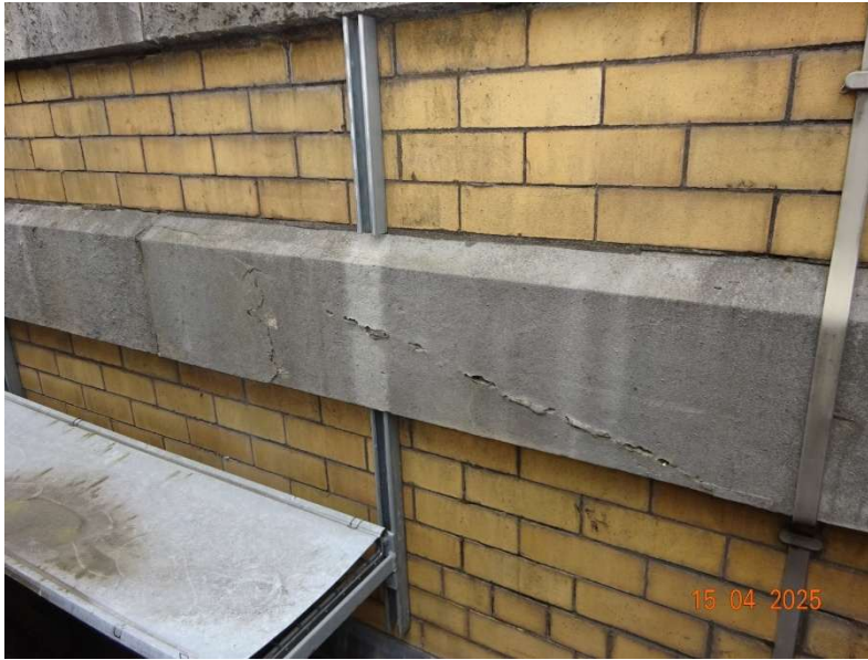
Photograph 12 North elevation parapet wall
