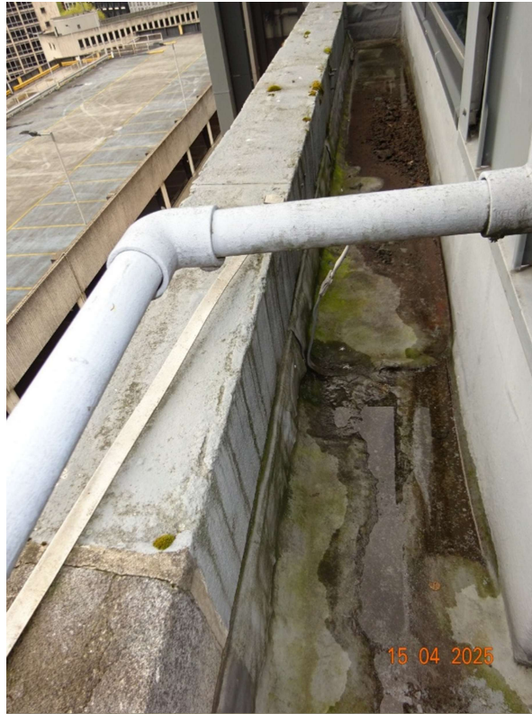
Photograph 8 6 th floor roof (looking west)
