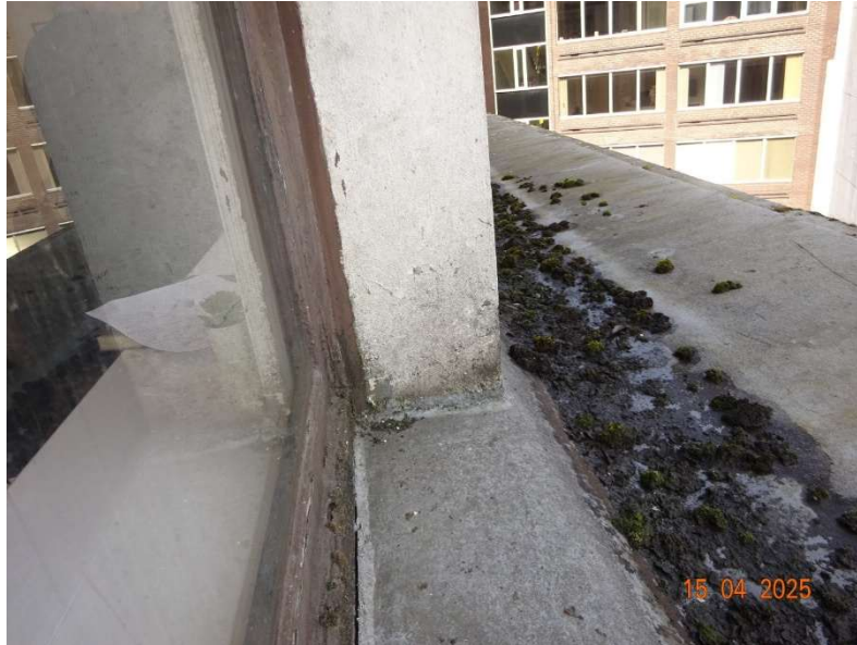
Photograph 1 North elevation 5 th floor ledge (looking west)
