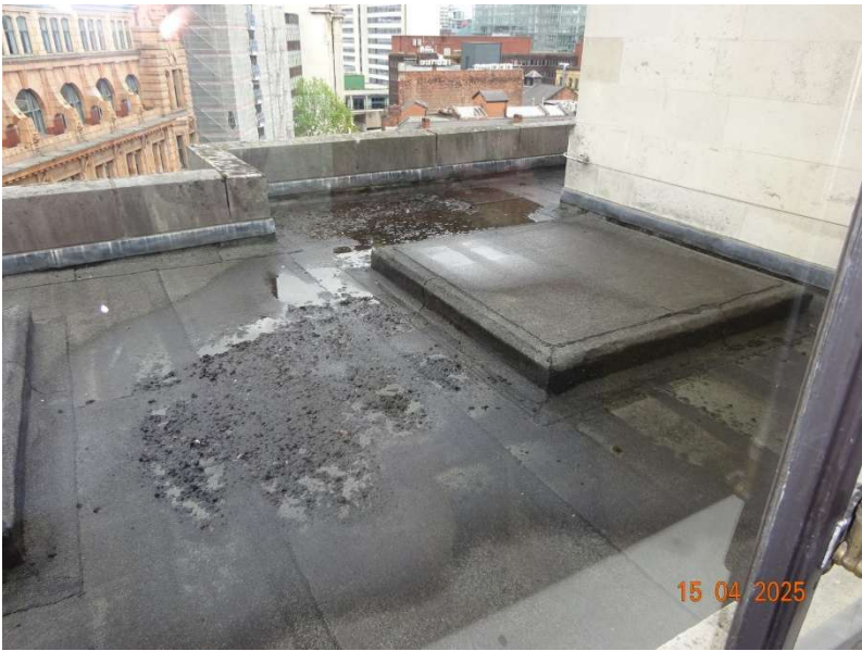
Photograph 16 5 th floor roof (looking north)
