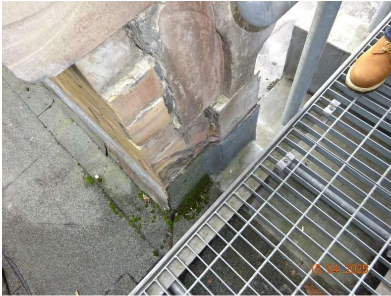
Photograph 10 Flashing to east elevation parapet
