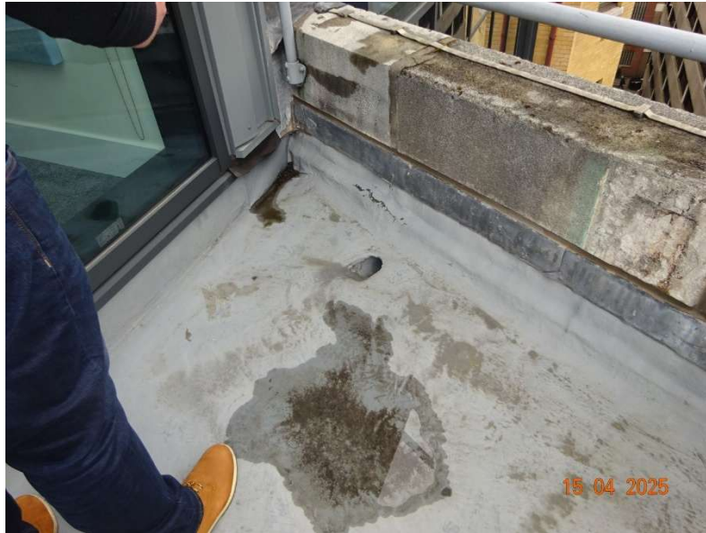
Photograph 18 6 th floor roof parapet (looking east)
