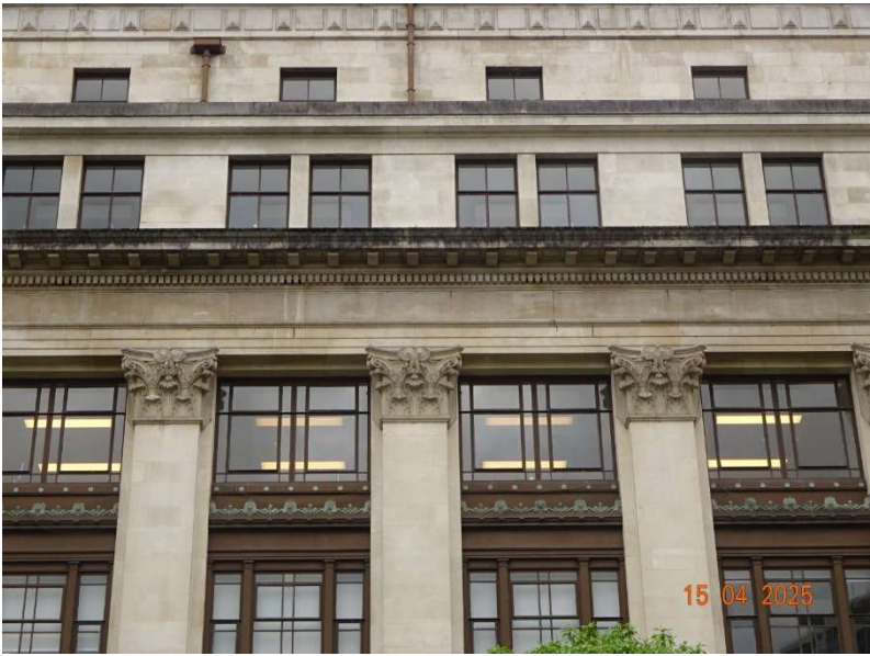
Photograph 23 View of north elevation (5 th floor ledge and roof)
