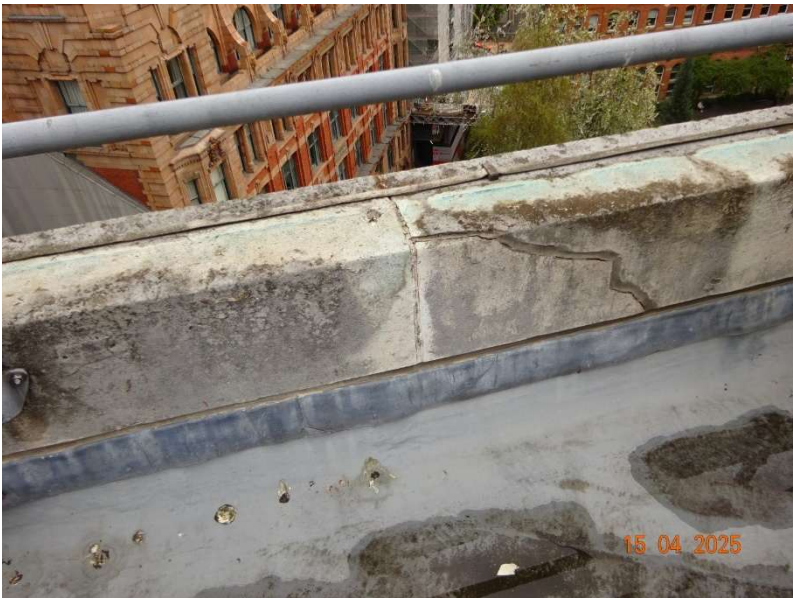
Photograph 20 6 th floor roof parapet (looking north)
