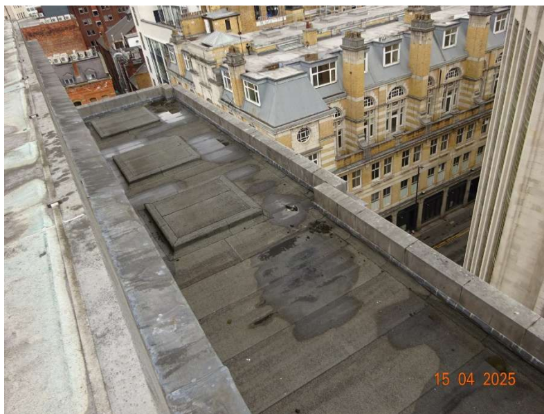
Photograph 6 5 th floor roof (looking east)
