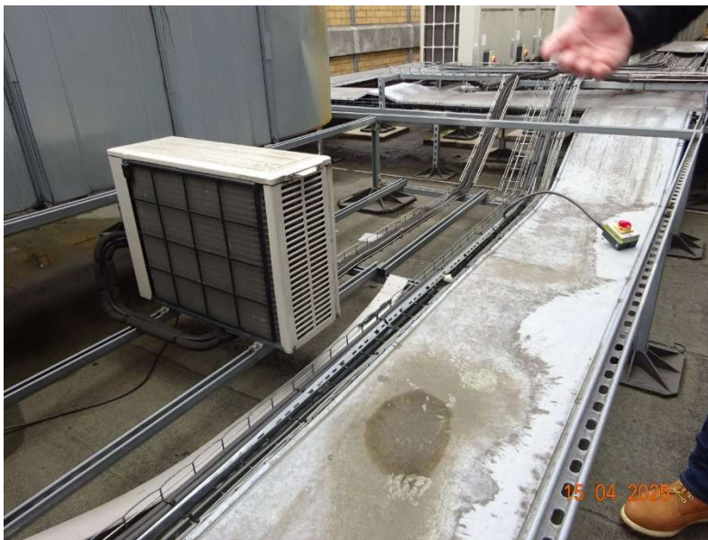
Photograph 13 View of roof mounted plant (6 th floor roof)
