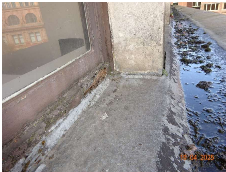
Photograph 4 North elevation 5 th floor ledge (looking west)
