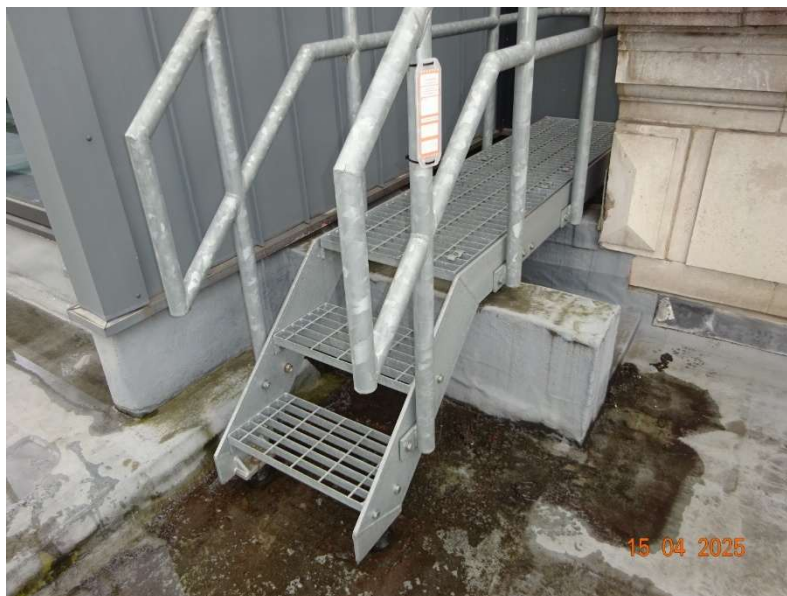
Photograph 9 Roof mounted steps (east elevation)
