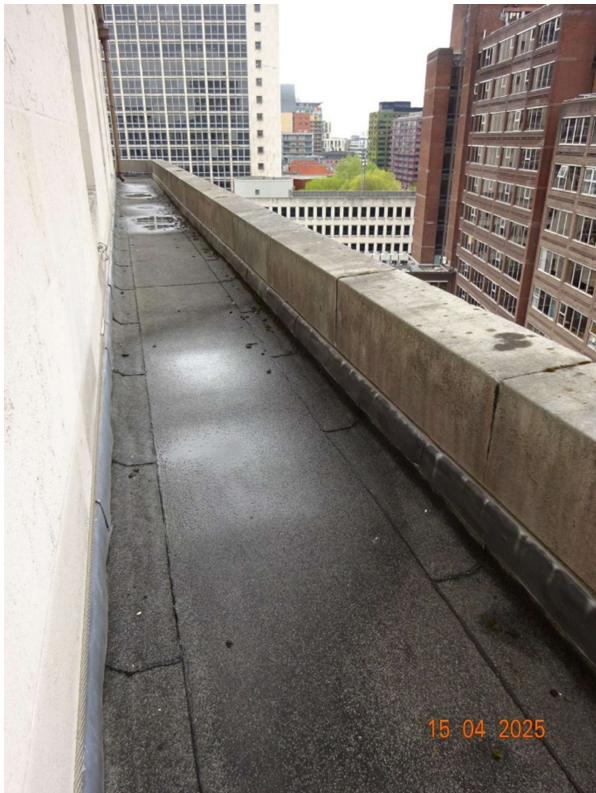
Photograph 17 5 th floor roof (looking west)
