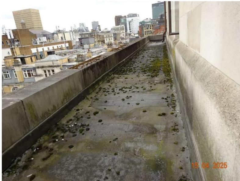
Photograph 14 5 th floor roof (looking east)
