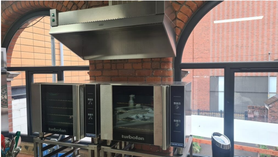
Image 6: Lincat internal air extraction and carbon filter hood situated above 2 x convection ovens in kitchen
