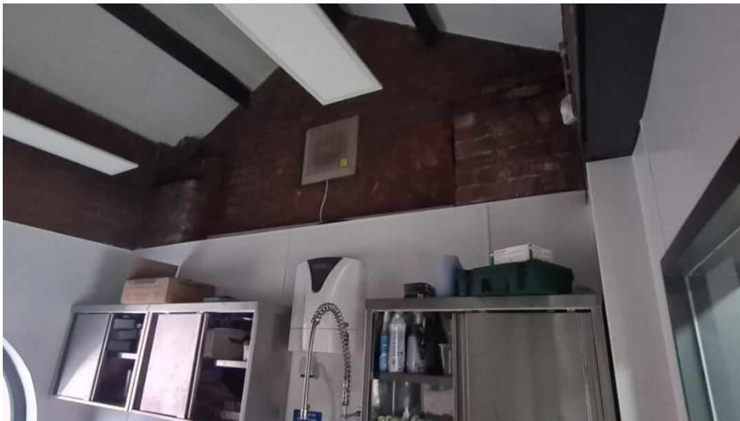
Image 2: Internal fan and vent to the preparation kitchen opposite Fairbairn House
