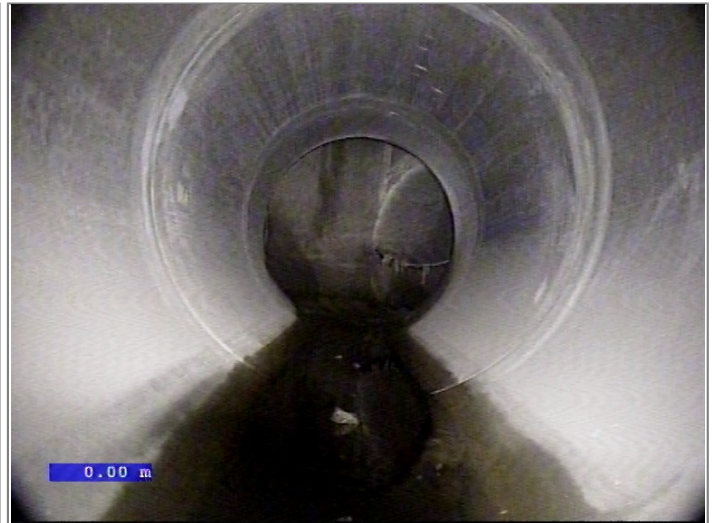
Water level 5% height/diameter
