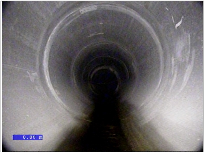
Water level 5% height/diameter
