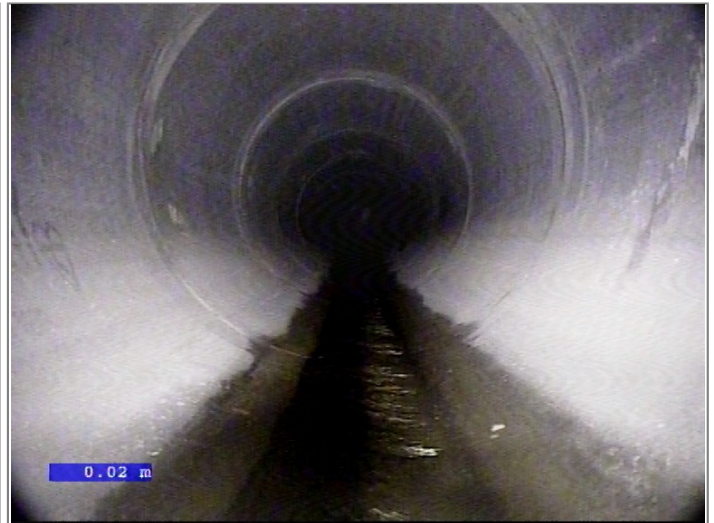
Water level 5% height/diameter
