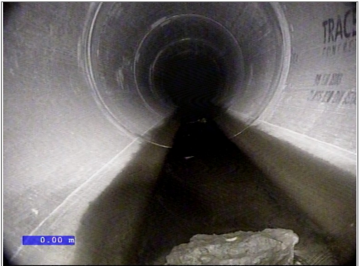
Water level 5% height/diameter
