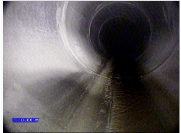
Water level 5% height/diameter
