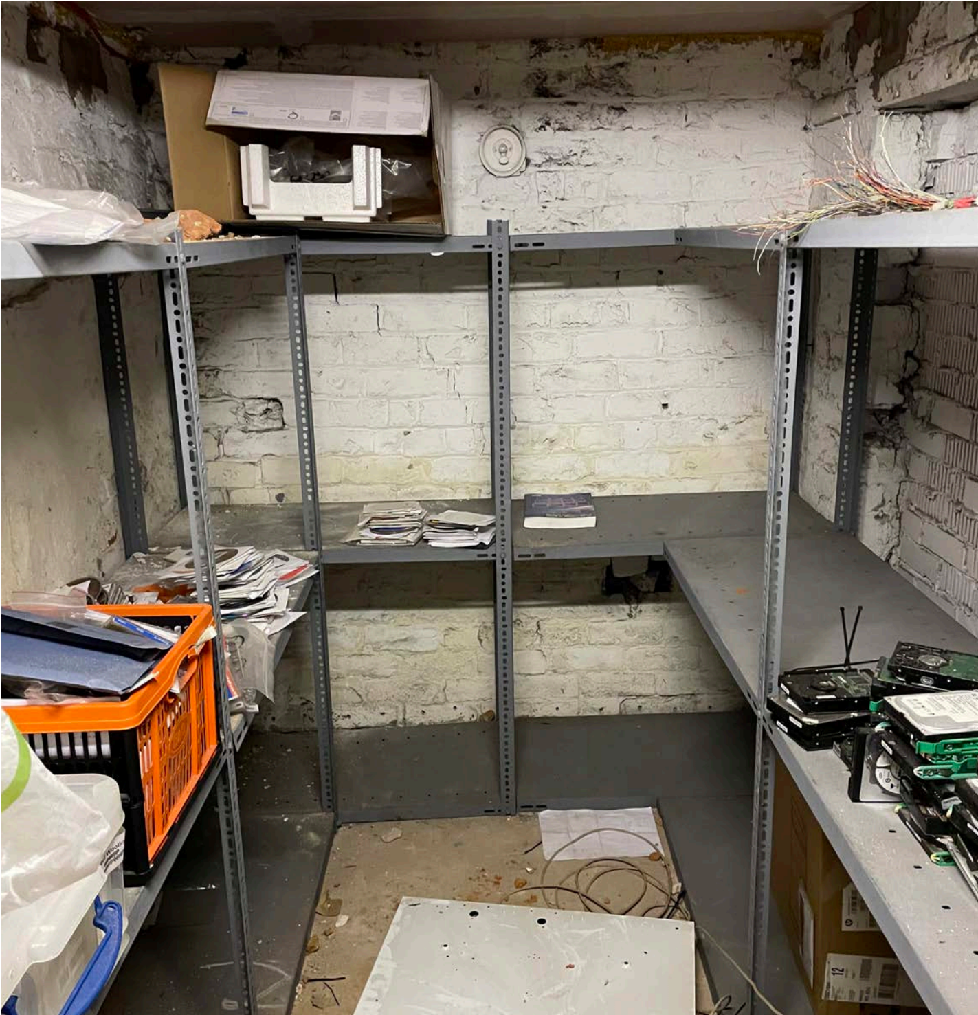
Store - Existing door and internal wall Dem.03 / 06
