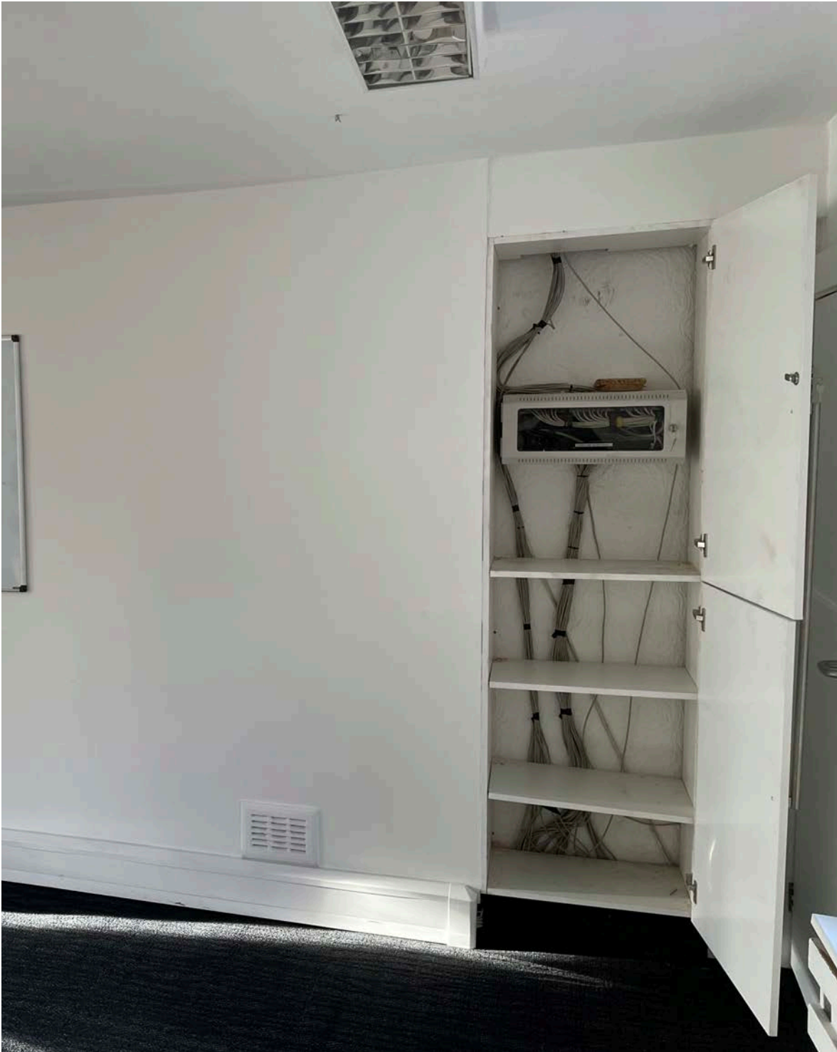
Office - Existing outrigger store and internal plasterboard lining / cupboard Dem.42 / 43 / 46
