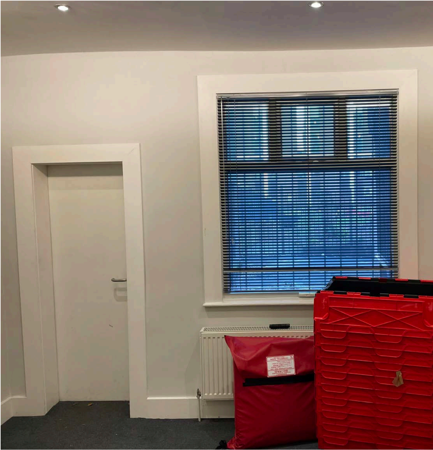
Meeting Room - Existing outriggers and boiler door Dem.15
