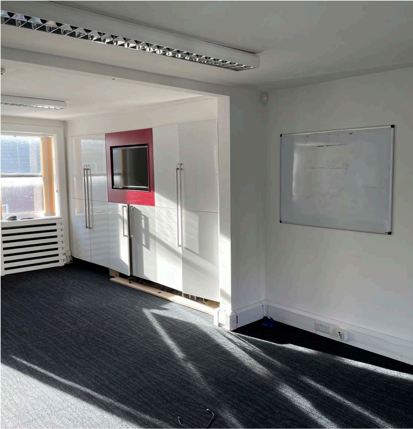
Office - Existing opening, internal wall linings / cupboards and false ceiling Dem.45 / 46 / 52
