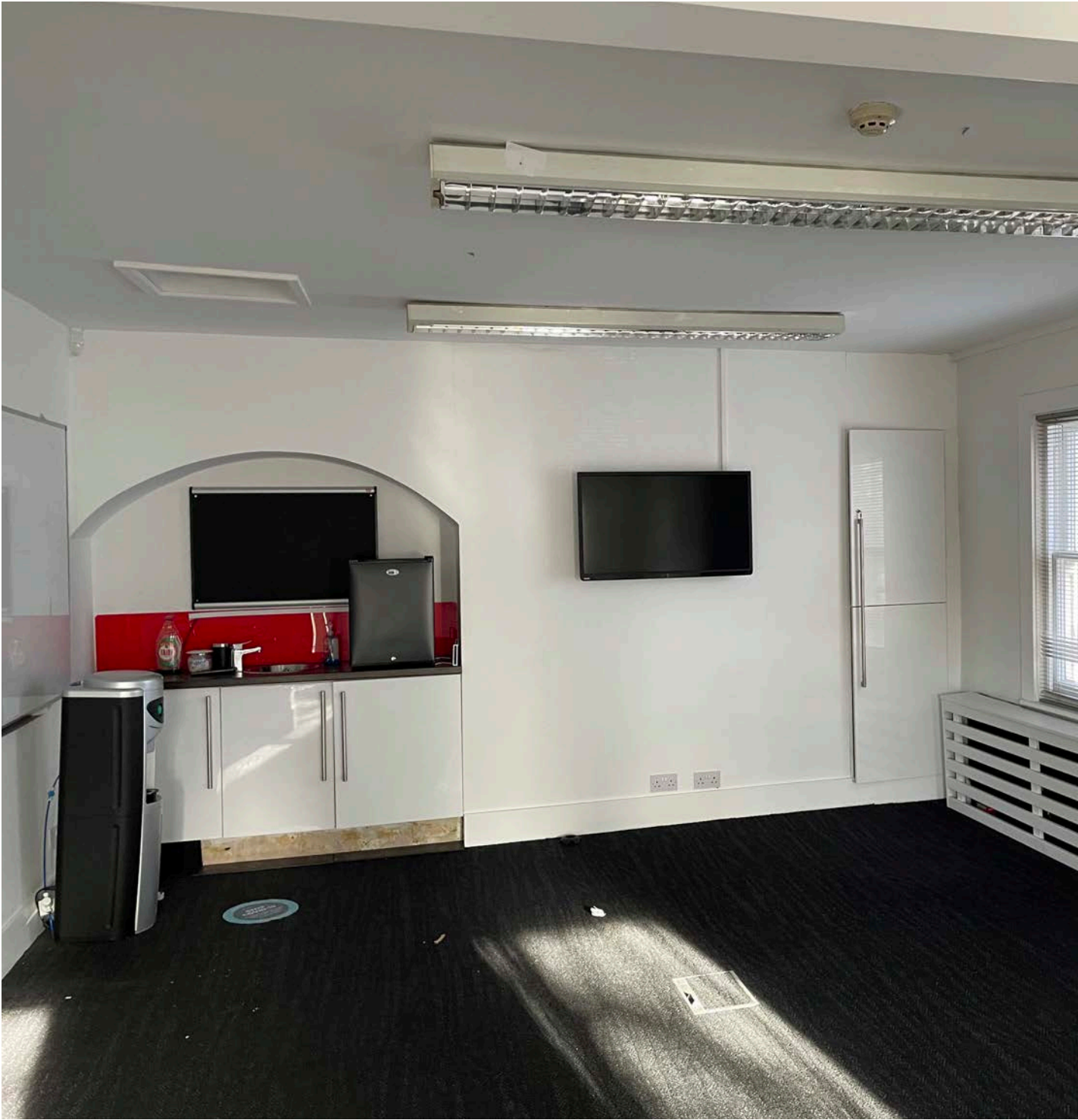
Office - Internal wall linings / cupboards, raised access floor, false ceiling and sanitary ware Dem.46 / 47 / 50 / 51 / 52 / 53
