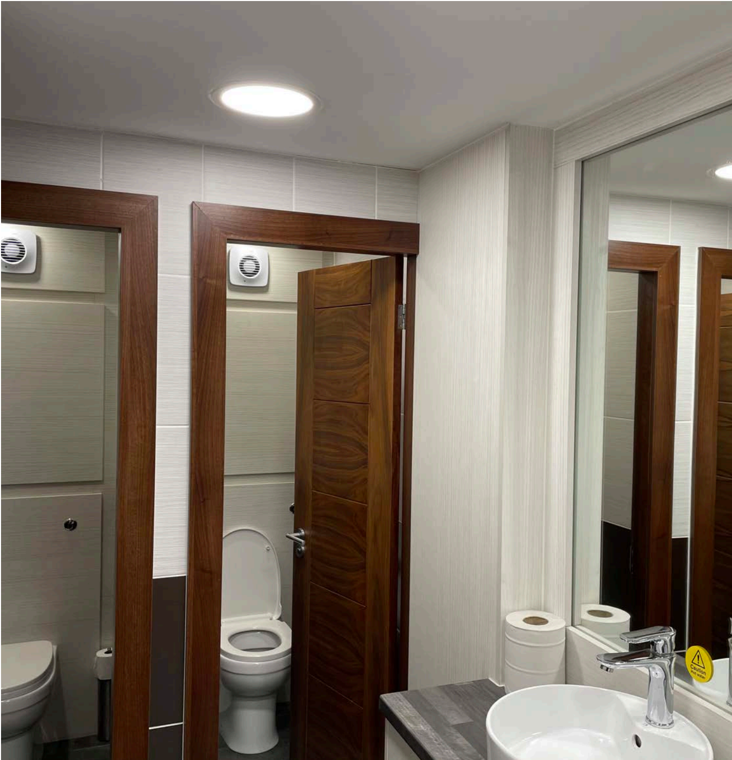
WC - Existing outrigger, WC and fixtures Dem.28 / 33
