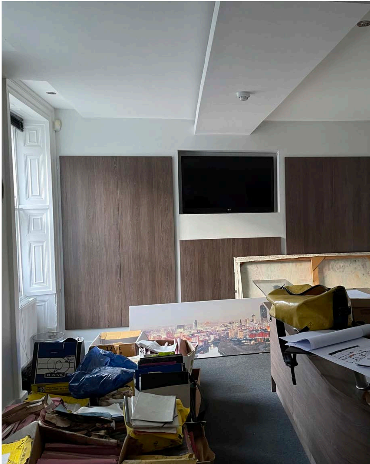
Reception - Modern internal wall linings Dem.17
