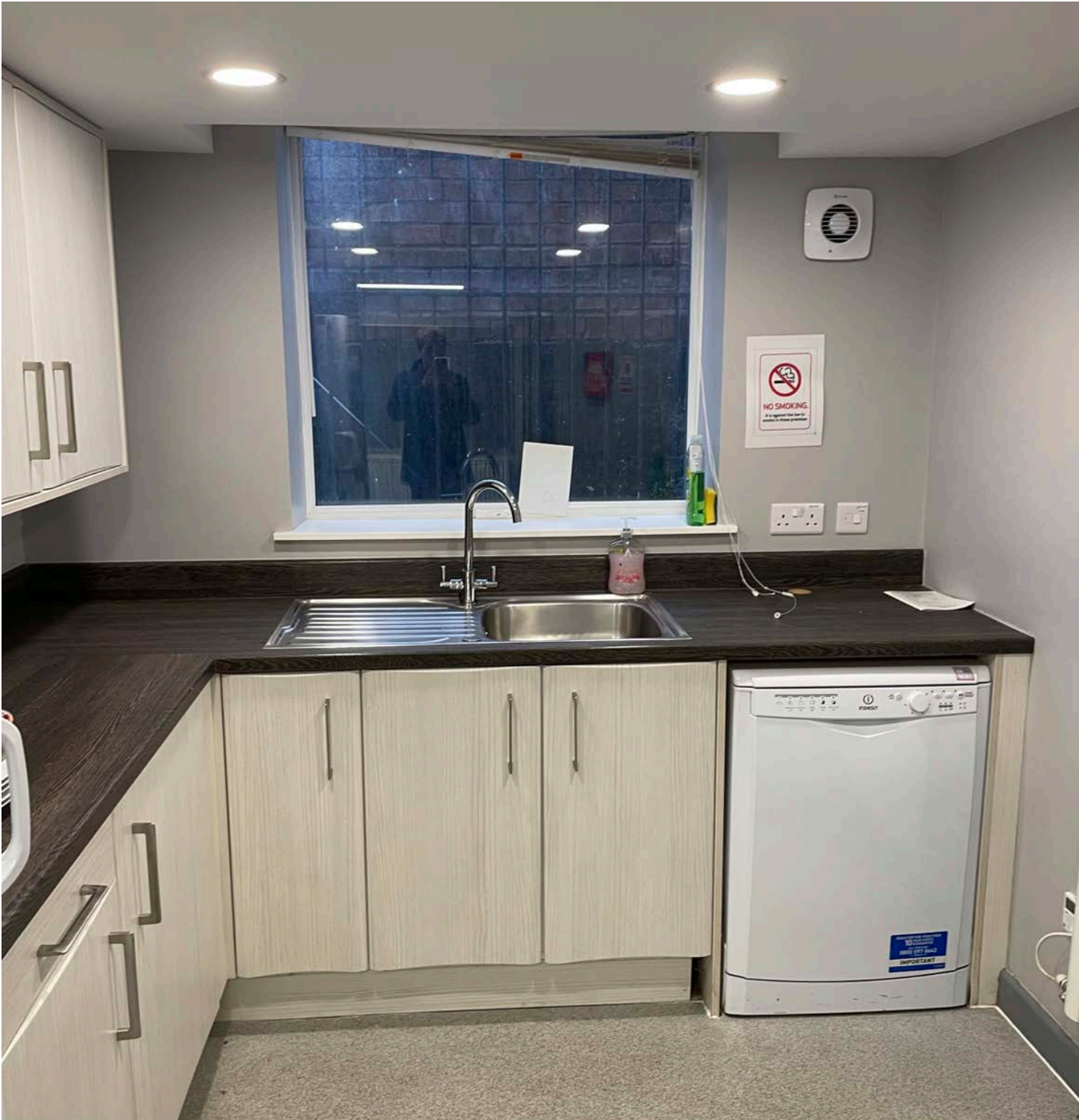
Kitchen - Sanitary ware and fixtures Dem.11 / 14
