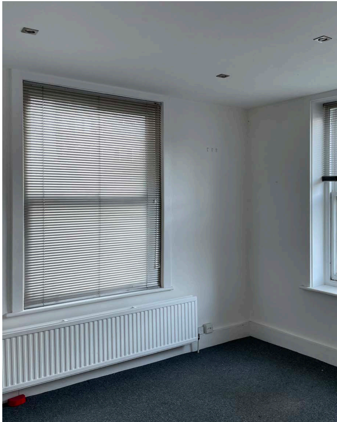
Office - Modern internal wall linings / boxing out, false ceiling and raised access flooring Dem.31 / 38 / 40
