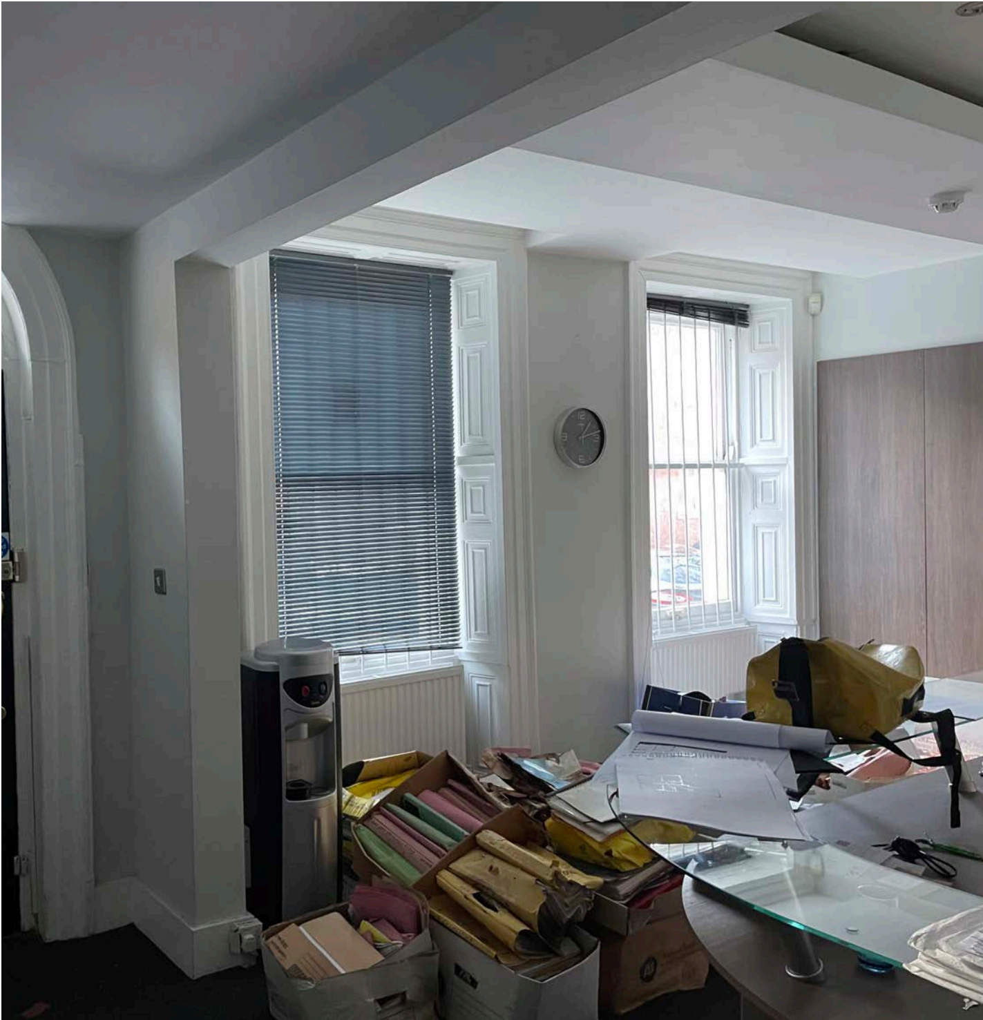
Reception - Existing wall opening and false ceiling Dem.17 / 19 / 26
