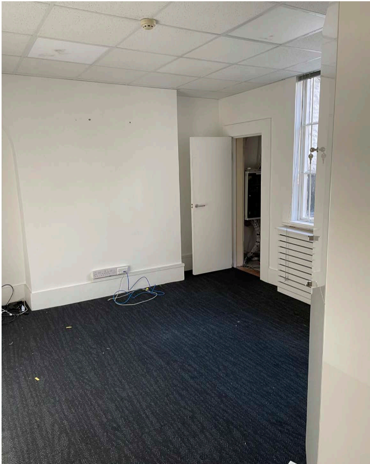
Office - Existing window / outrigger, false ceiling and modern internal wall linings Dem.29 / 31 / 32 / 40
