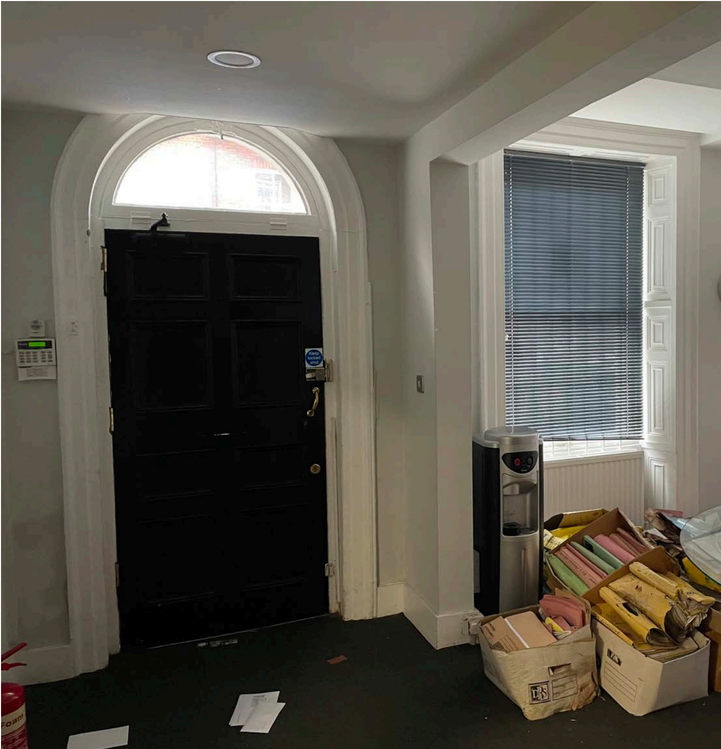
Hallway - Existing door / wall openings and false ceiling Dem.19 / 26
