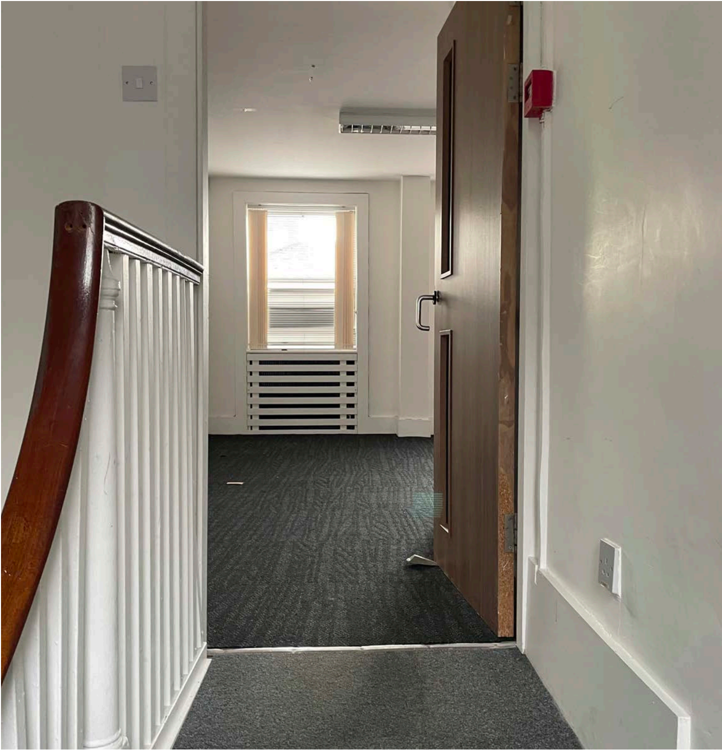
Hallway - Existing landing and false ceiling Dem.48 / 52
