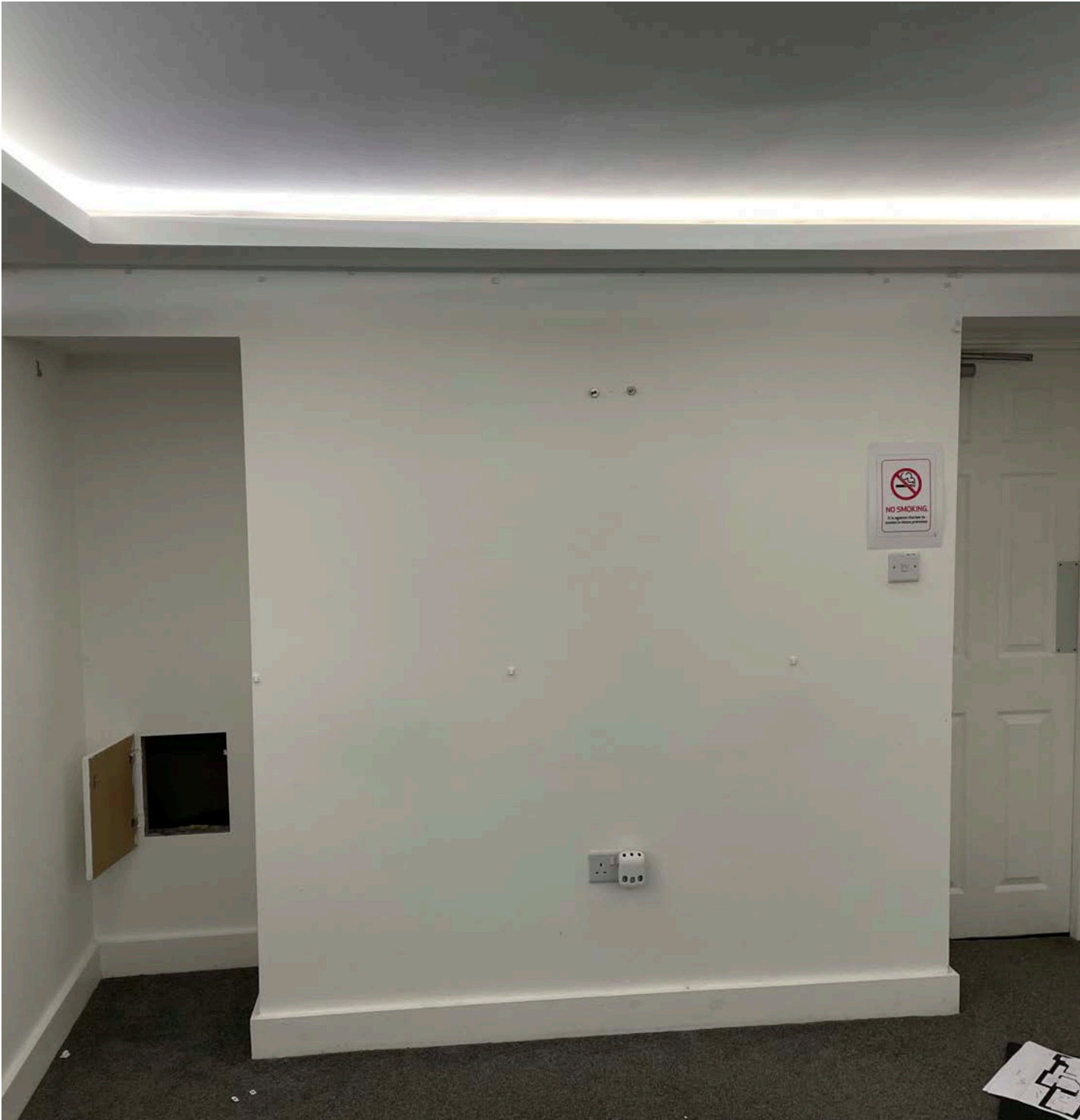
Office - Existing wall and door Dem.08
