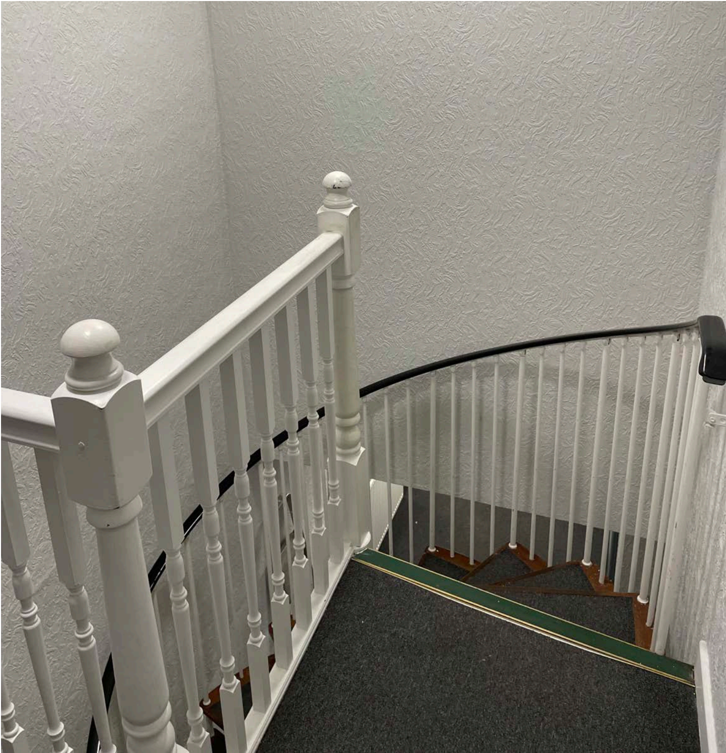
Landing - Existing spiral stair and raised access floor Dem.21 / 25
