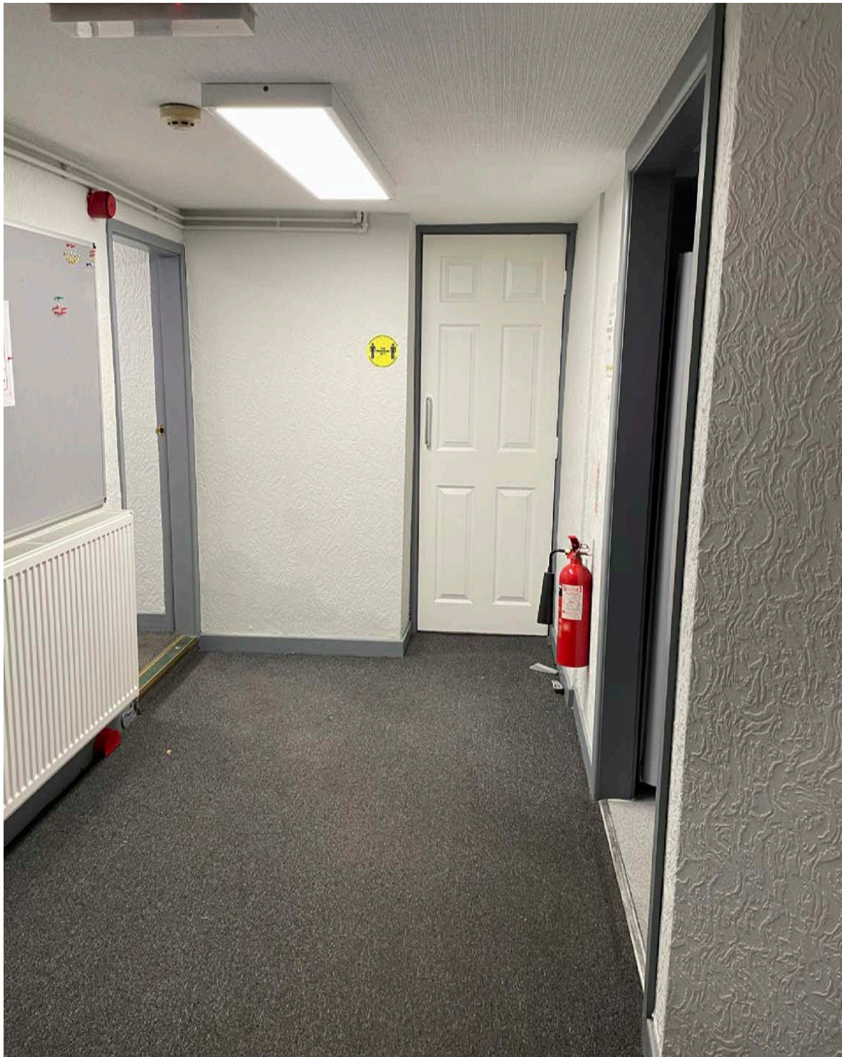
Corridor - Existing corridor door, internal partitions and false ceiling Dem.03 / 08 / 14
