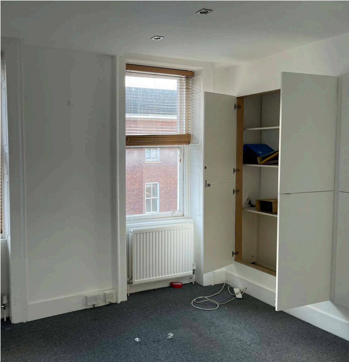
Office - Modern internal wall linings / cupboards and false ceiling Dem.31 / 40
