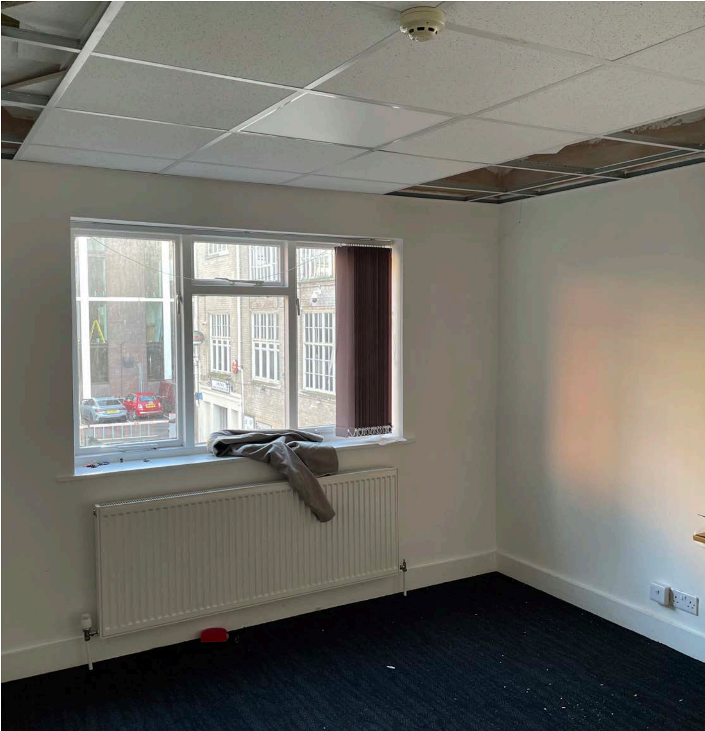
Office - Existing north elevation outrigger and false ceiling Dem.37 / 39 / 40
