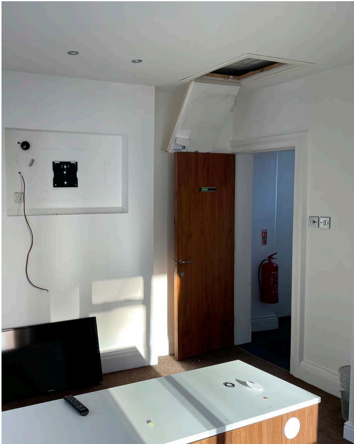
Office - Existing office door, false ceiling and plasterboard wall linings Dem.46 / 47 / 52
