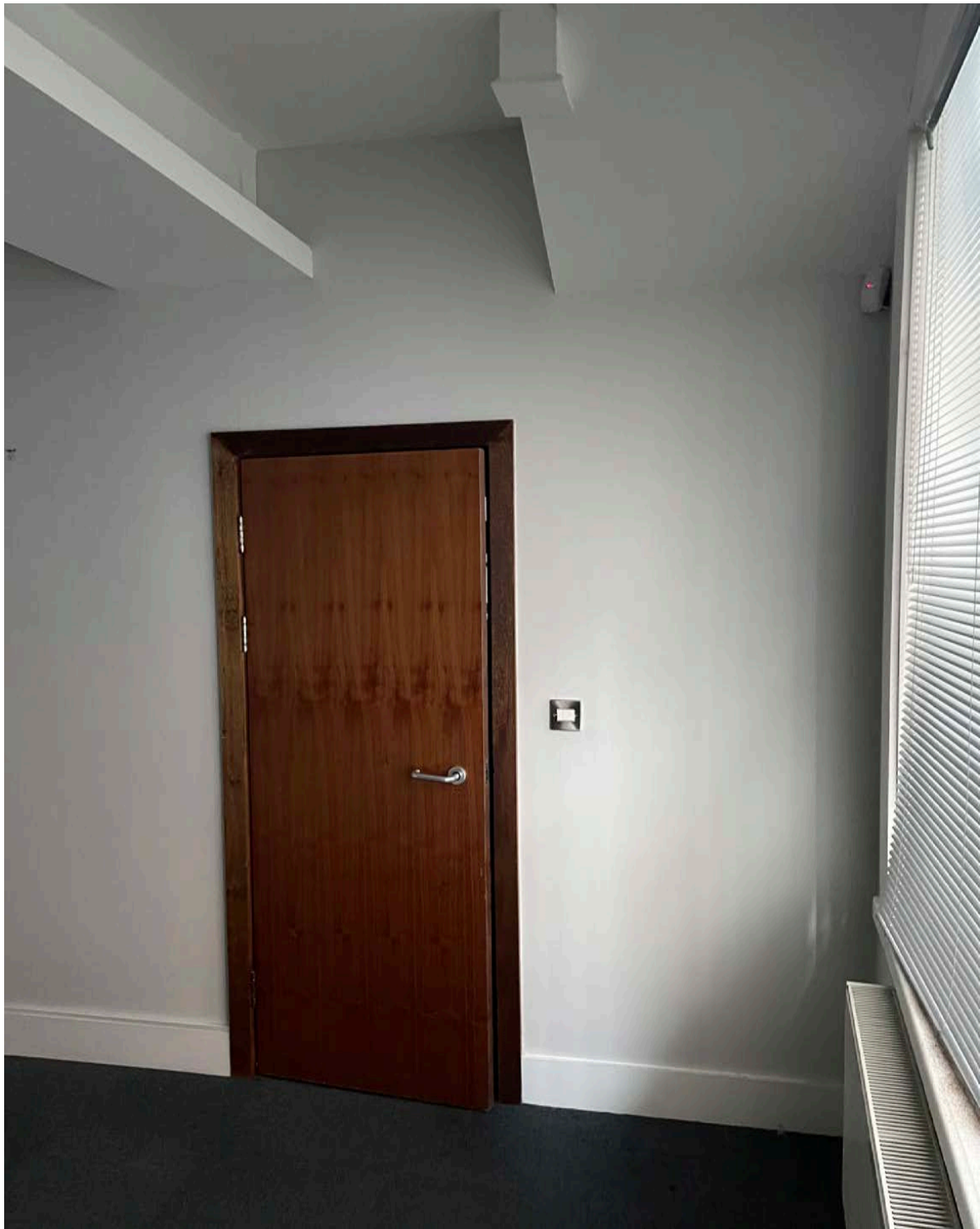
Meeting Room - Existing wall linings and corridor door Dem.15 / 16
