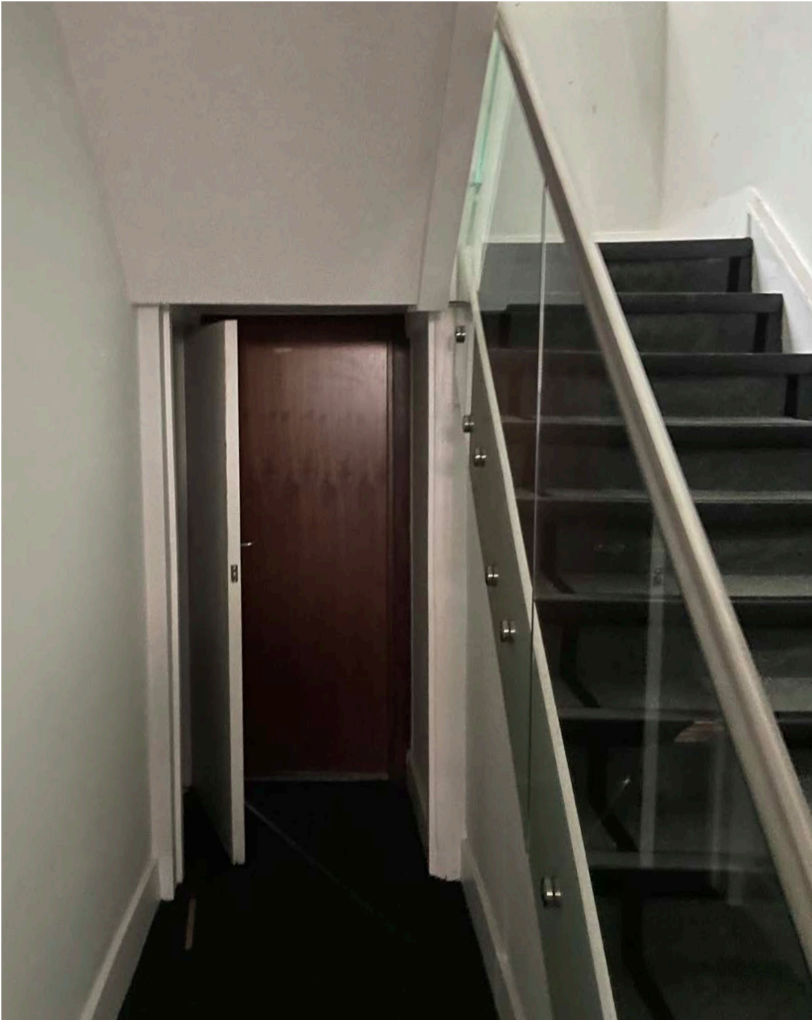
Hallway - Modern glazed balustrade and existing door / wall openings Dem.18 / 19
