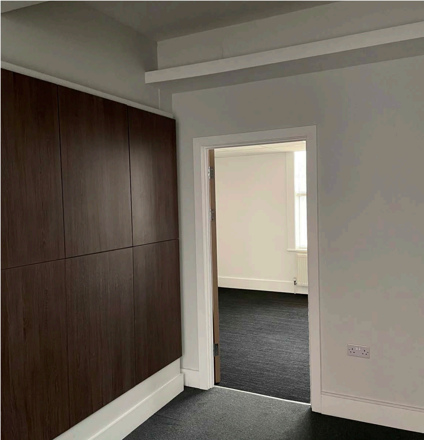
Meeting Room - Existing wall linings and office door Dem.15
