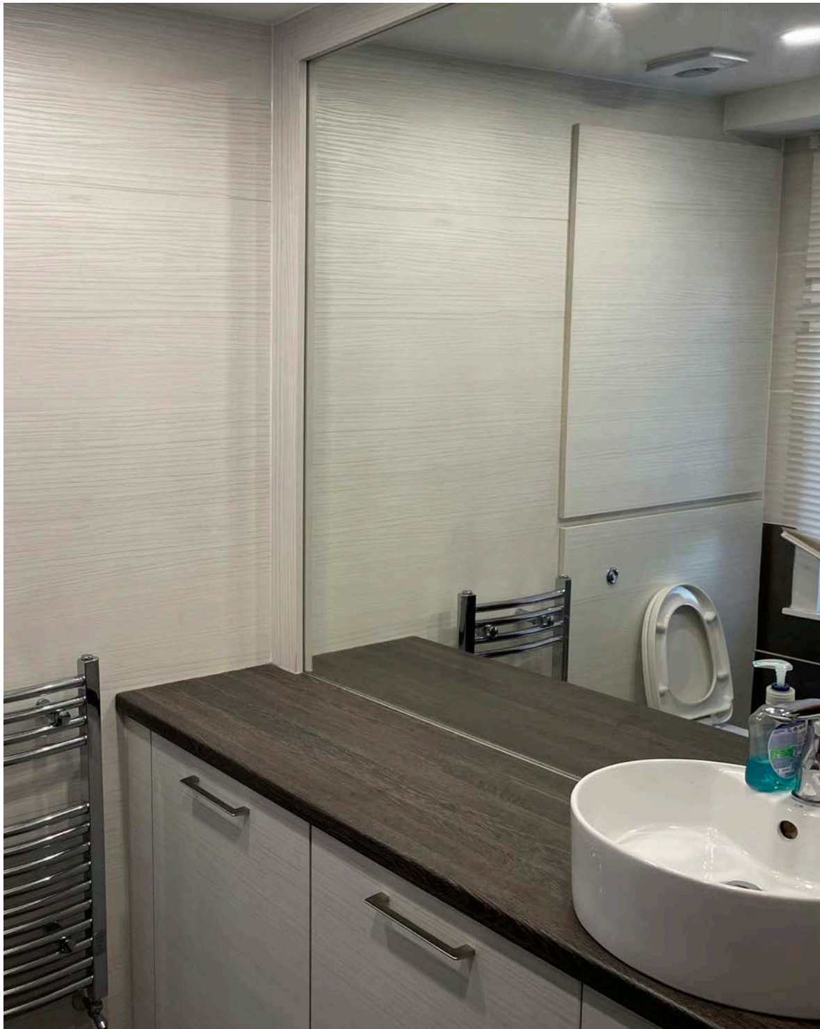
WC - Existing outrigger, WC and fixtures Dem.28 / 33
