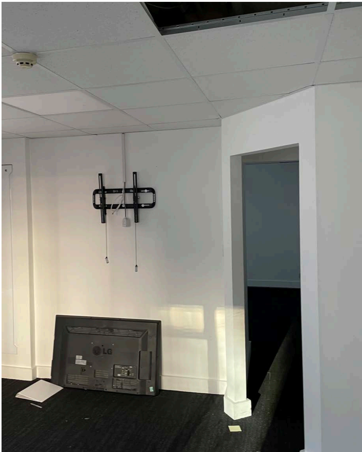
Office - Modern internal wall linings, false ceiling and boxing out Dem.31 / 39 / 40
