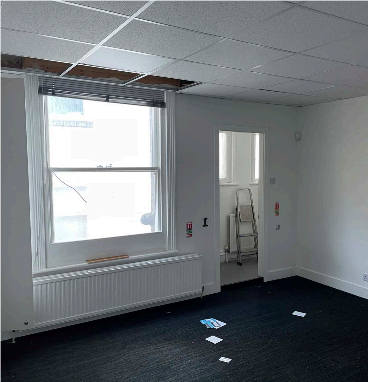
Office - Modern internal wall linings / boxing out, door into store, false ceiling and raised access flooring Dem.31 / 32 / 38 / 40
