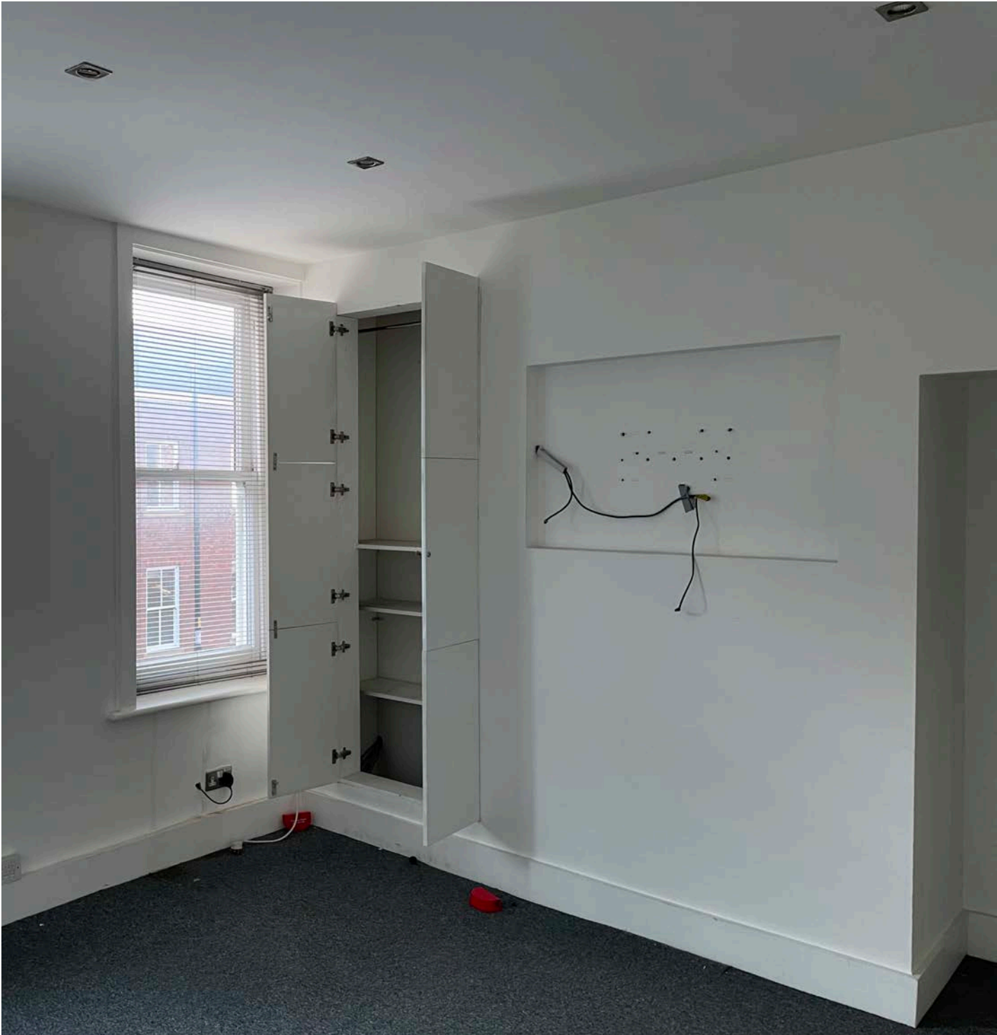
Office - Modern internal wall linings / boxing out, false ceiling and raised access flooring Dem.31 / 38 / 40
