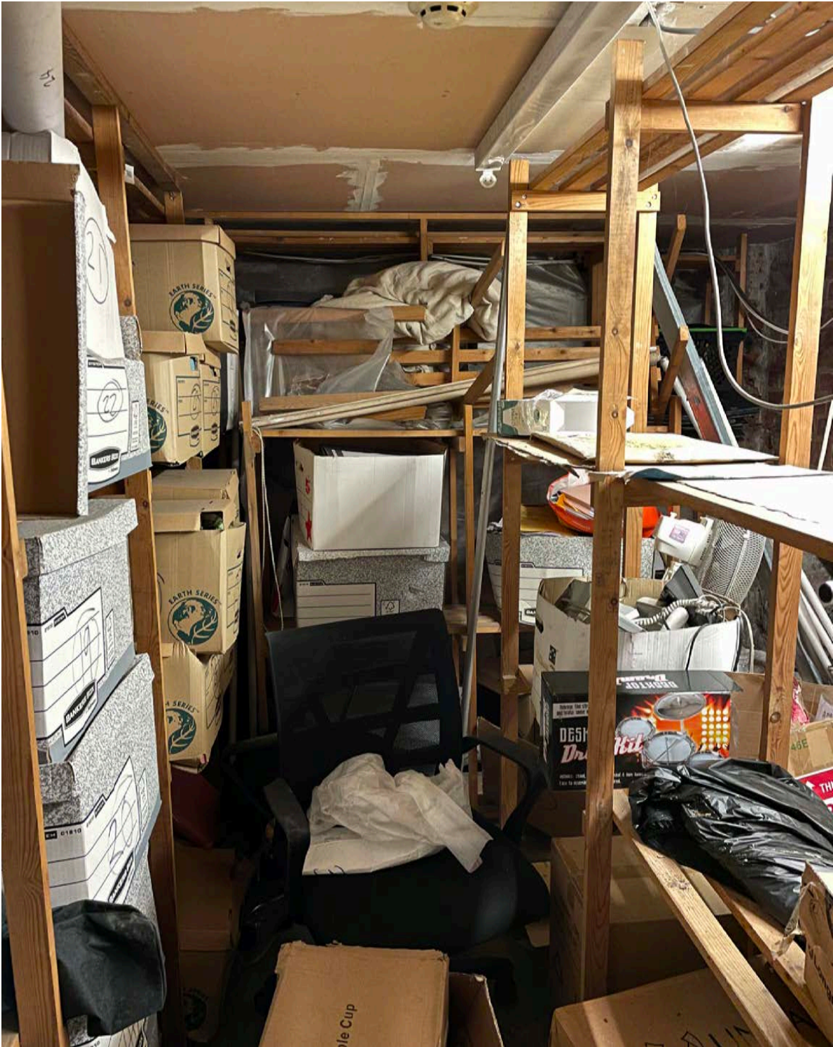
Store - Existing wall return and stair Dem.04 / 05
