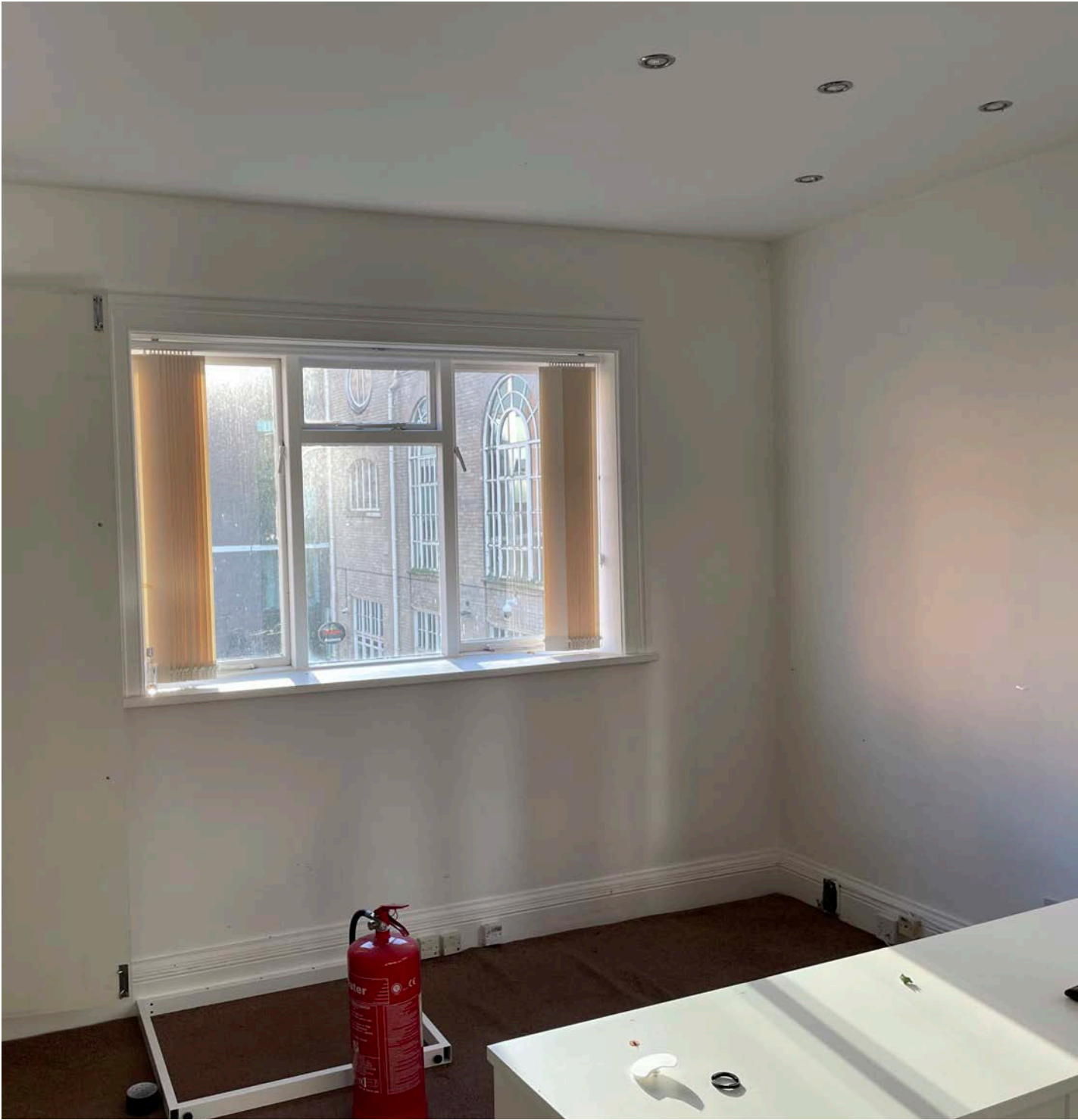
Office - North elevation outrigger window and false ceiling Dem.49 / 52
