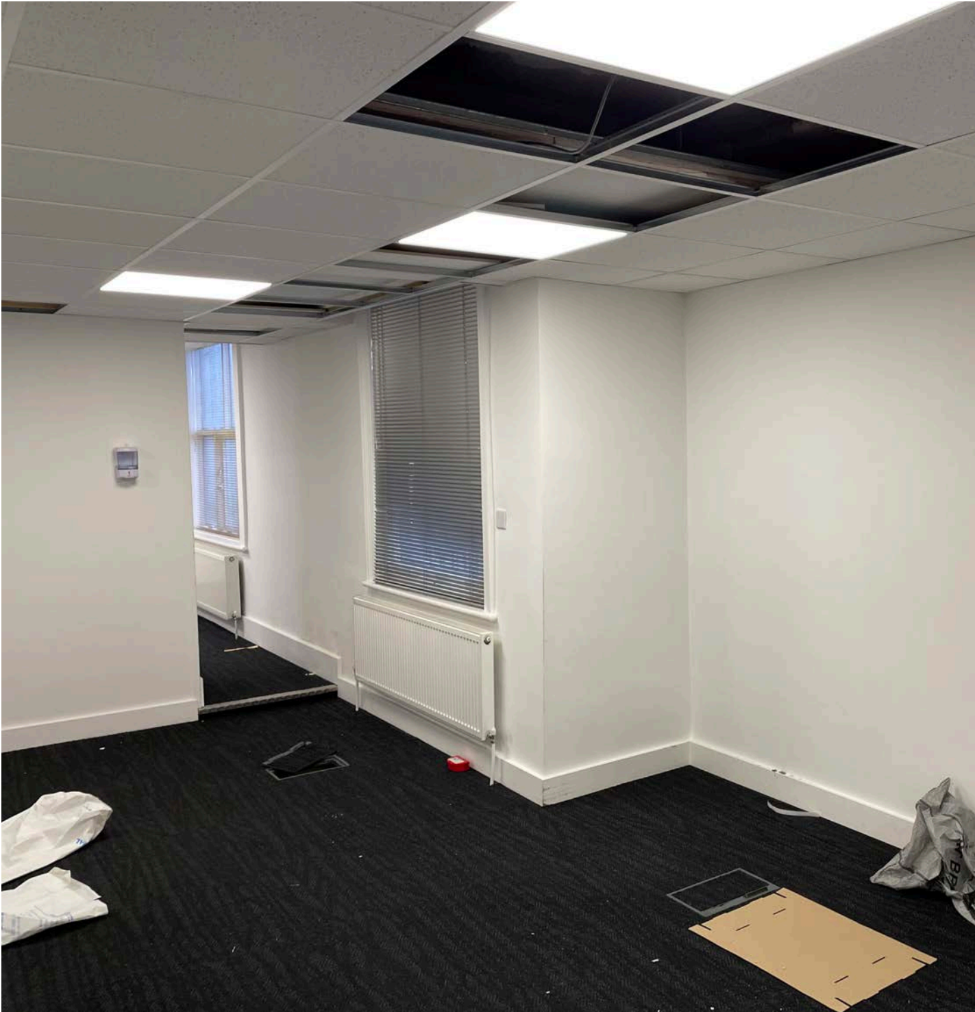
Office - Modern internal wall linings and boxing out Dem.17
