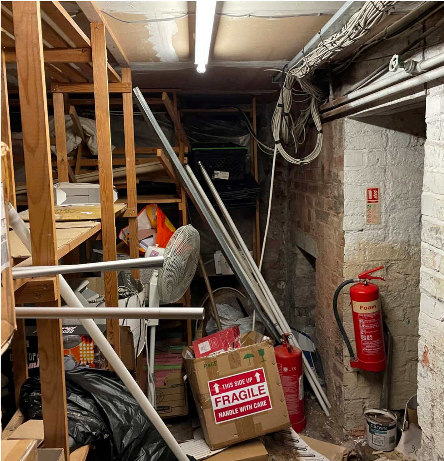
Store - Existing wall Return Dem.04 / 05
