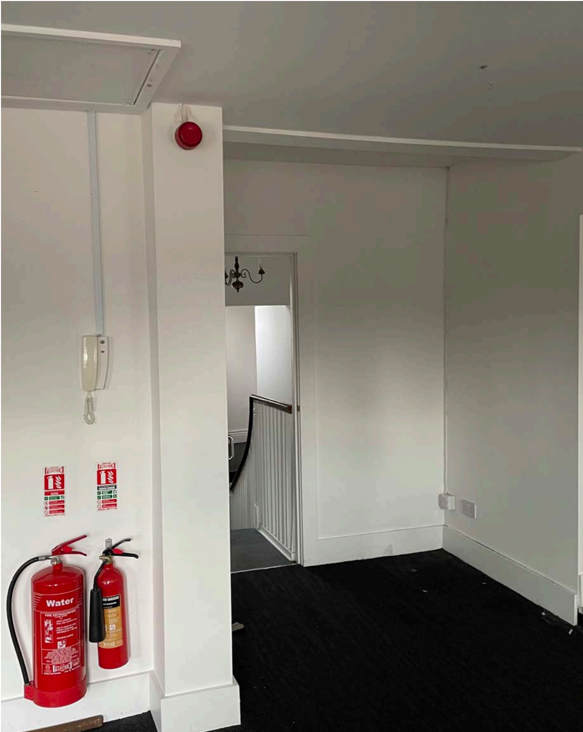
Hallway - Existing landing, false ceiling and fitted furniture Dem.48 / 52 / 53
