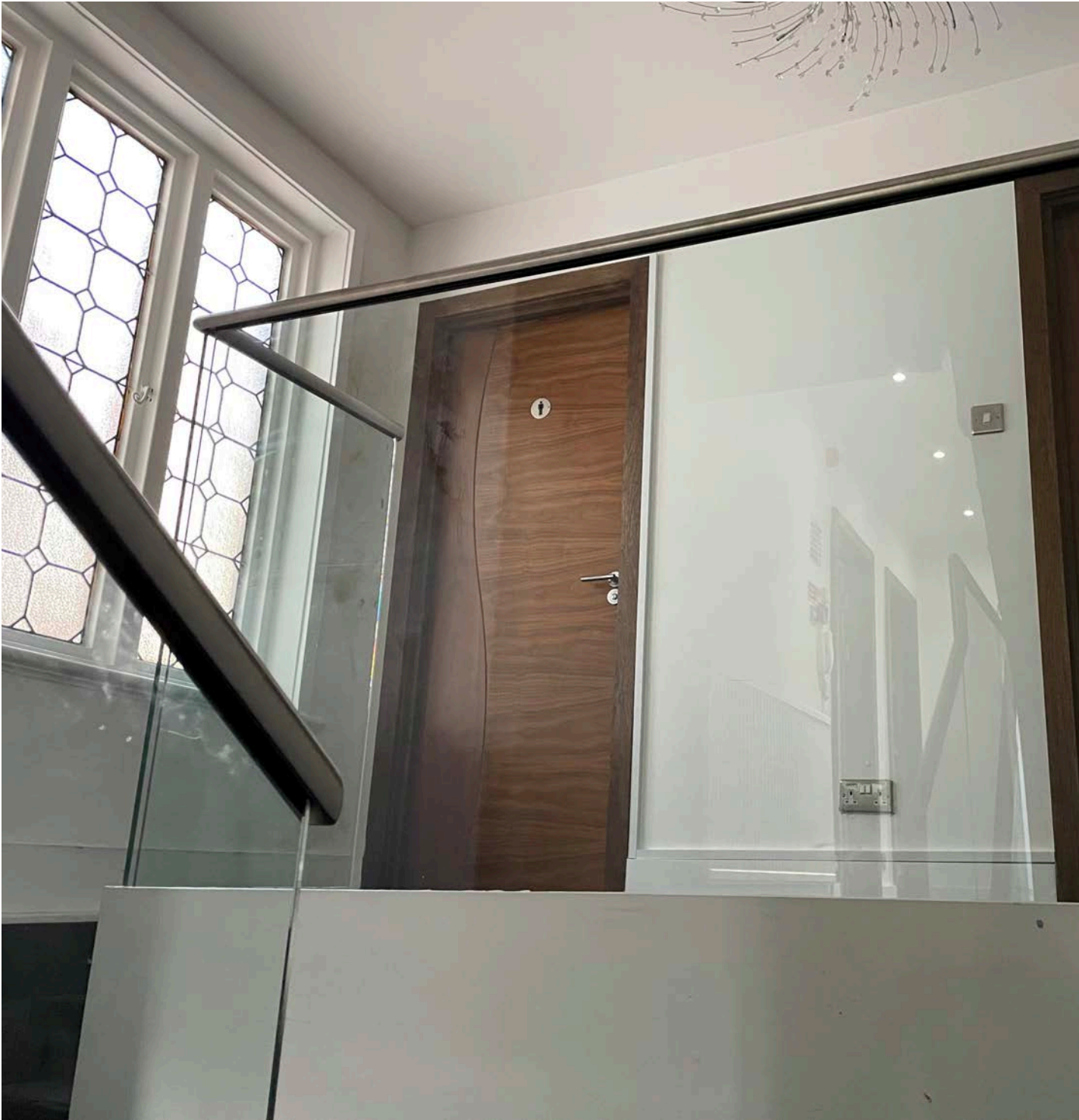
Landing - Existing glazed balustrade / risers, false ceiling and modern internal wall linings / boxing out Dem.30 / 31 / 40
