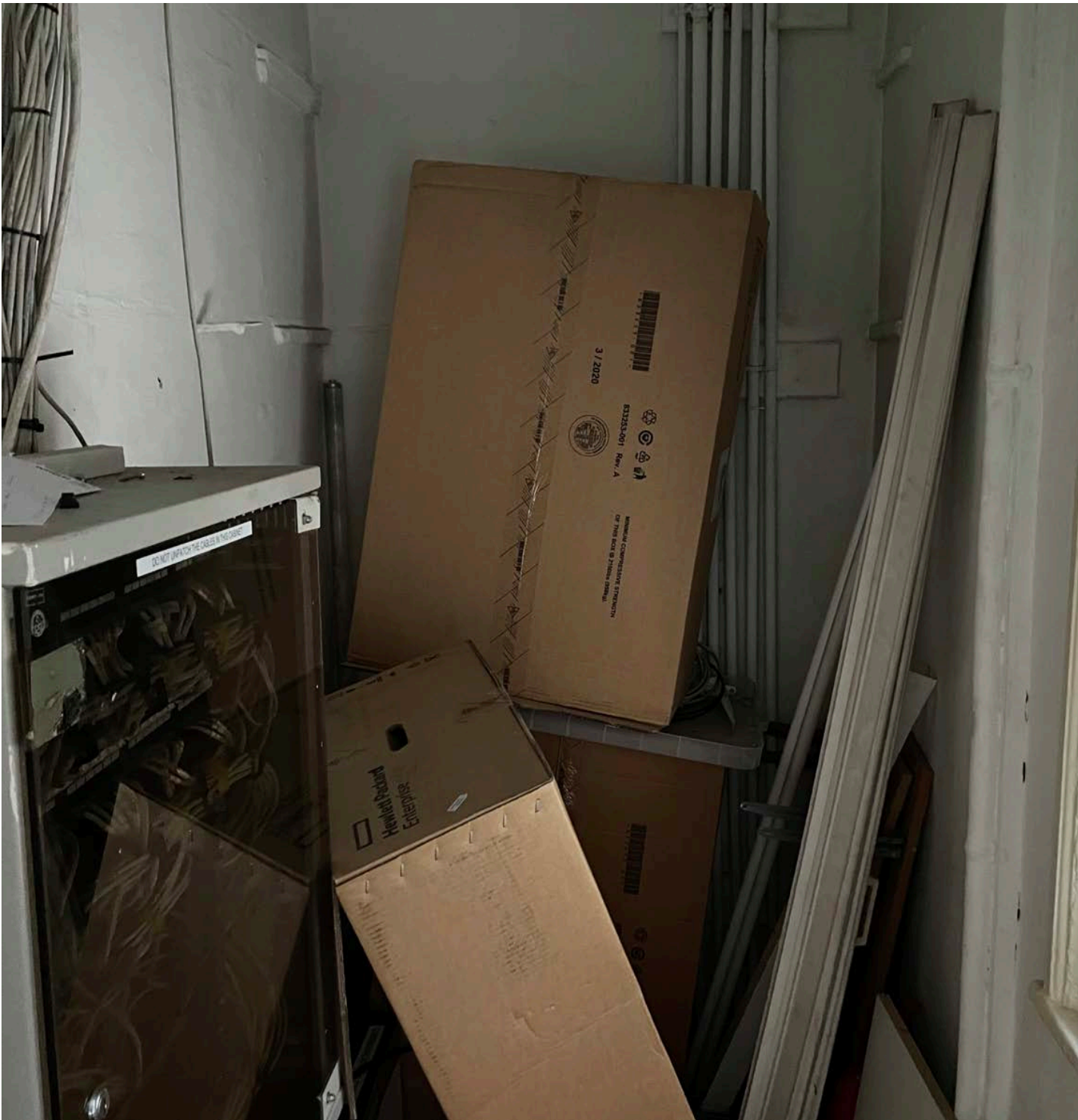
Cupboard - Existing outrigger cupboard Dem.28
