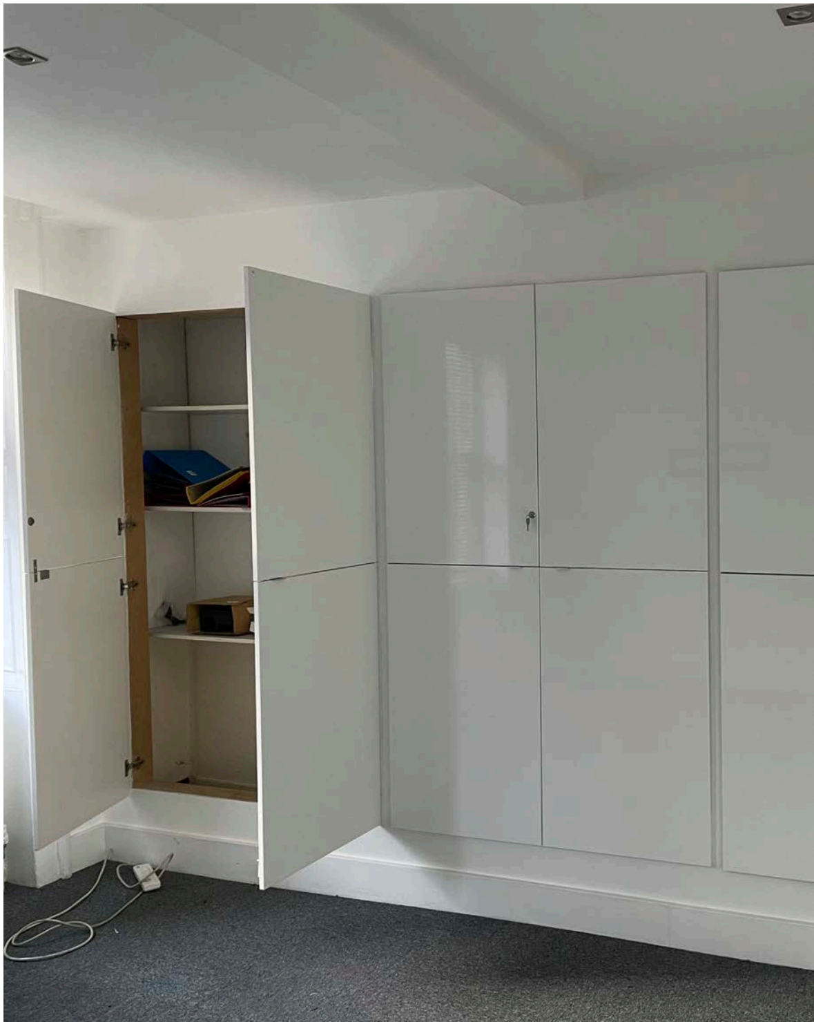
Office - Modern internal wall linings / cupboards and false ceiling Dem.31 / 40
