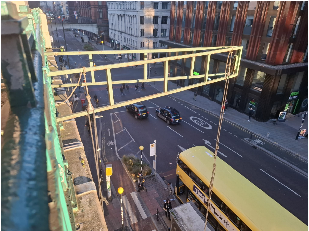
VIEW OF EXISTING BANNER GANTRY AND OXFORD ROAD
