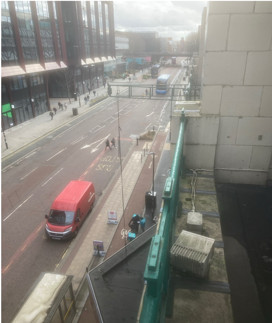
VIEW OF EXISTING BANNER GANTRY AND ENTRANCE CANOPY ROOF
