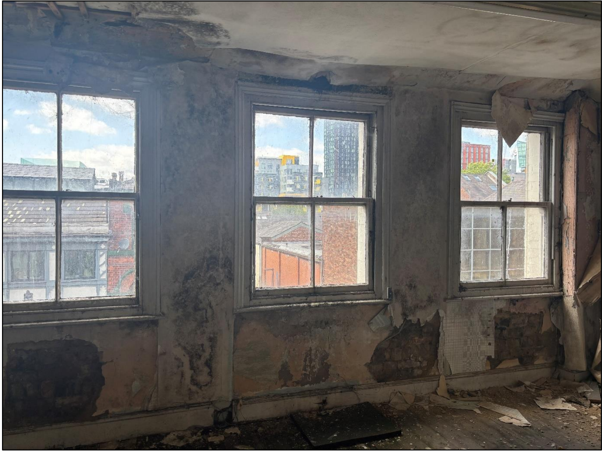
Figure 25: The windows on the second floor of No.68, facing north
