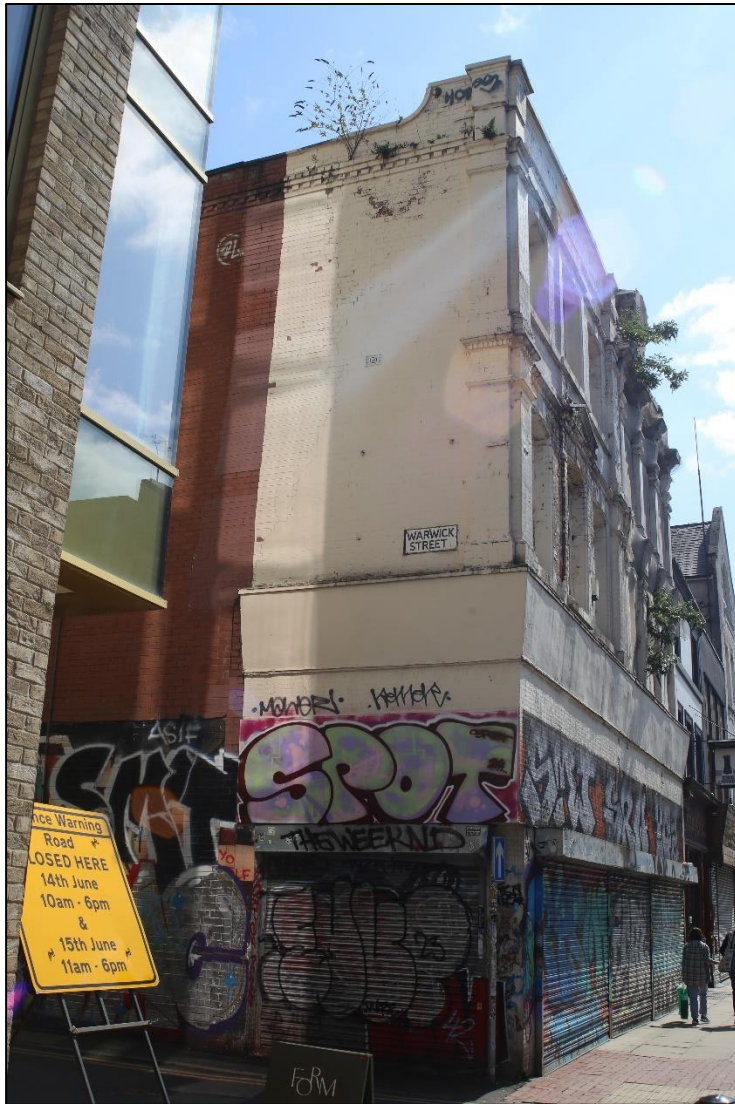
Figure 17: General view of the north-east façade of No.70, facing south-west
