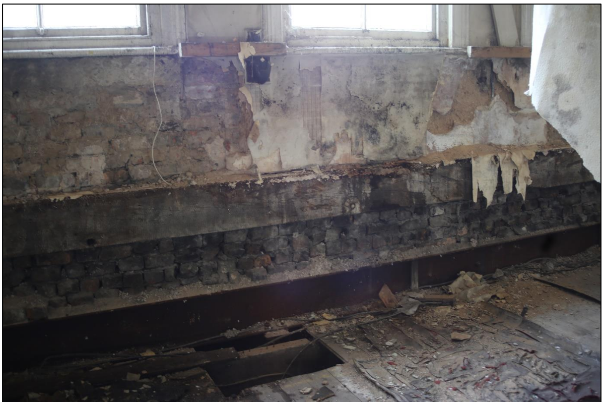
Figure 24: ]The timber beam within the façade of No.70, facing north
