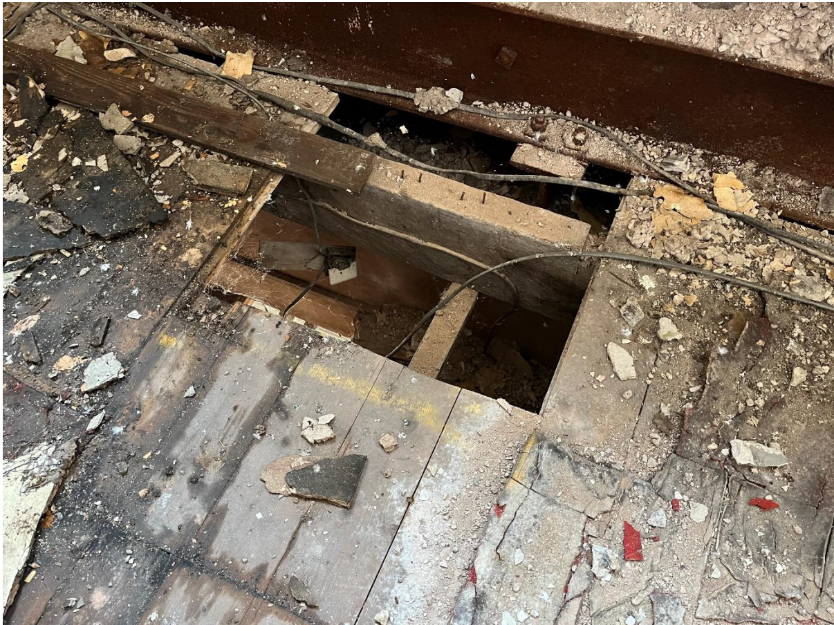
Figure 7: No.70 First Floor joist
