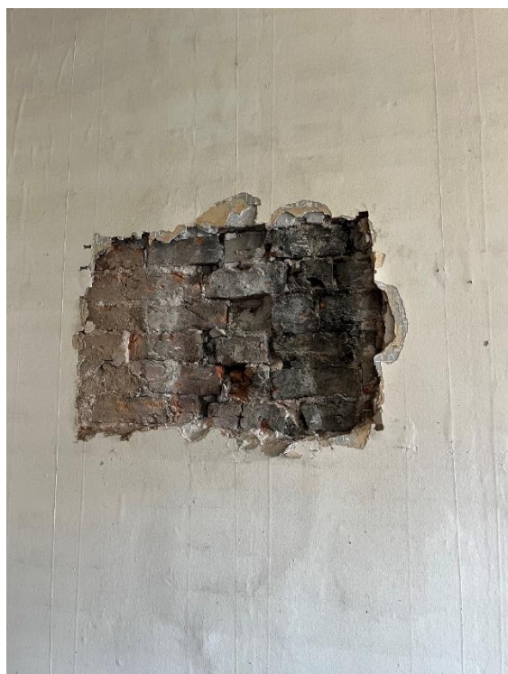
Figure 10: First Floor level - Party wall with No.68 and Castle Hotel
