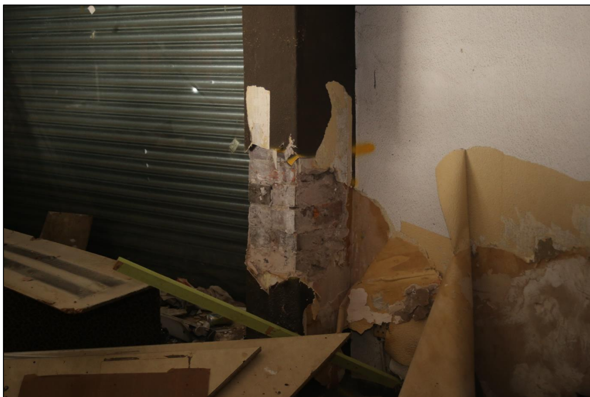
Figure 21: Detail of the brick pier situated within the north-east wall of No.70, facing north
