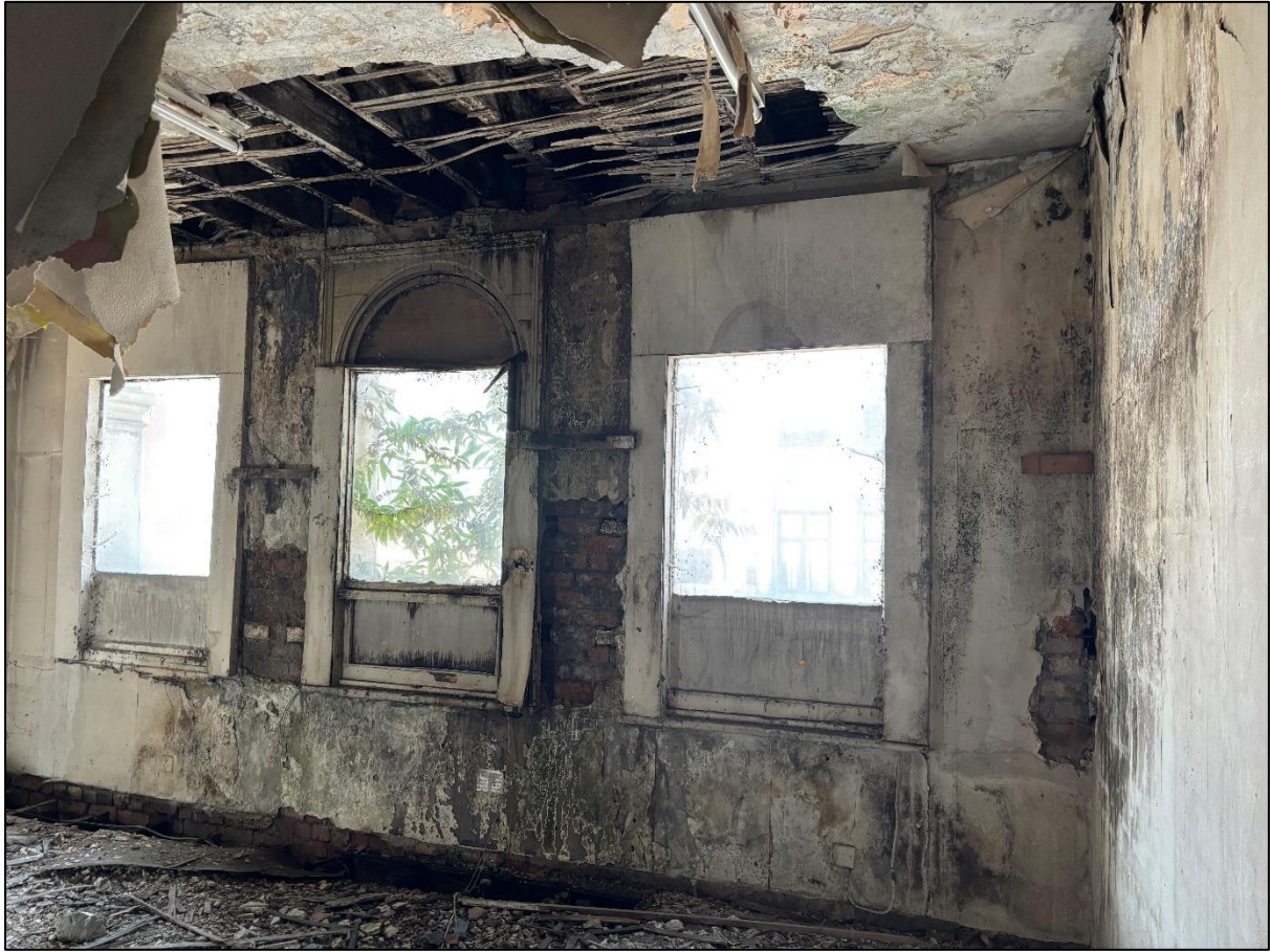
Figure 22: The windows on the first floor of No.68, facing west
