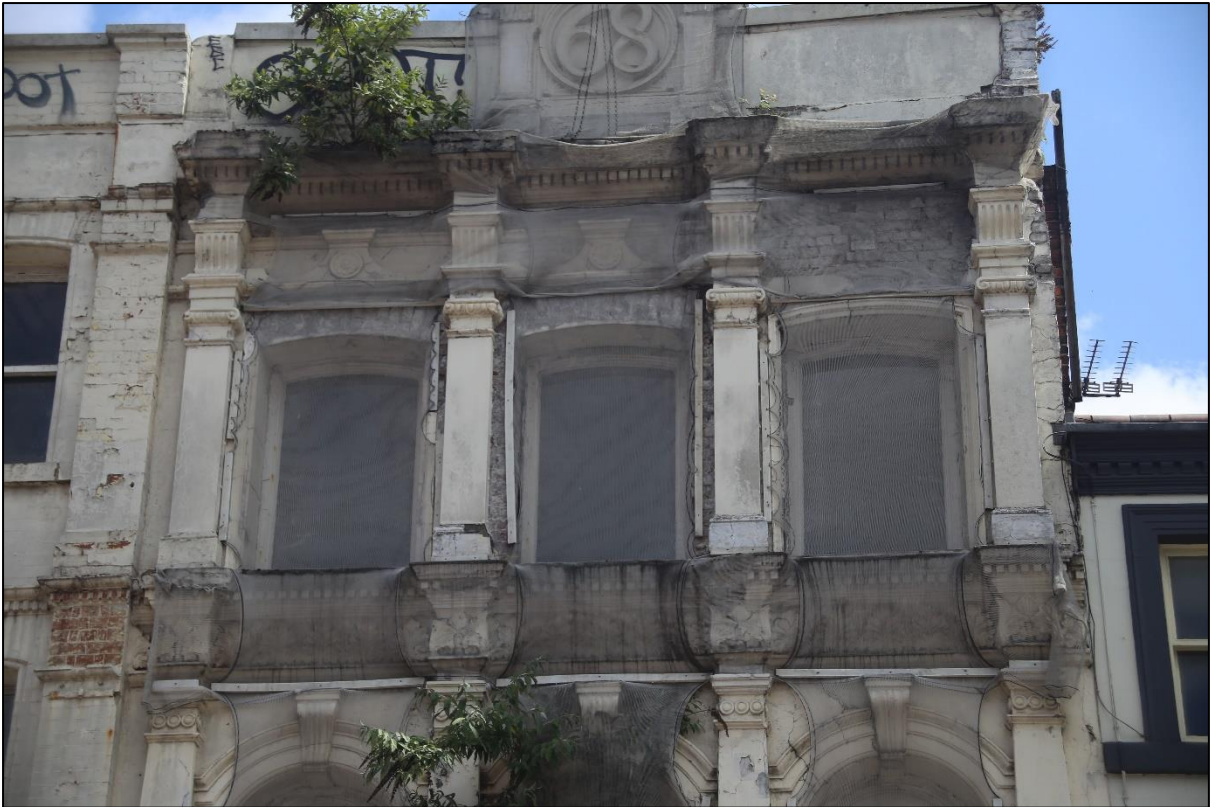
Figure 13: Detail of the second floor windows to No.68, looking south-east
