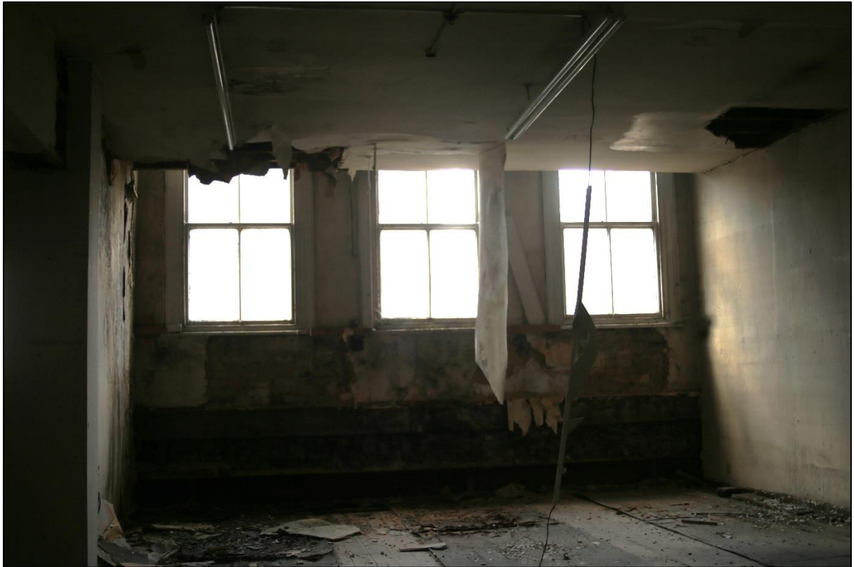
Figure 23: The windows on the first floor of No.70, facing north-west
