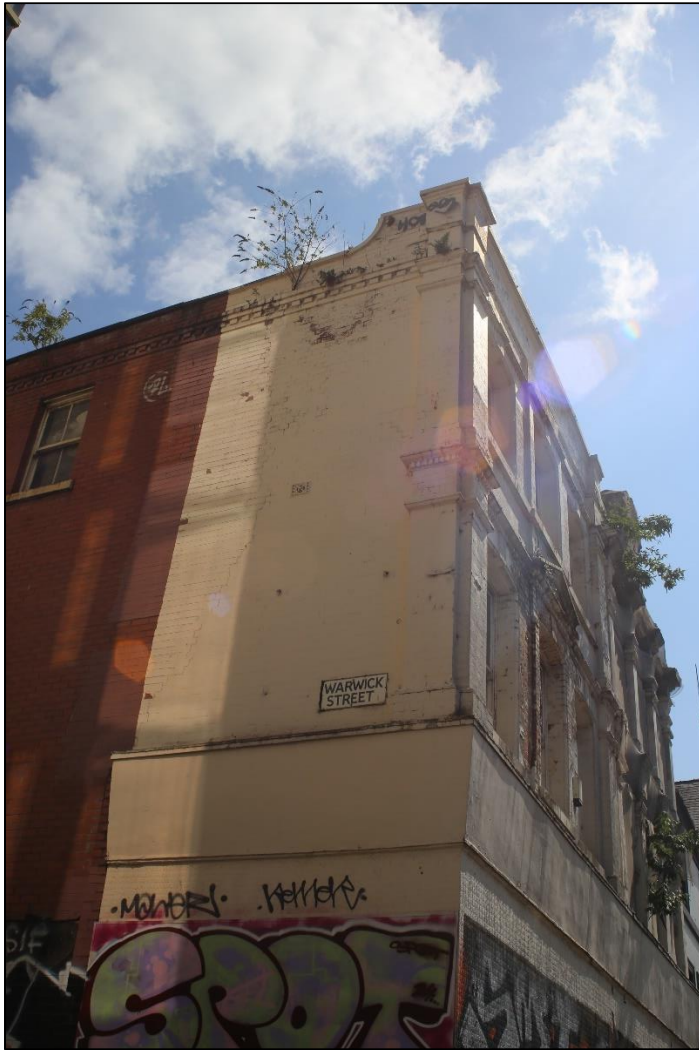
Figure 18: Detail of the upper floors to the north-east façade of No.70, facing south-west
