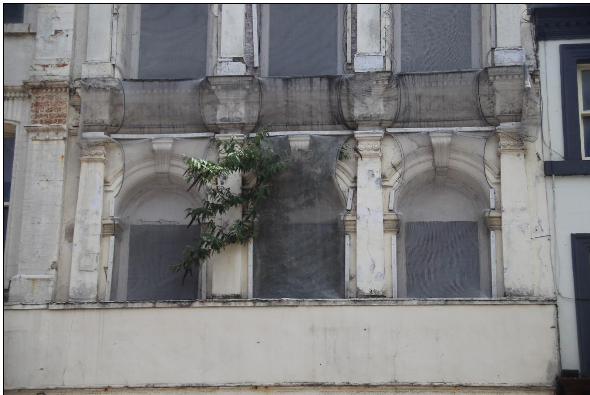
Figure 12: Detail of the first floor windows to No.68, looking south-east
