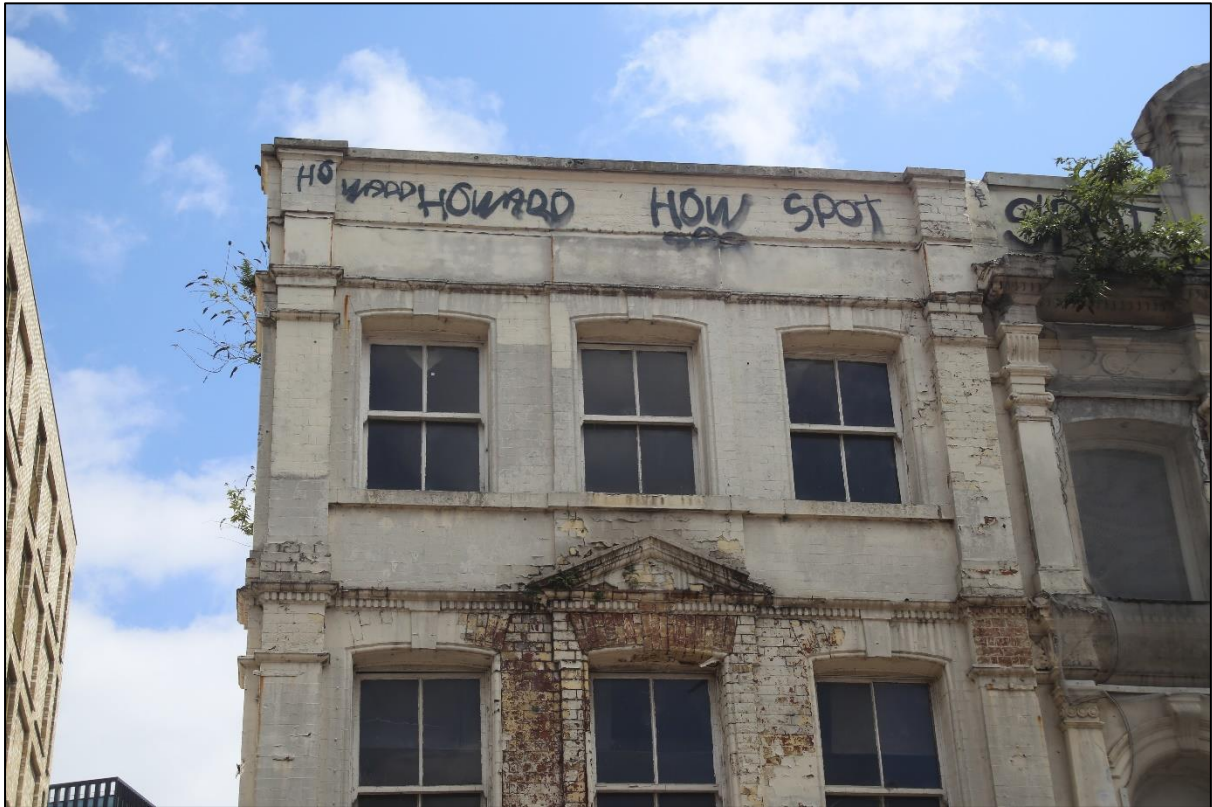
Figure 16: Detail of the second floor of the north-west façade of No.70, facing south-east
