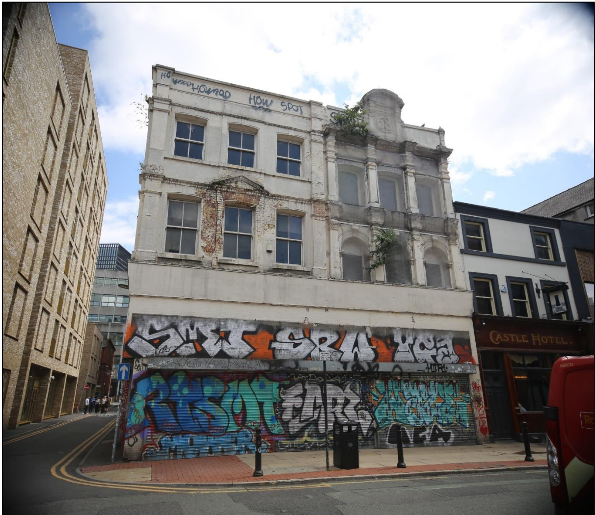
Figure 11: General view of the north-west façade of No.68 and No.70, facing south-east
