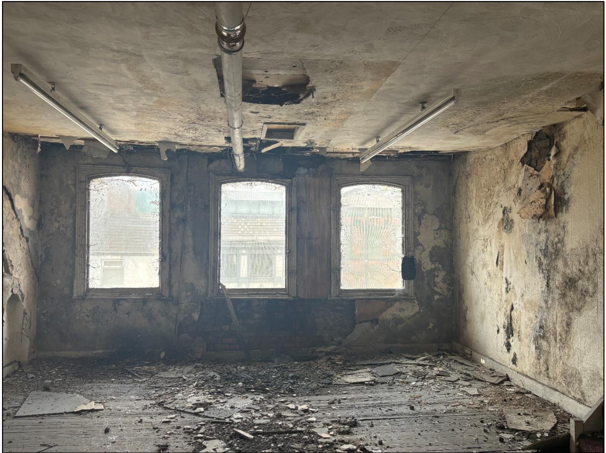
Figure 26: The windows on the first floor of No.70, facing north
