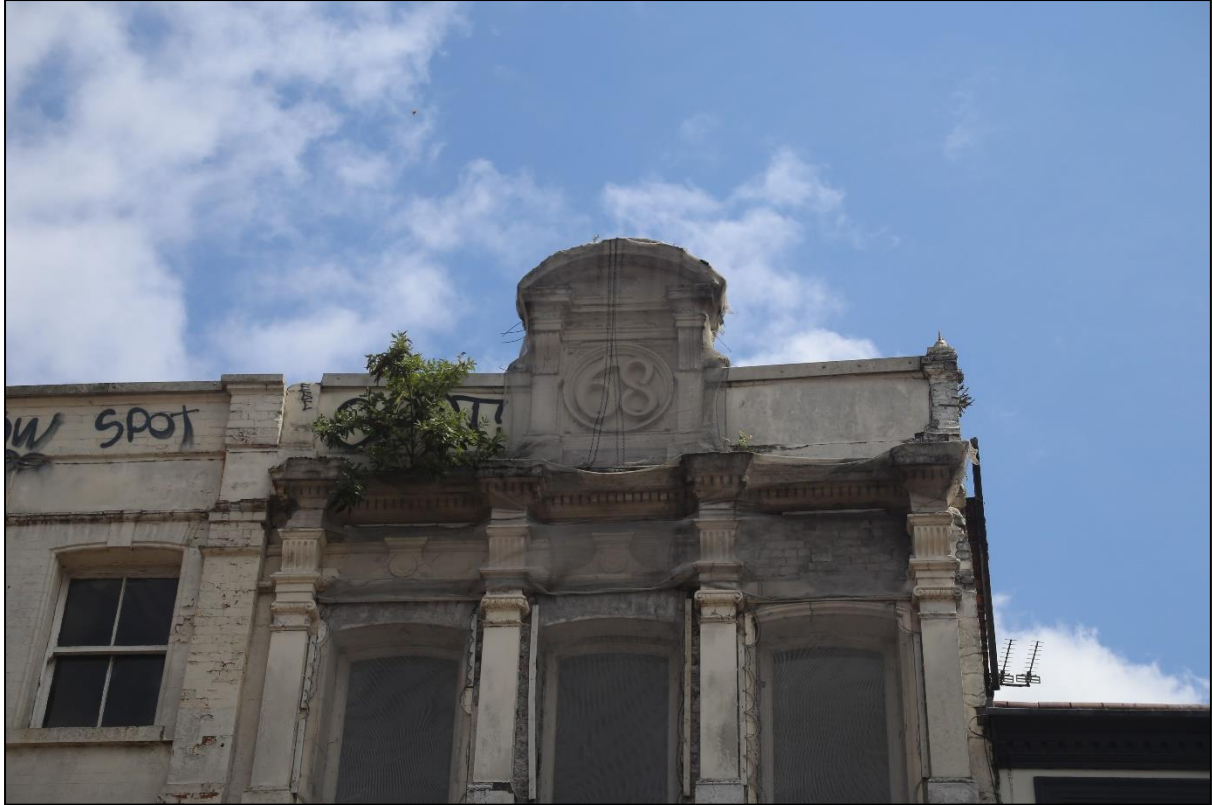
Figure 14: Detail of the pediment of No.68, facing south-east
