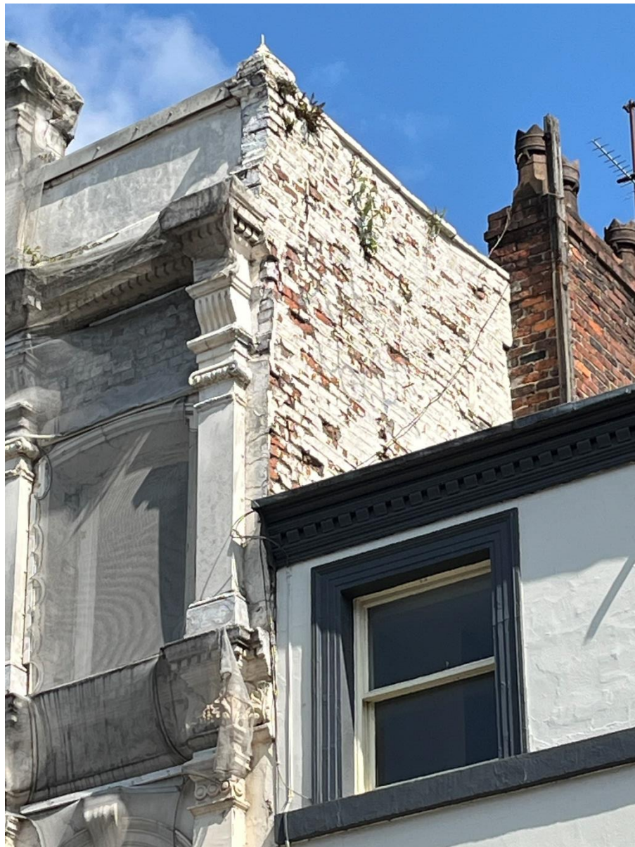
Figure 27: Facade of party wall between No.68 and Castle Hotel
