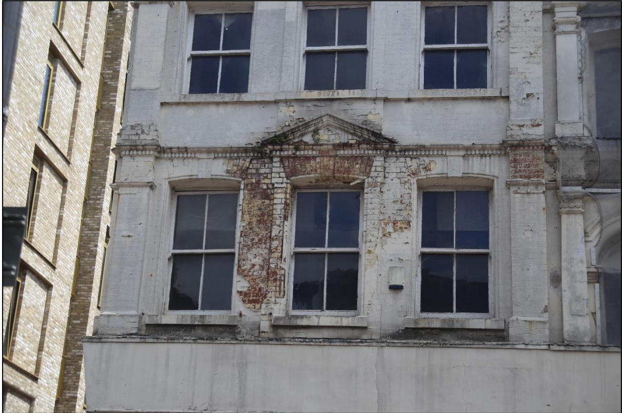
Figure 15: Detail of the first floor of the north-west façade of No.70, facing south-east
