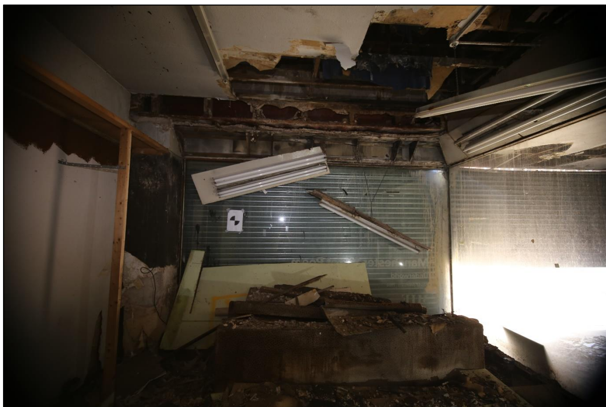
Figure 20: General the mid-20th-century shopfront to the ground floor of No.68, facing north-west
