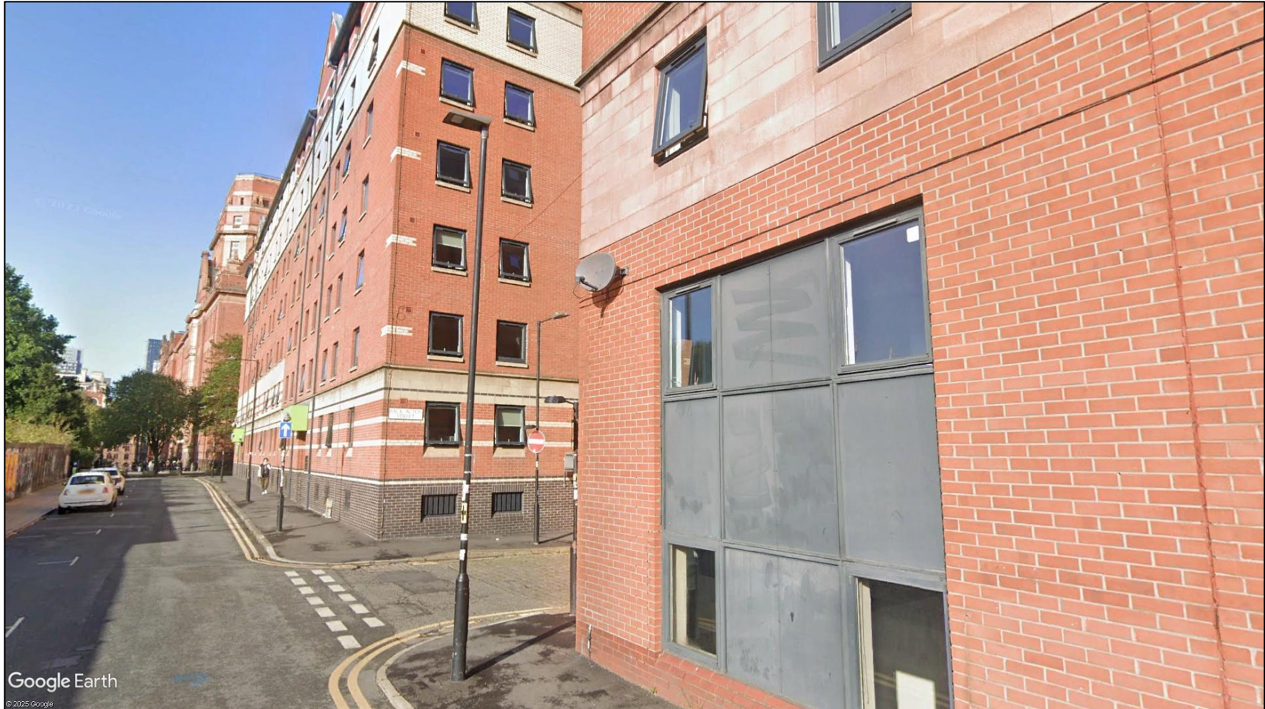
Figure 13 Streetview imagery of observed satellite dish upon Building 12
