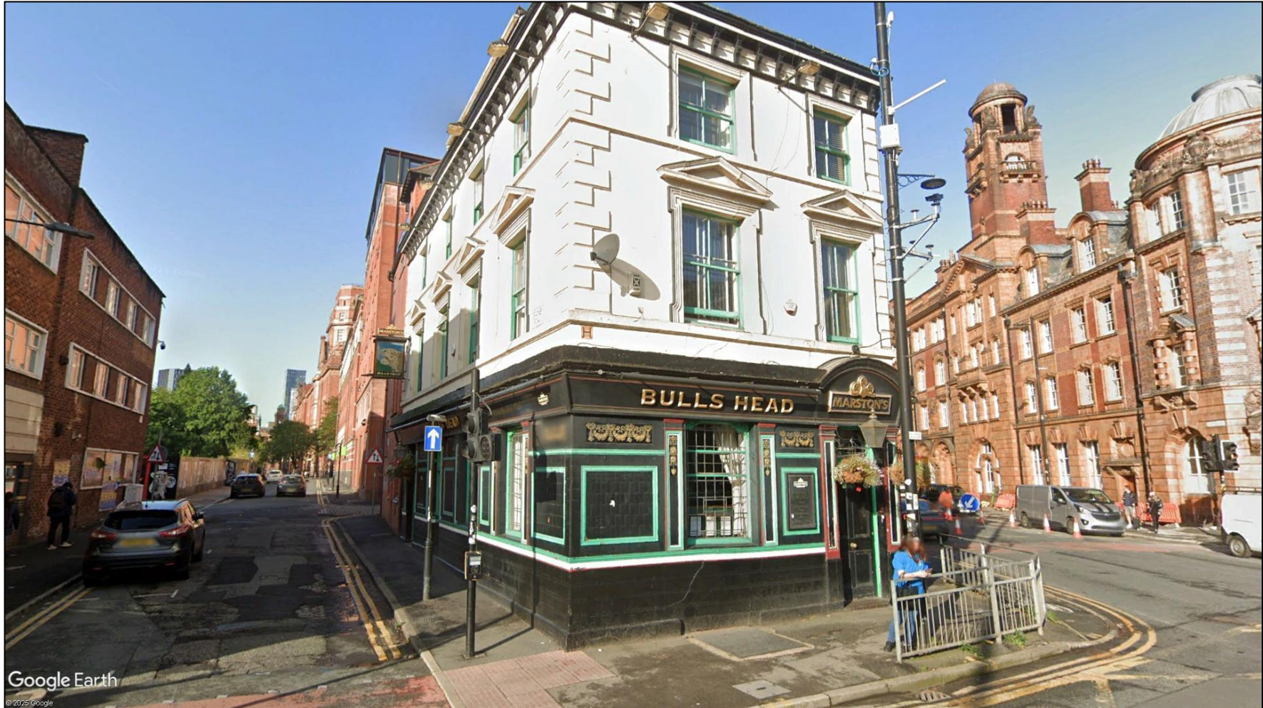
Figure 14 Streetview imagery of observed satellite dish upon Building 13
