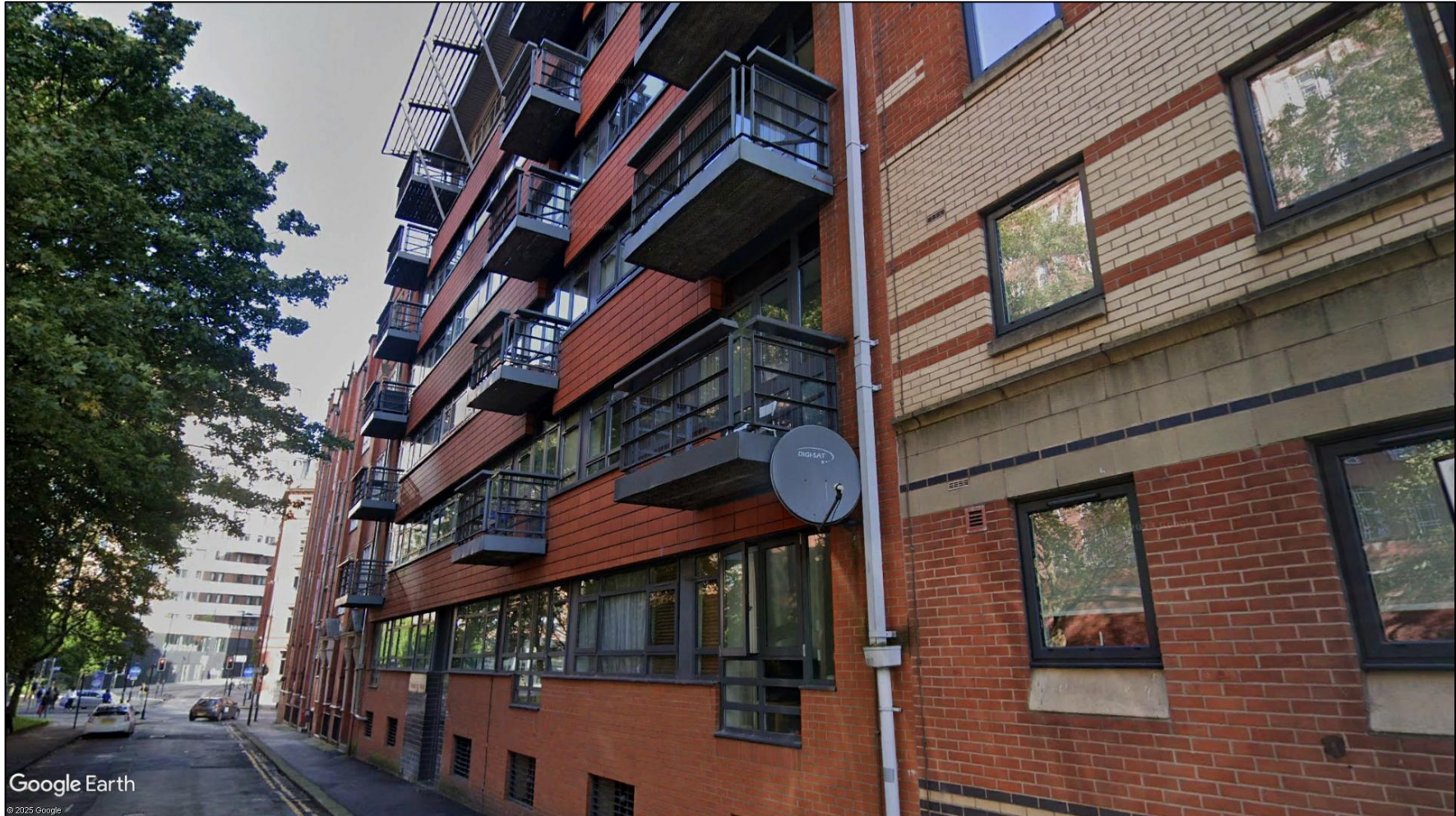
Figure 11 Streetview imagery of observed satellite dish upon Building 9
