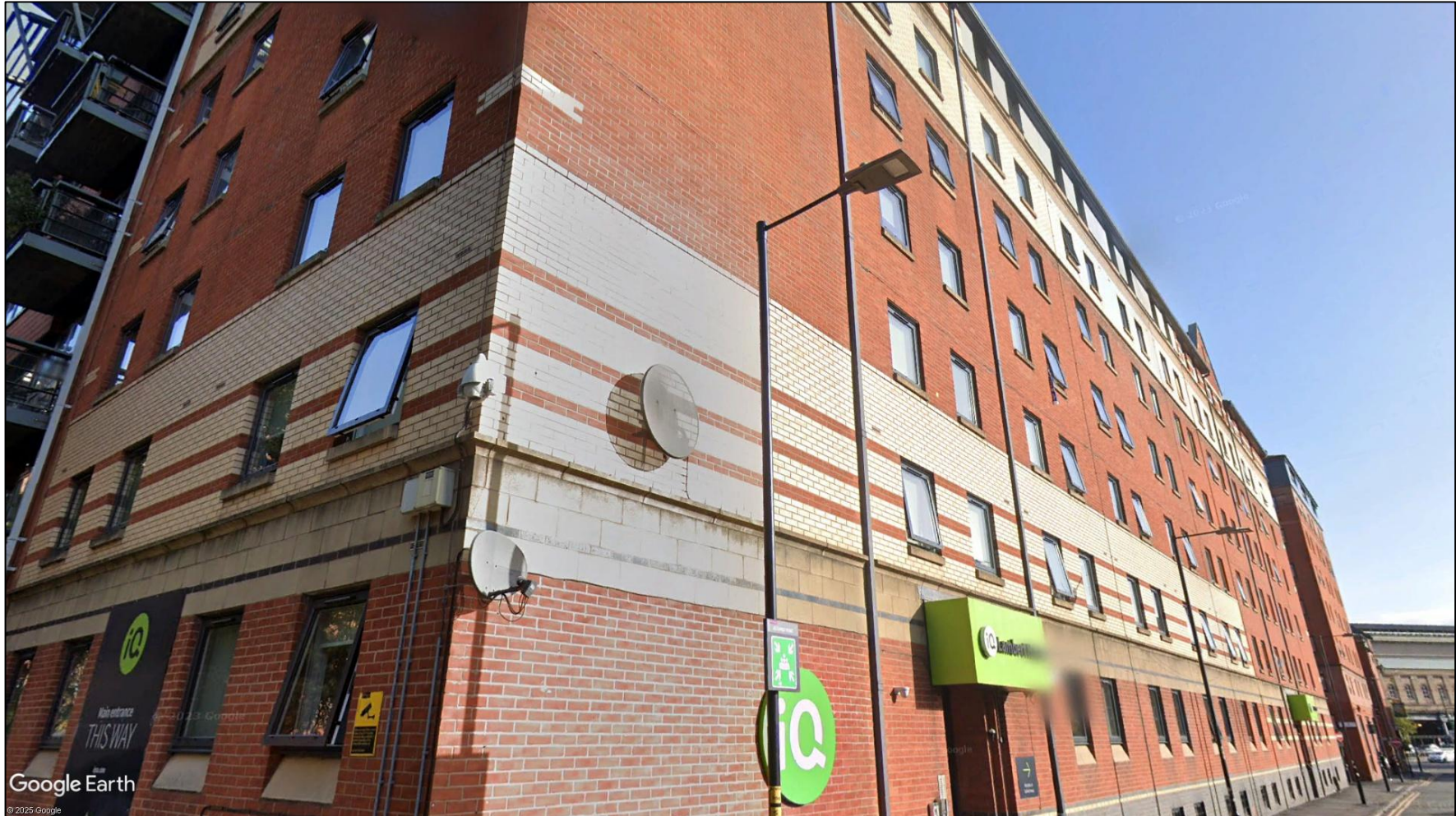
Figure 12 Streetview imagery of observed satellite dishes upon Building 11
