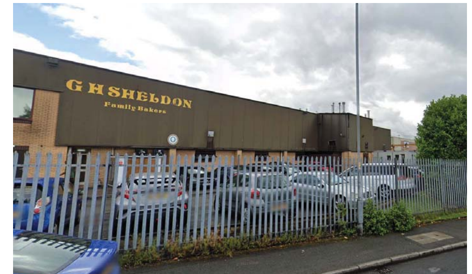
Car parking and service areas back onto the pavement
