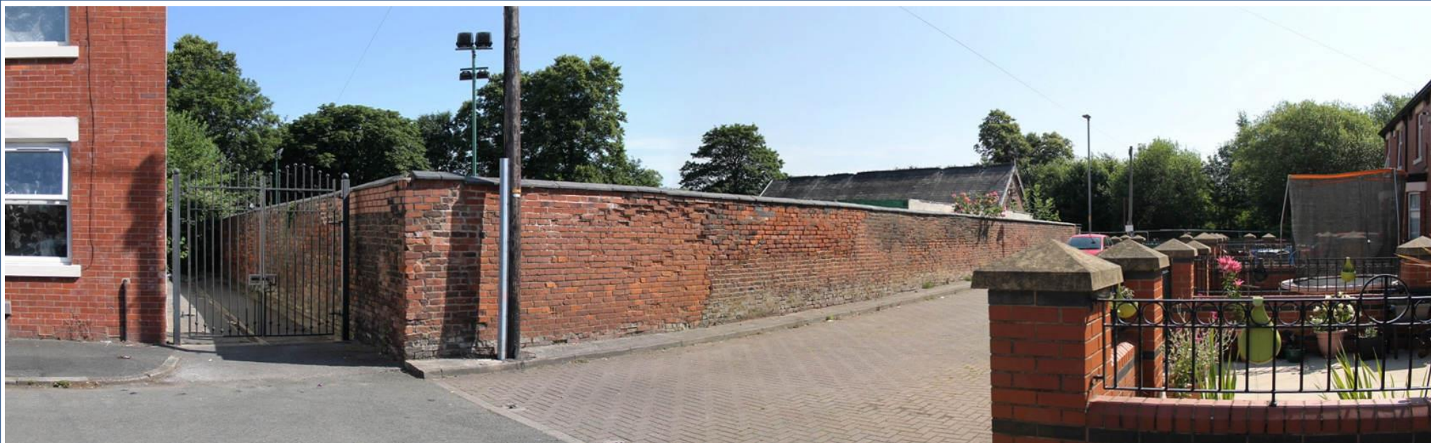
Photo 3, July 2021: Area 1: Site boundary wall from Backwell Street looking north
