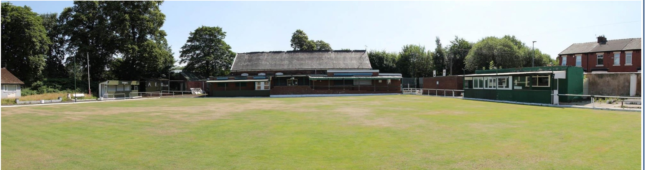
Photo 11, July 2021: Area 1: Looking east across the green towards the main club building
