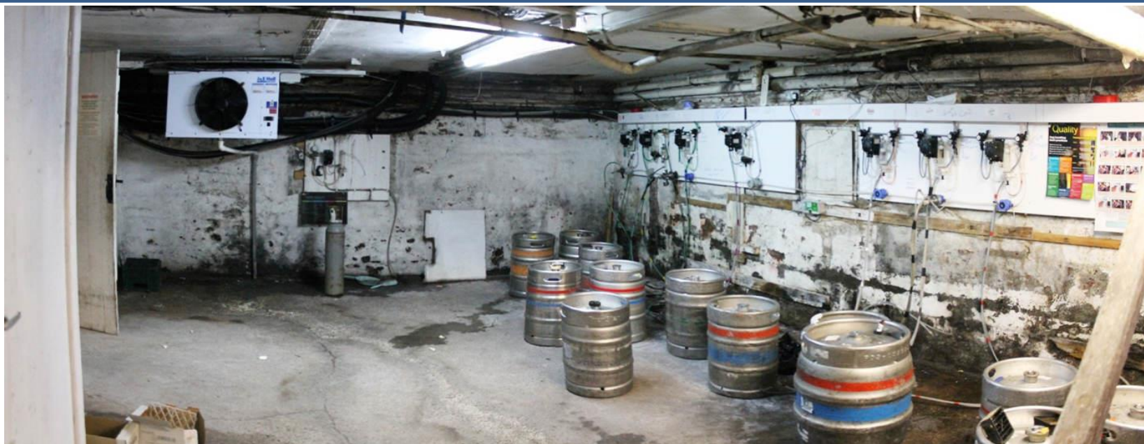
Photo 13, July 2021: Area 1: Main club building basement area 1
