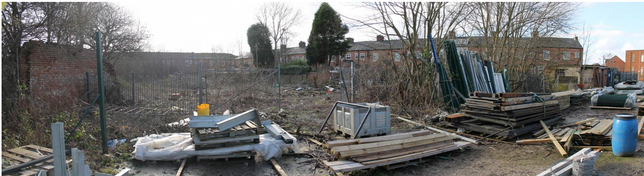
Photo 15, February 2022: Area 2: Access to the west of the site via Burman Street and the Termstall fencing yard
