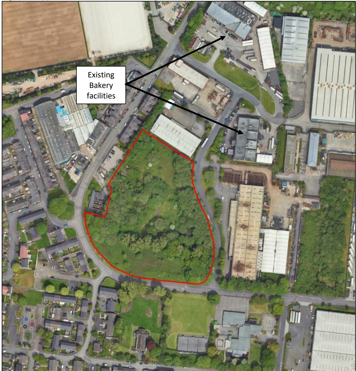
Figure 1: Application site and surroundings
