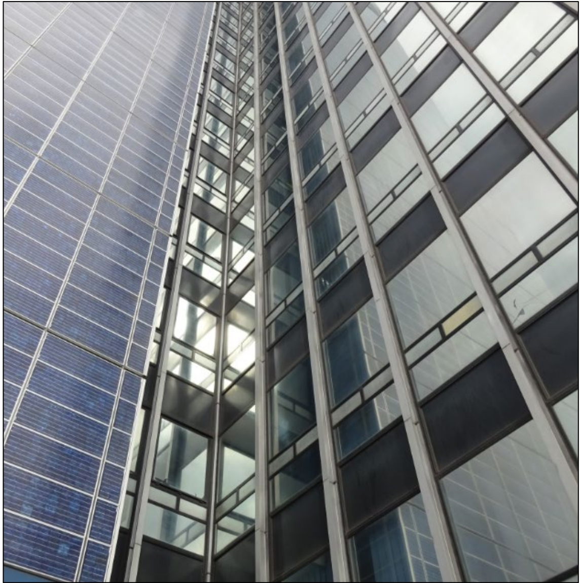
Figure 25. Details of the structural aluminium-alloy (hiduminium) mullions, the internally-fixed glazing panels with the horizontal inset and the black, vitreous-enamelled steel panels fixed externally using sprung-in beads. Note the reflective and opaque character of the glazing.
