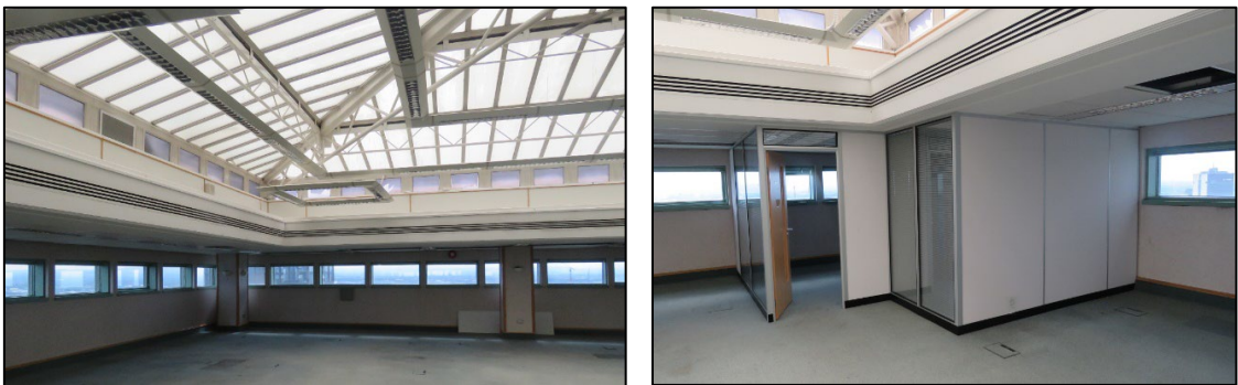
Figure 57. The 25th floor as extant in 2019, following the clearance of the 25th floor, showing the banded observation windows and the inserted corner office partitions.
