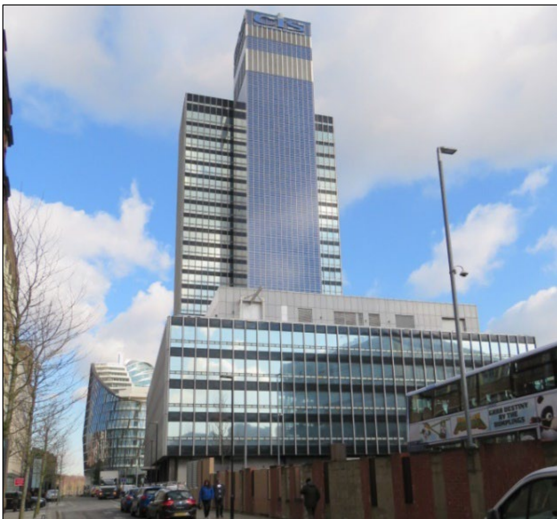
Figure 23. View of the service tower from Dantzic Street (2018), looking north-east towards One Angel Square and illustrating the change in the character of the streetscape. The on-going re-development of the 'listed estate' is expected to further enhance the vitality of the street.
