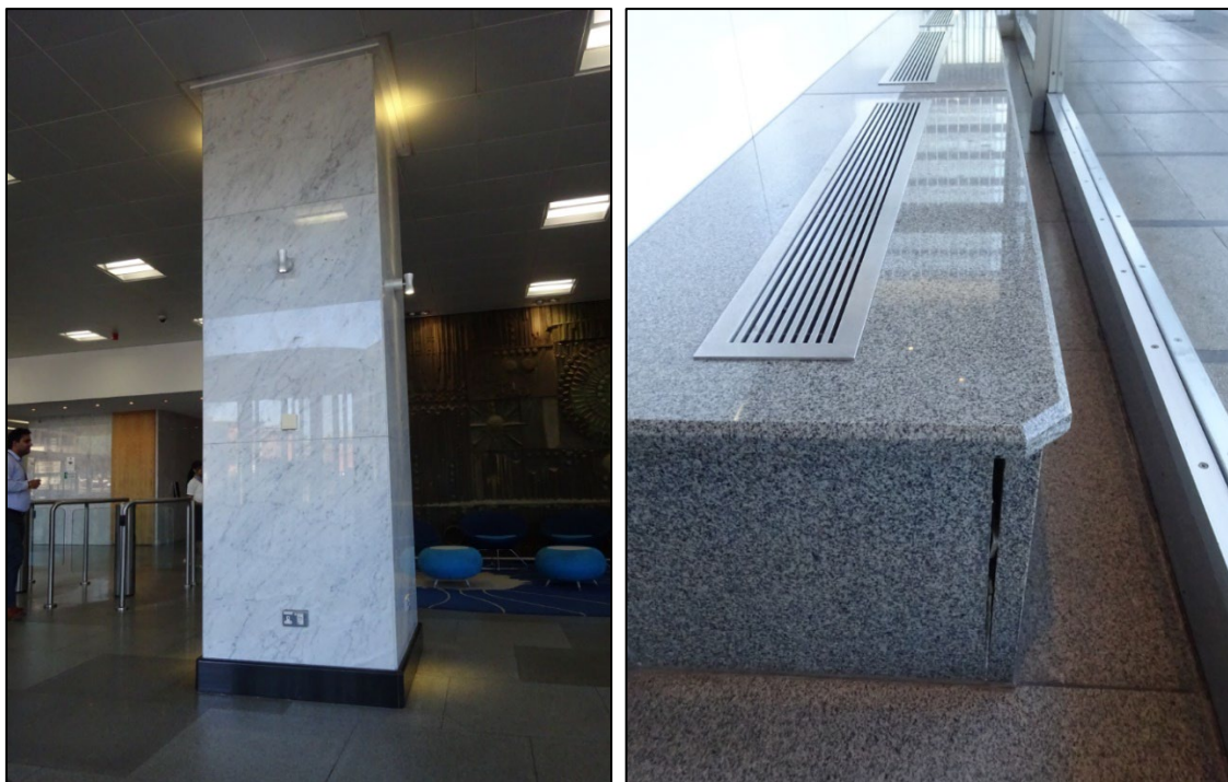
Figure 33. Over-clad columns, encased in the 1980s (originally black, fluted sheet metal cladding) and the cladding to the Weathermaster system in the entrance hall.
