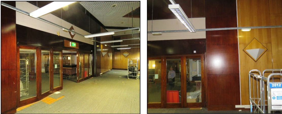
Figure 39. Views (2019, extant as of December 2024) showing the surviving original screen, looking into the bar area (left-hand side) and the additional dark-stained panels and replacement lighting (right-hand view).
