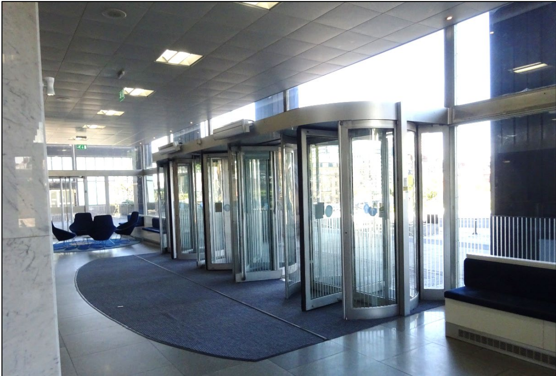
Figure 34. View of the entrance hall (2019, extant as of December 2024) showing the replacement doors and ceiling.
