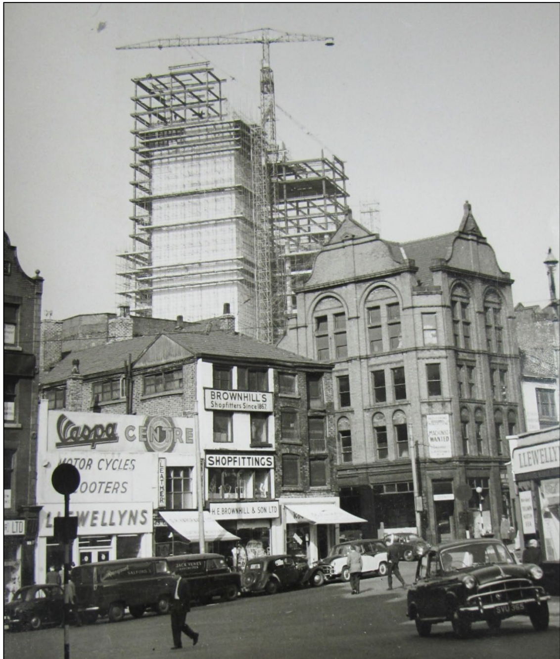
Figure 13: View of the service tower and steel frame of the office floor under-construction from Shudehill. Note that the service tower was enclosed by the rear of commercial and industrial properties and was not intended to be the focus of the architectural expression. Source: Greater Manchester Lives Archive
