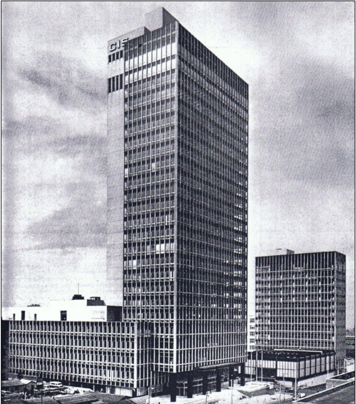
Figure 15: View of the completed building in 1963. Note the transparency of the glazed façade and the deliberate under-statement of the service tower and the podium plant roof.
