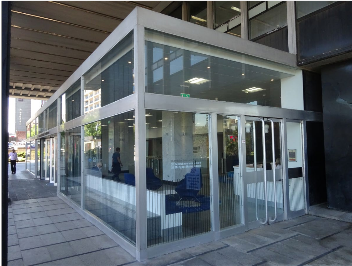
Figure 28. The projecting entrance lobby and access to the reception (2019, extant as of December 2024). All the doors within the projecting box have been replaced. The original arrangement had a single, central revolving door and paired side doors.
