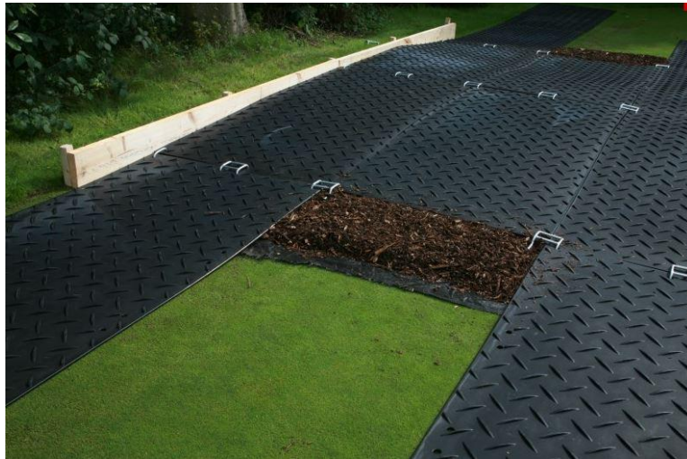
Figure 4. Ground protection interlinked plastic boards with a layer of wood chippings at least 150mm deep.
