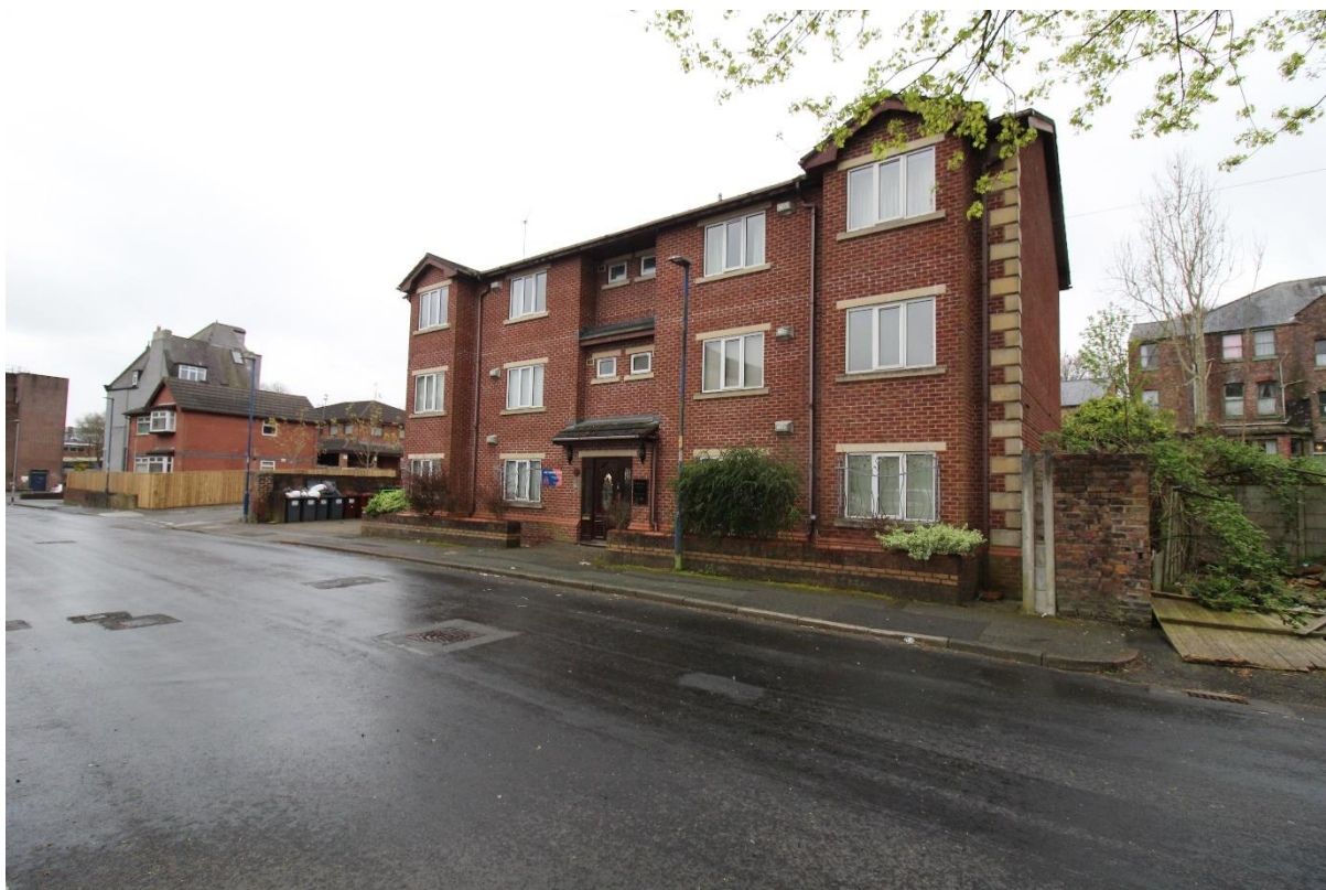
Plate 8 – 1 to 6 Catherine Road to rear of site
