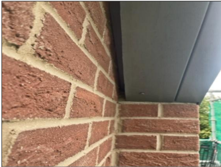
Plate 2: The renewed soffit maintained the roost access for bat via a stand-off from the brickwork.
