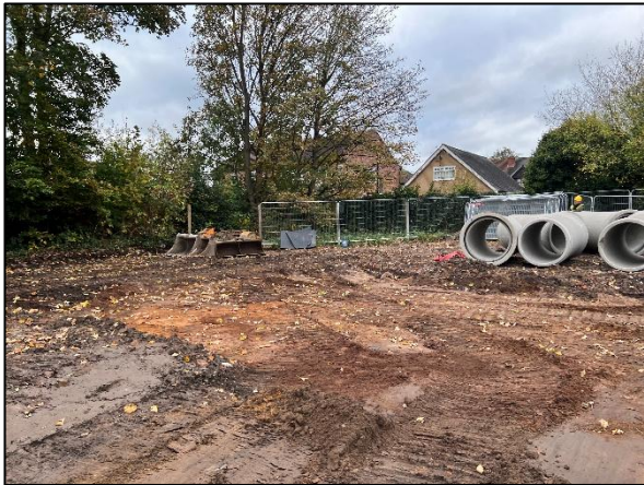
Photographs 9 & 10: Showing the removal of made ground similar to topsoil, exposing the underlying natural strata within Plots 1-4. Photographs taken 24 th October 2024.
