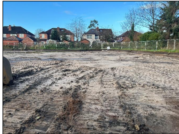
Photograph 12: Shows the removal of made ground similar to topsoil, exposing the underlying natural strata within Plots 15-20. Photograph taken looking from Plot 21 towards the northwestern most corner of site. Photographs taken 25 th November 2024.
