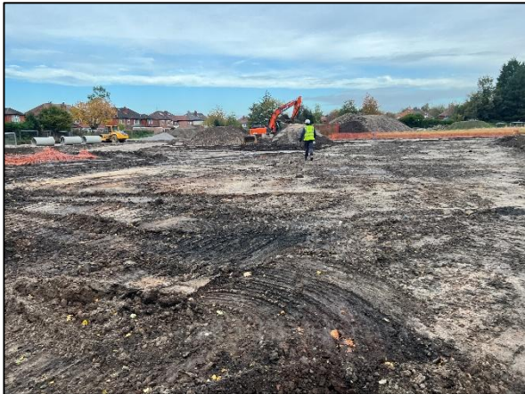
Photograph 7: Shows the removal of made ground similar to topsoil, exposing the underlying natural strata within Plots 41-43. Photograph taken looking from Plot 41 towards Plot 48 to the north. Photographs taken 21 st October 2024.
