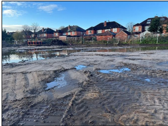
Photograph 11: Shows the removal of made ground similar to topsoil, exposing the underlying natural strata within Plots 10-14 & frontages of Plots 54-57. Photograph taken looking from Plot 17/18 towards Plots 10-14 to the southwest. Photographs taken 25 th November 2024.
