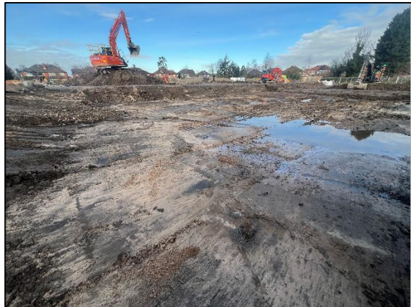
Photograph 18: Shows the removal of made ground similar to topsoil, exposing the underlying natural strata within Plots 29-31. Photograph taken looking from the rear garden of Plot 31 towards Plot 29. Photograph taken 14 th March 2025.
