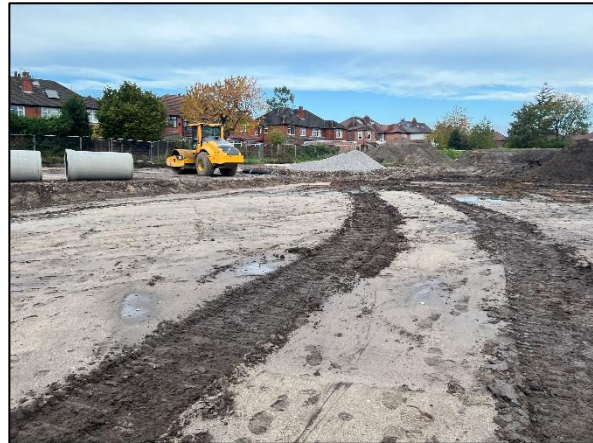
Photograph 8: Shows the removal of made ground similar to topsoil, exposing the underlying natural strata within Plot 58 & 57 driveway. Photograph taken looking from Plot 49 towards the northwest of site. Photographs taken 21 st October 2024.
