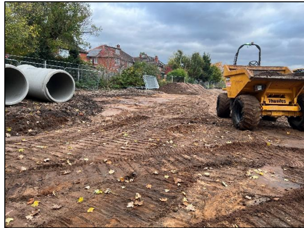
Photographs 9 & 10: Showing the removal of made ground similar to topsoil, exposing the underlying natural strata within Plots 1-4. Photographs taken 24 th October 2024.
