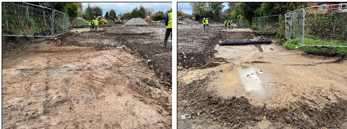
Photographs 1 & 2: Showing the removal of made ground similar to topsoil, exposing the underlying natural strata within the gardens of Plots 5-9. During this visit the pile mats had been placed on plots following the removal of the topsoil. Photographs dated 9 th October 2024.
