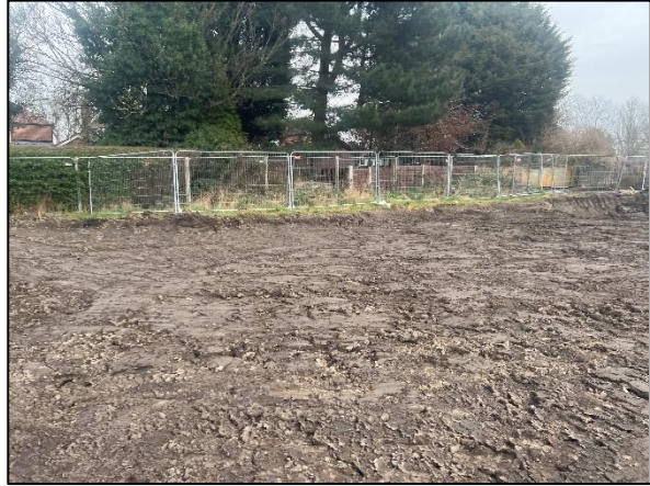
Photographs 15 & 16: Showing the removal of made ground similar to topsoil, exposing the underlying natural strata within Plots 25-28. Photograph taken looking from Plot 28 towards the northern site boundary following removal of the stockpile that was in place across these areas during the previous visit. Photographs taken 19 th February 2025.
