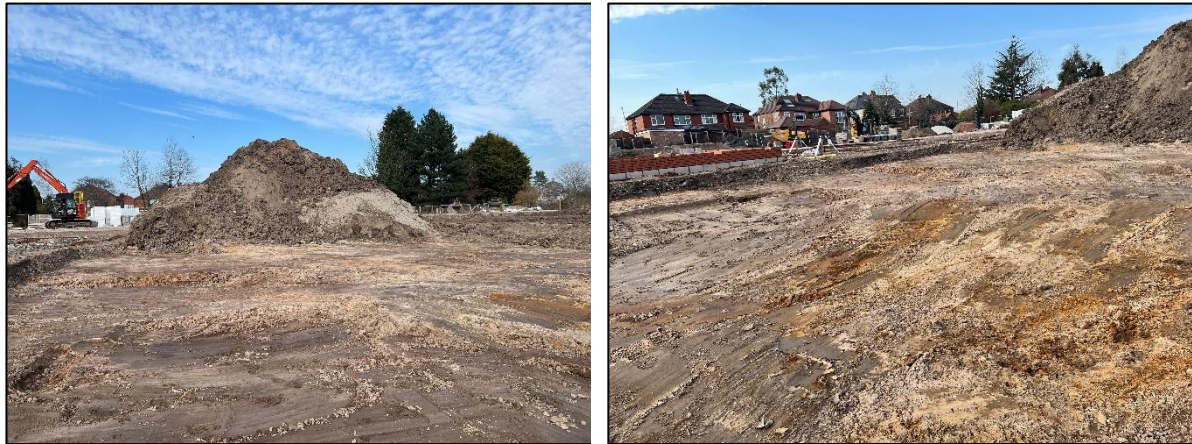
Photographs 19 & 20: Showing the removal of made ground similar to topsoil, exposing the underlying natural strata within the rears of Plots 50-51 & 56-57. Due to limited space across site, the material removed was stockpiled over the location of Plots 52-55, to be validated once the stockpile has been removed. Photographs taken 19 th March 2025.
