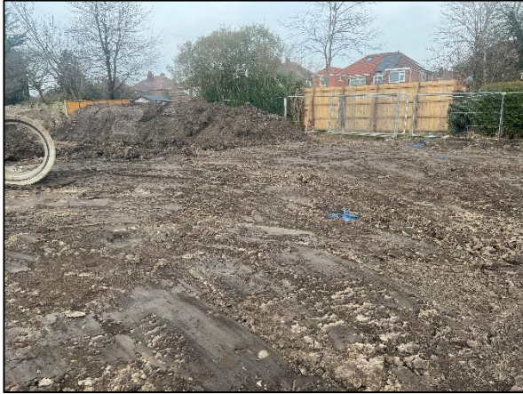
Photographs 15 & 16: Showing the removal of made ground similar to topsoil, exposing the underlying natural strata within Plots 25-28. Photograph taken looking from Plot 28 towards the northern site boundary following removal of the stockpile that was in place across these areas during the previous visit. Photographs taken 19 th February 2025.
