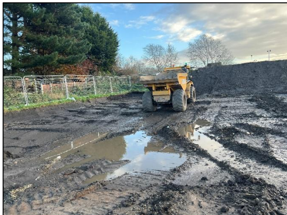
Photograph 13: Shows the removal of made ground similar to topsoil, exposing the underlying natural strata within Plots 21-24. Photograph taken looking from Plot 20 towards to the northeastern most corner of site. A stockpile was located within the location of Plots 25-28 at the time of the visit (shown in the background). Photographs taken 25 th November 2024.
