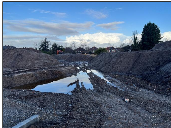
Photograph 14: Shows the removal of made ground similar to topsoil, exposing the underlying natural strata within Plots the frontages of Plots 49-54. The photograph is shown looking towards stockpiles located within the rear gardens of Plots 50-57. The photograph shown is obscured by water due to the site being waterlogged at the time of the visit, however Coopers validated the natural strata visible in these areas during the visit. Photographs taken 25 th November 2024.
