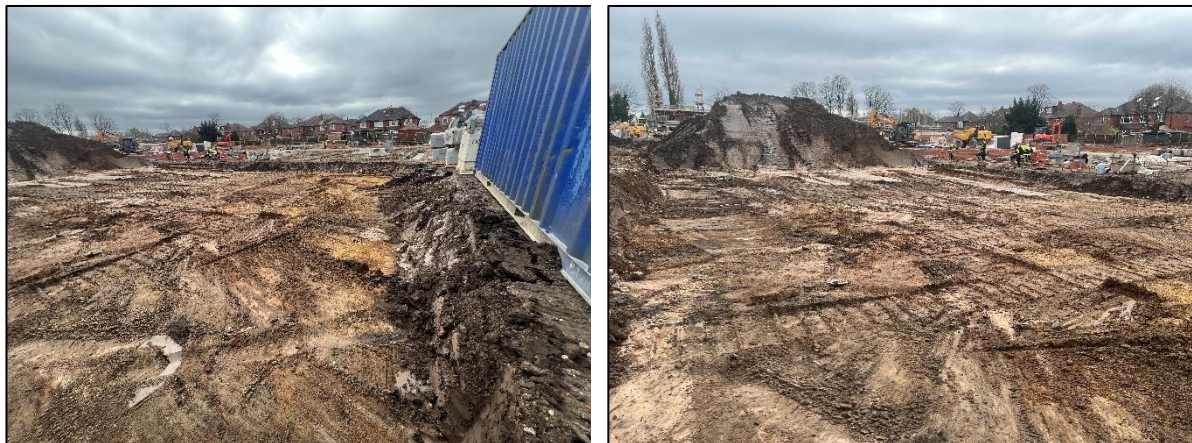
Photographs 21 & 22: Showing the removal of made ground similar to topsoil, exposing the underlying natural strata within the rears of Plots 52-55. Photographs taken looking towards the southwest/south of site. Photographs taken 25 th March 2025.
