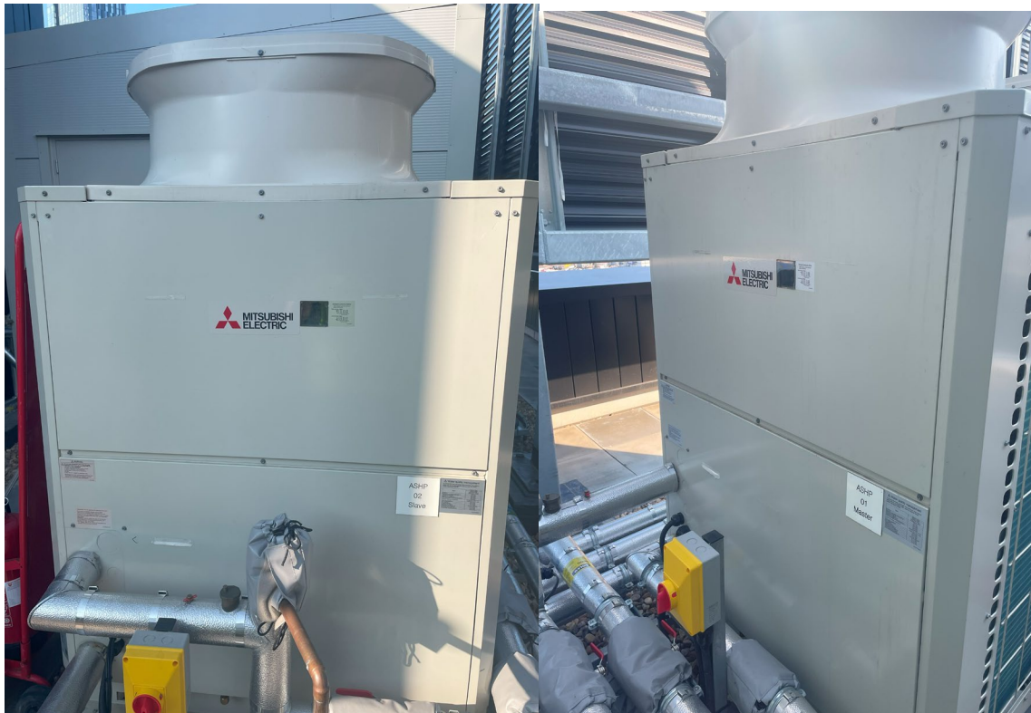
The site visit confirms the installation of ASHP
